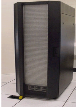
Figure 1.6: IBM's Rear door heat exchanger [10]
