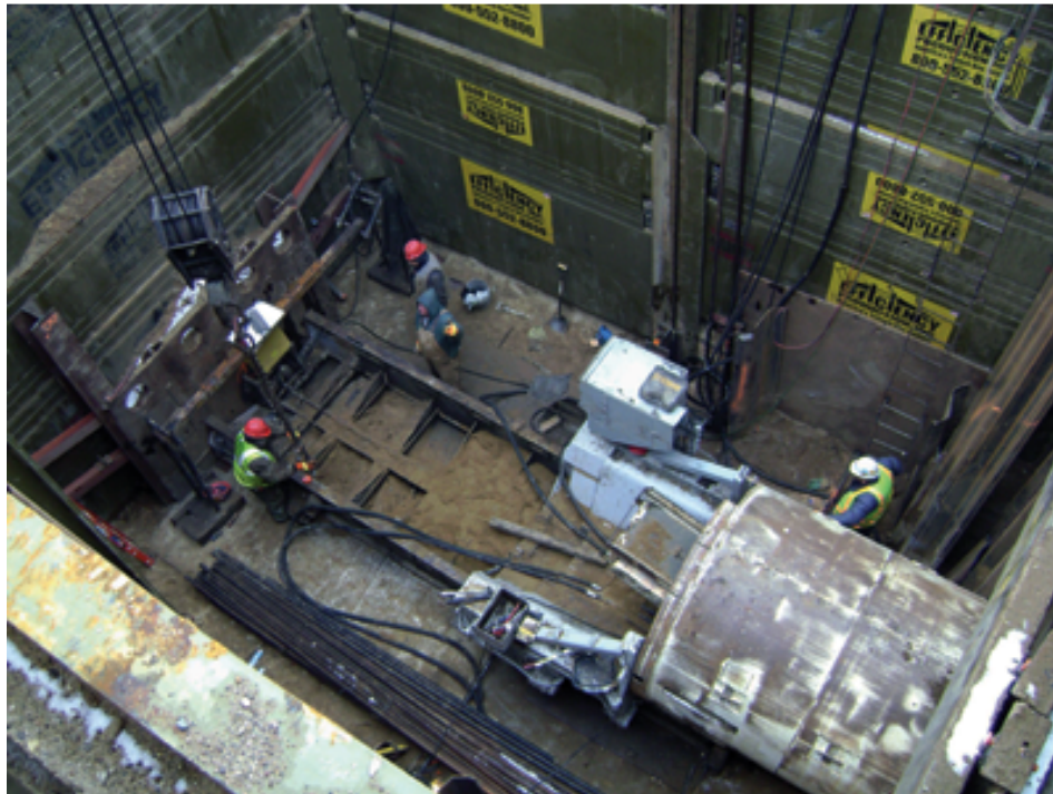
Figure 2.14: Slide Railing System (Shoring Solutions, 2012)
