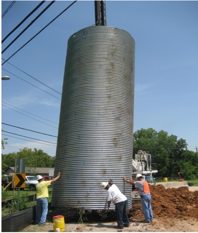
Figure 2.17: Corrugated Metal Pipe Shaft (Reed, 2012)
