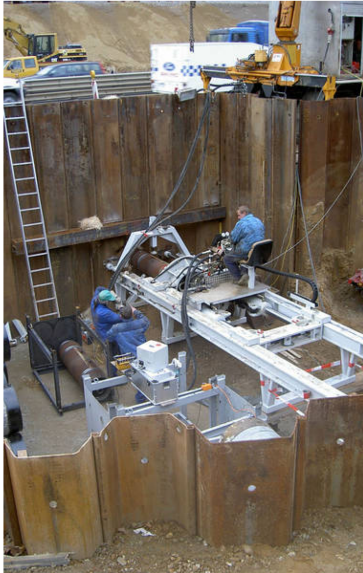
Figure 2.15: Steel Sheet Piles (Midwest Mole Inc., 2012)
