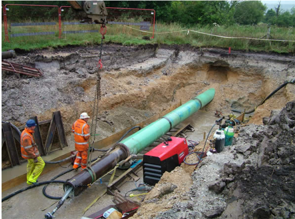
Figure 2.5: Pipe Ramming (Allen Watson Ltd, 2012)
