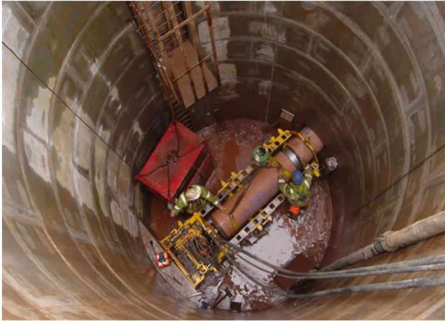
Figure 2.18: Circular Concrete Shaft (Allen Watson Ltd, 2012)
