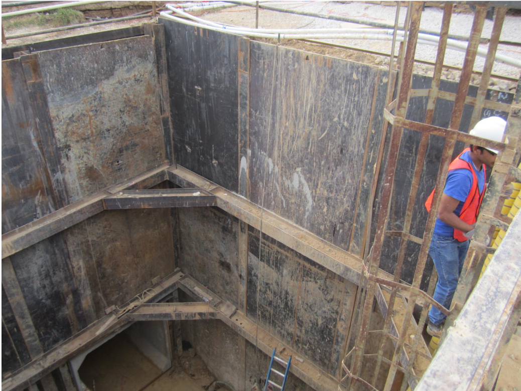
Figure 2.16: Soldier Piles with Steel Lagging
