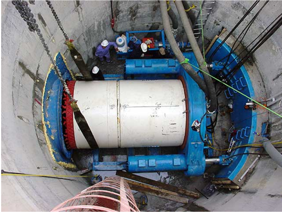
Figure 2.3: Microtunneling Machine (Allen Watson Ltd, 2012)
