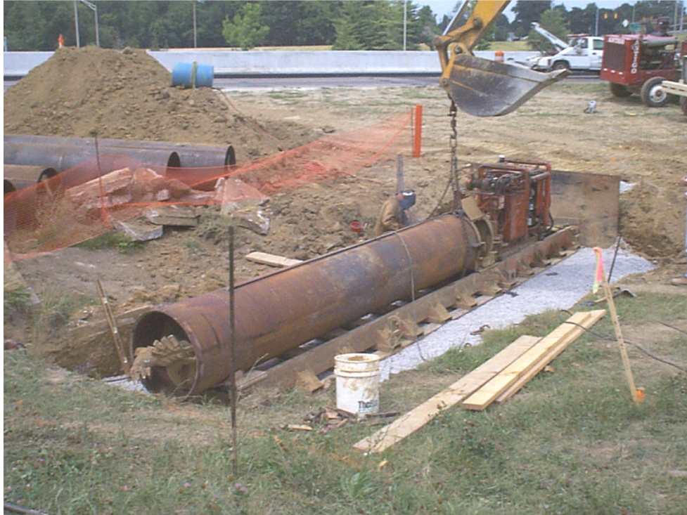
Figure 2.2: Horizontal Auger Boring Machine (Abraham, et al, 2002)
