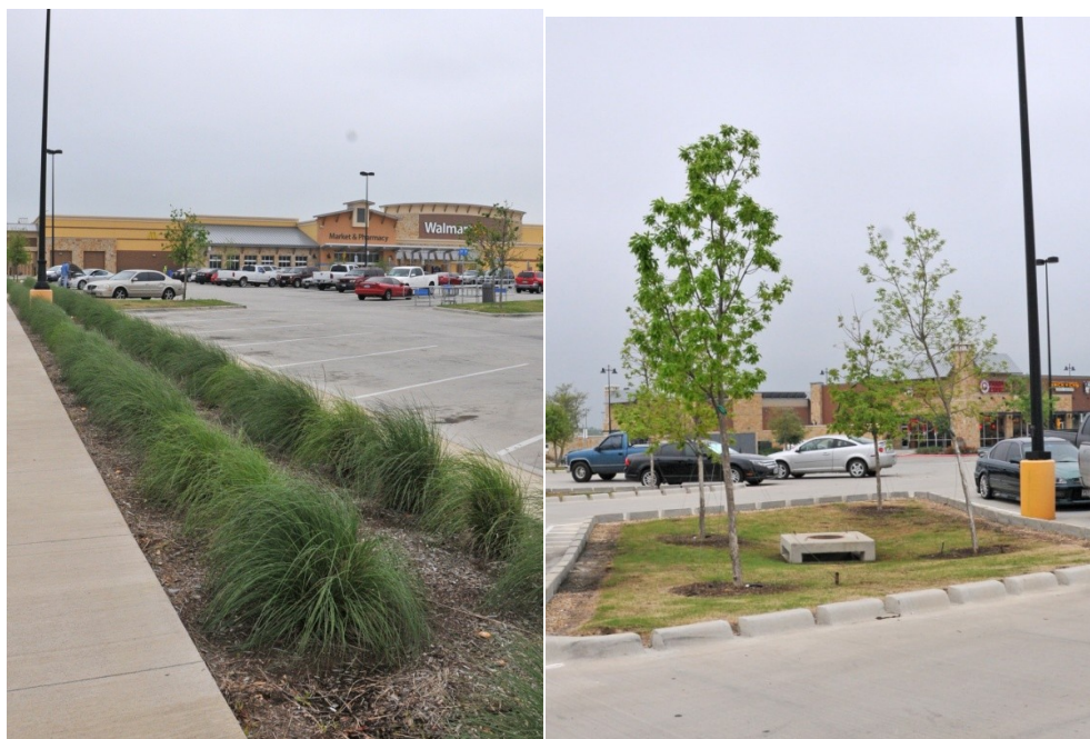
Figure 4.10 LID practices constructed at Rayzor Ranch
