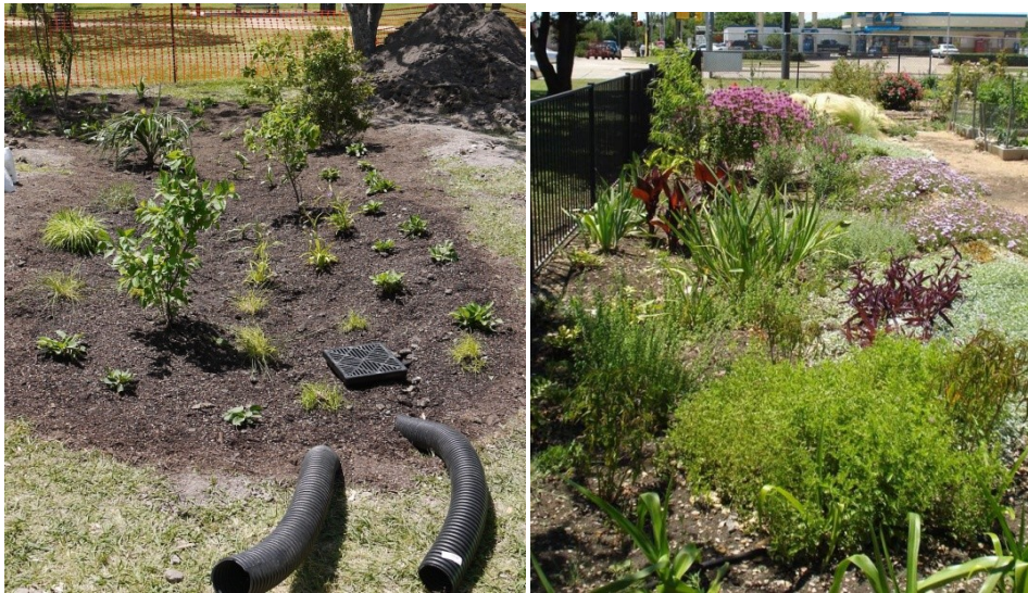
Figure 2.12 Rain Garden and Bioretention Area (Source: Dr. Fouad Jaber, Texas Agrilife Research and Extension Center, 2012)
