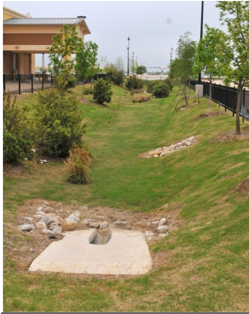
Figure 4.11 LID practices constructed at Rayzor Ranch
