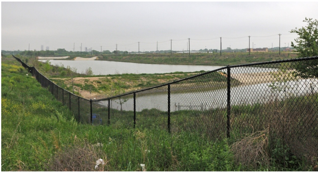
Figure 4.12 LID practices constructed at Rayzor Ranch
