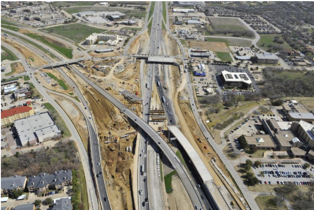
Figure 3.2 SH 121/183 Split Facing East (NTE 2010)
