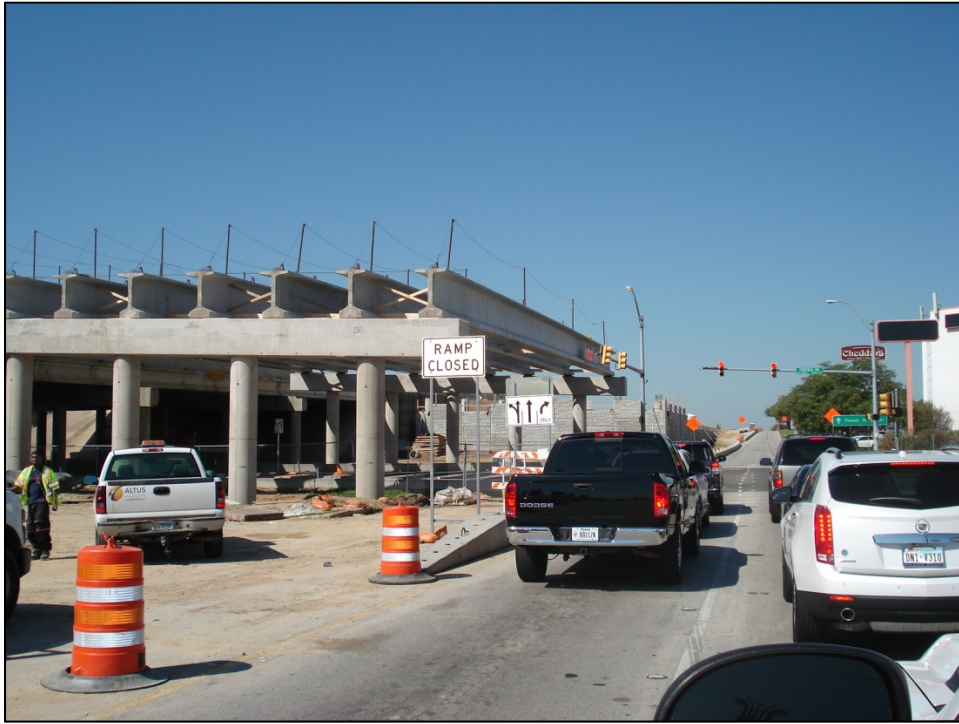
Construction on South Side of SH 121 at Central Dr.
