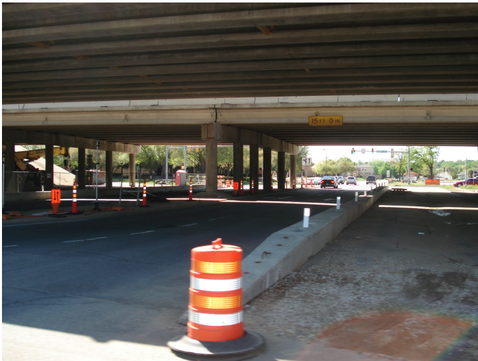
Construction Underneath SH 121 at Forest Ridge
