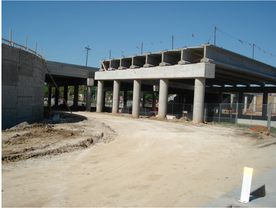
Construction on the South Side of SH 121 at Bedford Road
