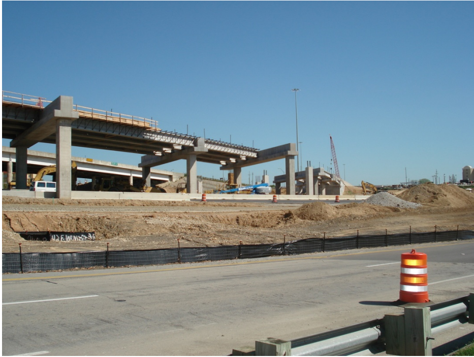
Construction of the SH 121 Northbound Connector
