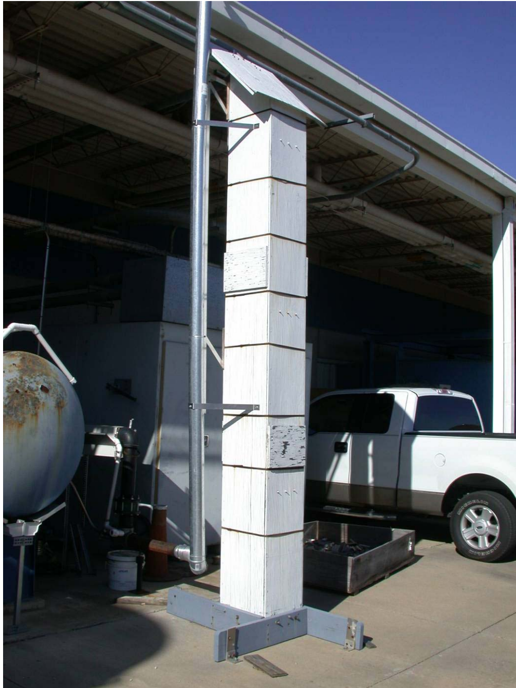
Figure 2.16 Ejector Pump Silencer
