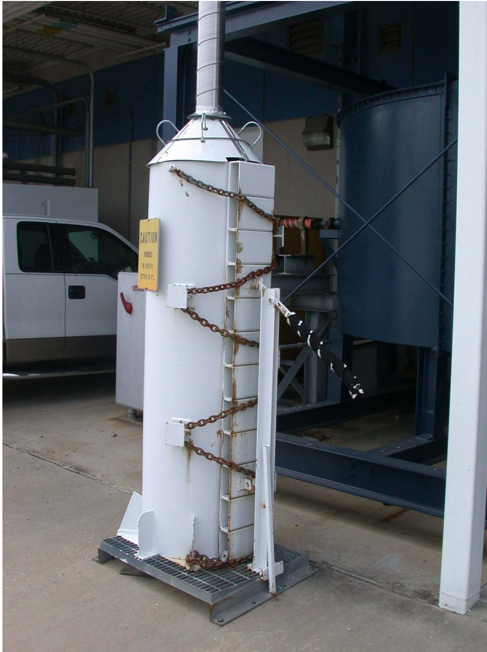
Figure 2.27 Fuel Storage Building
