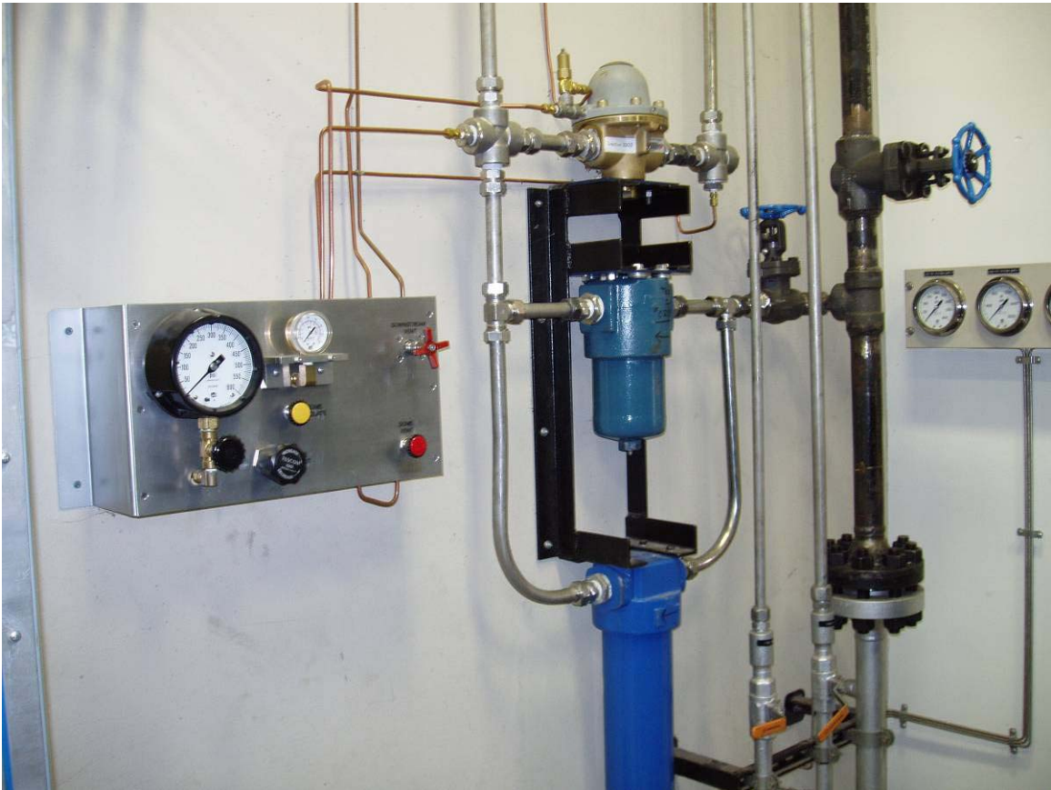
Figure 2.11 Air Injection System for Ejector Pump
