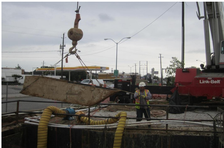
Figure.3.7: Bucket Filled with Soil Lifted to be Unloaded at Ground Surface
