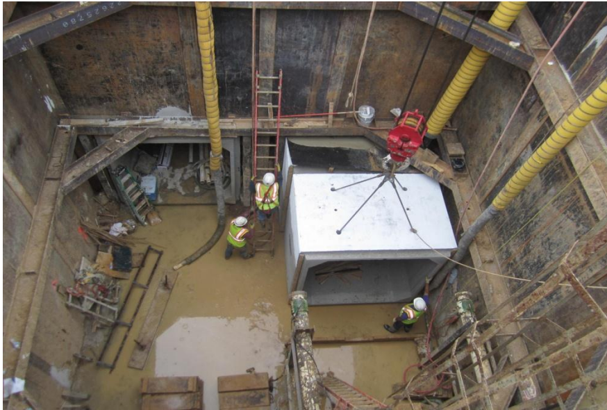
Figure.3.5: Placing Box Segment on the Guide Rails
