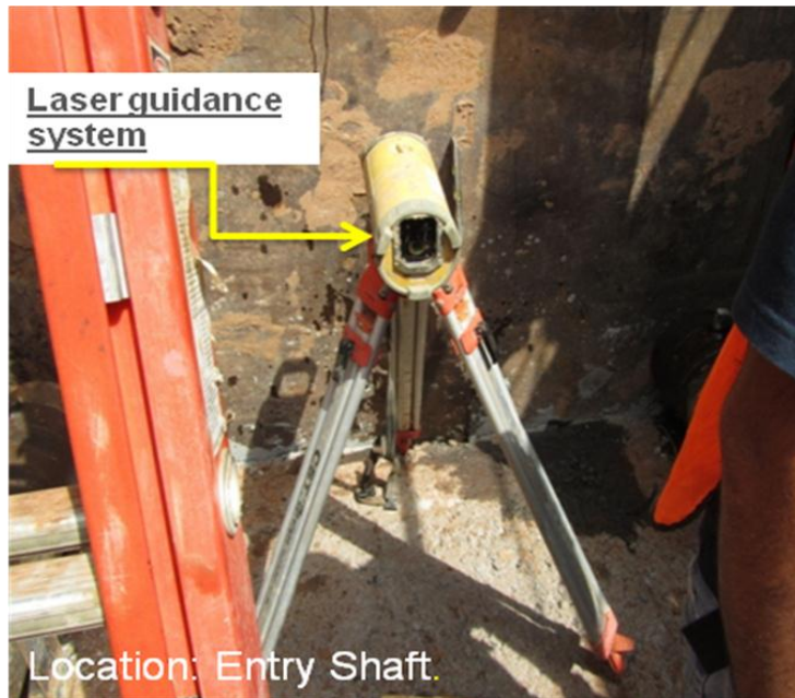
Figure.3.15: Close-Up View of Laser Guidance System
