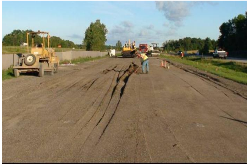
Figure 4.6 Rutting Caused in Cell 77 and 78
