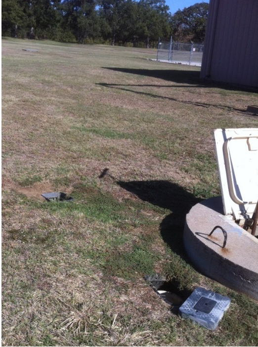
Yard Piping showing venturi tap locations
