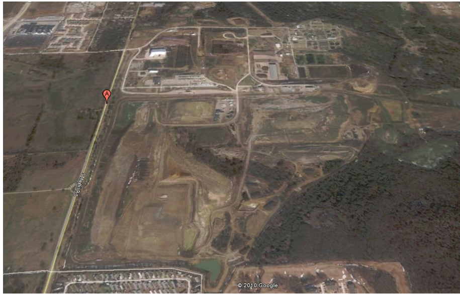
Figure 3.1 City of Denton Landfill (Aerial View)
