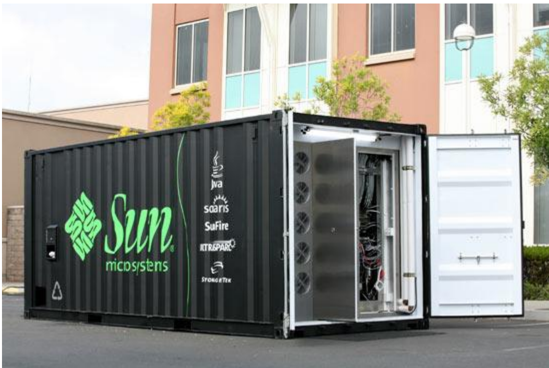
Figure 1.1: Sun Microsystems Modular Data Center [5]
