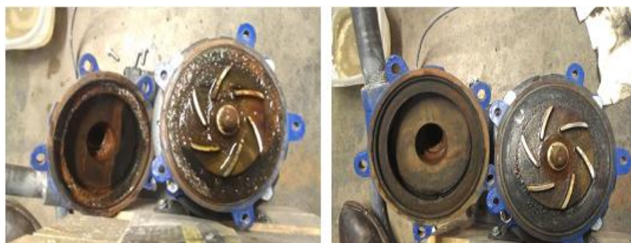
Figure 5.9: Pump Casing before and after cleaning
