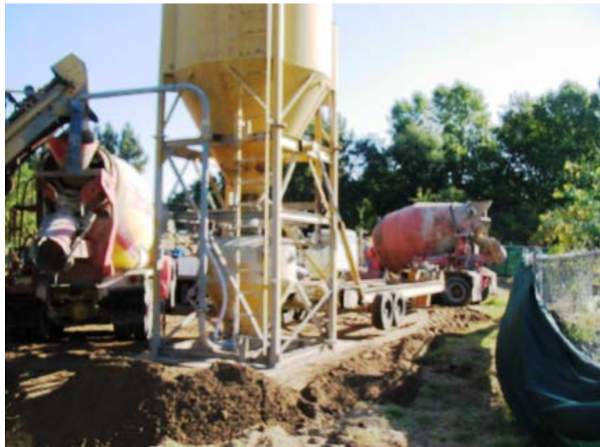
Figure 2.6 Small On–Site Batch Plant for CLSM Mixing (Finney et al.,1998).
