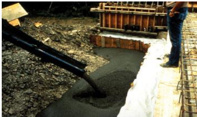
Figure 2.3 Bridge Abutment Backfill with Flowable Fill (Source: FHWA/ Flowable fill)
