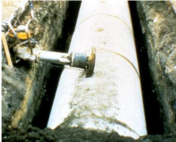
Figure 2.4 CLSM as Bedding Material for Narrow Trench (Source: FHWA/Flowable fill)
