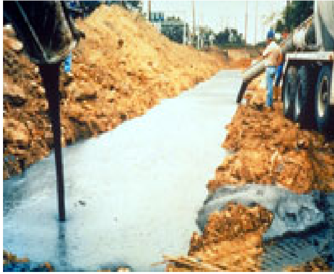
Figure 2.1 Shows the Quick Discharge of CLSM (Source:www.cement.org)
