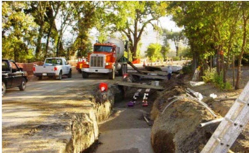
Figure 2.7 CLSM Discharge into trench from Ready -Mix Truck (Finney.,1998)
