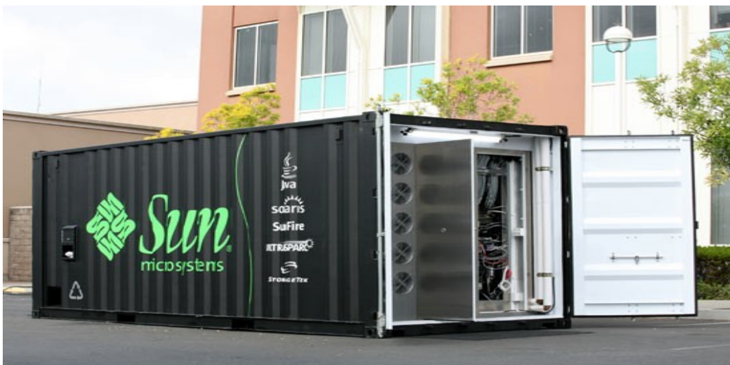
Figure1.1: Sun Microsystems Modular Data Center: Project Black Box [6]
