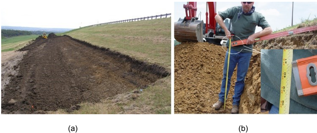
Figure 4.2. Excavation of top soil (left) and core soil (right) (Dronamraju, 2008)
