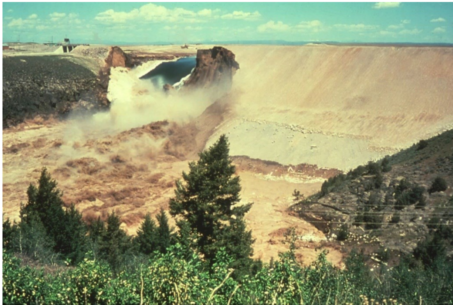
Figure 2.10. Failure in Teton Dam, 1976 (Bureau of Reclamation, www.usbr.gov )
