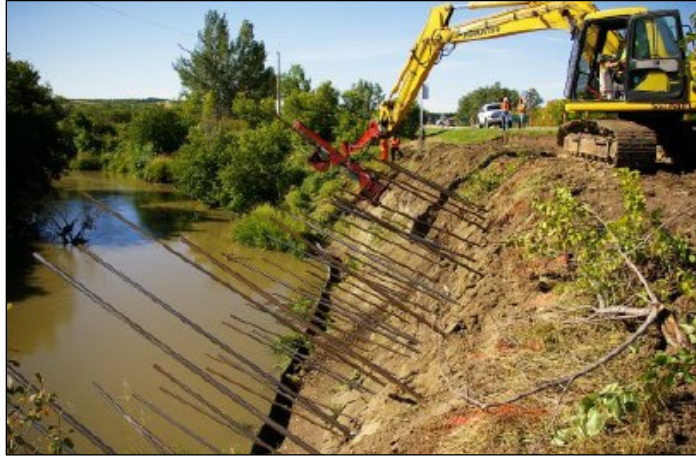
Figure 2.49. Installation of soil nails (Titi and Helwany, 2007)
