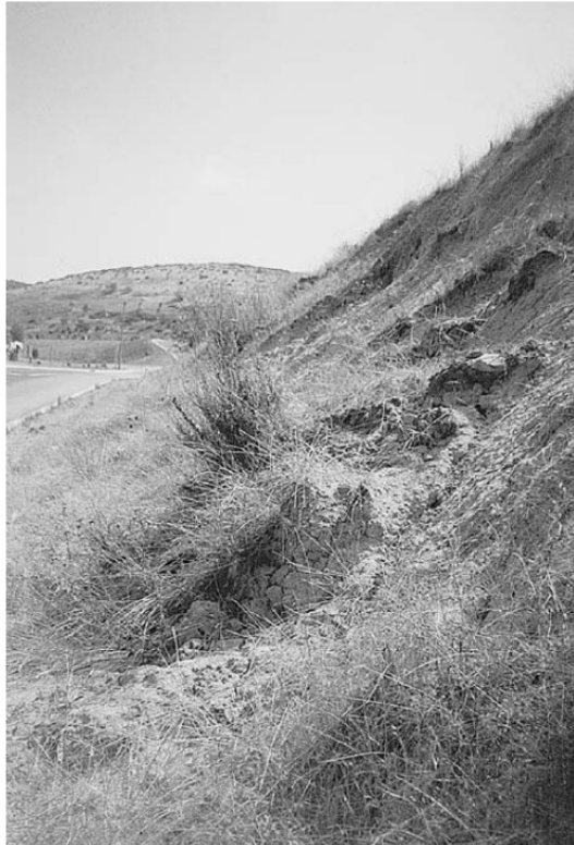
Figure 2.27. Surficial failure, cut slope for road in Poway, California (Day, 2010)
