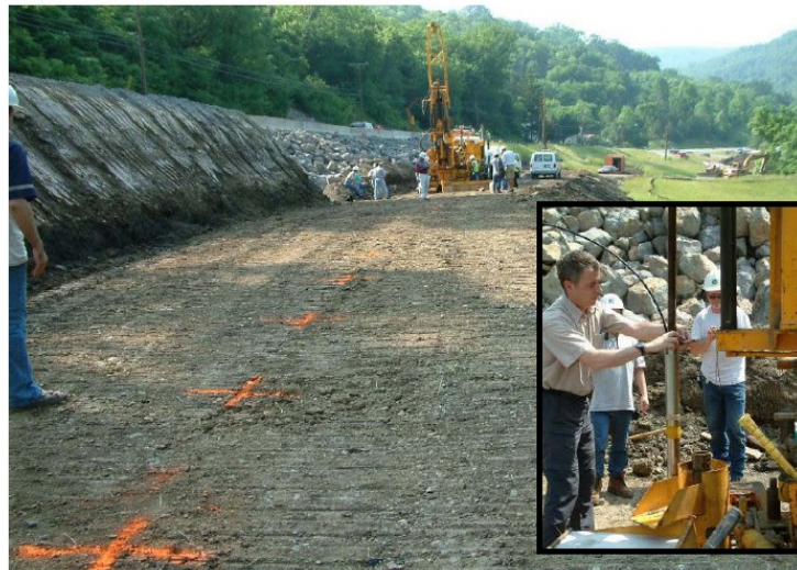
Figure 2.58. JEF-152 Failed Slope under Repair (Liang 2010)
