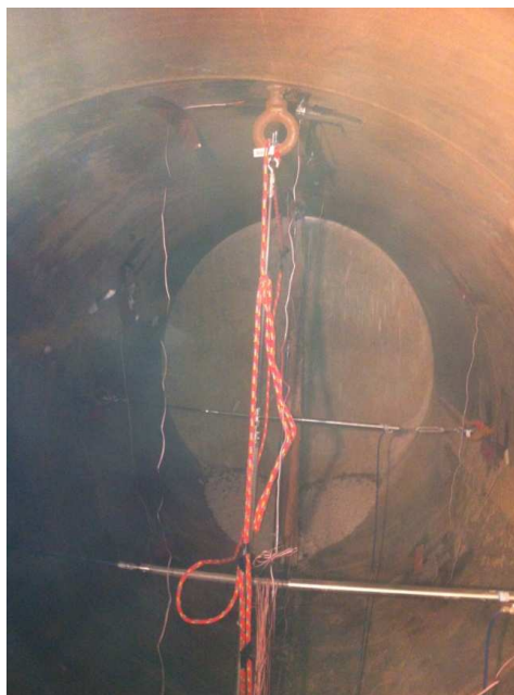
Figure 5.15: Peaking of Pipe during Test 4
