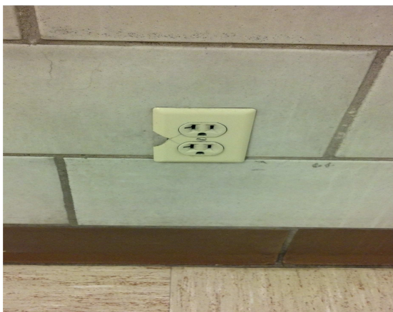
Figure 4.14 Broken Wallplate
