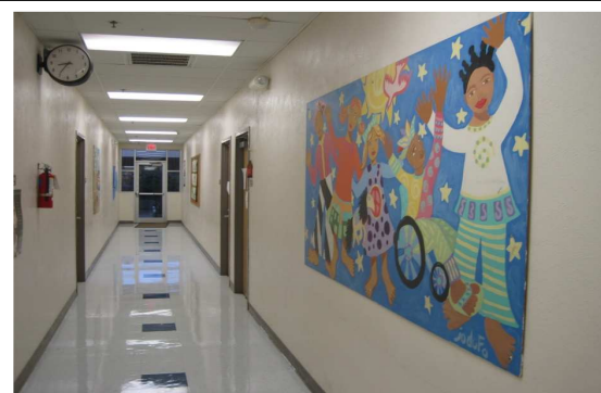
Figure 4.44 Former Department Store “Transformed” With Color
