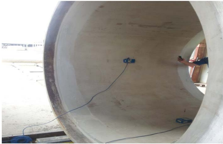
Figure 2.8 CDs attached to the PCCP-ECP
