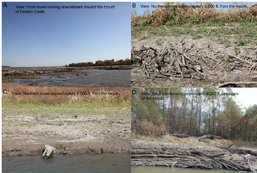
Figure 3-20 Wood debris on and within the levees (images A-D). Image A shows woody debris trapped on the emerging levee. Images B-D show buried woody debris at the base of the levee. Image D also shows woody debris contained within the upper sandier portions of the levee.
