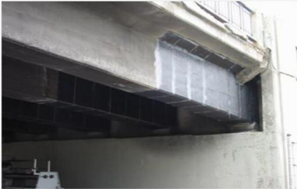
Figure 1.6 Girders being reinforced with Tyfo SCH-41 FRP sheets ( www.fyfeco.com ).
