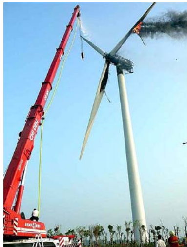
Figure 5.1 Wind generation unit at fault
