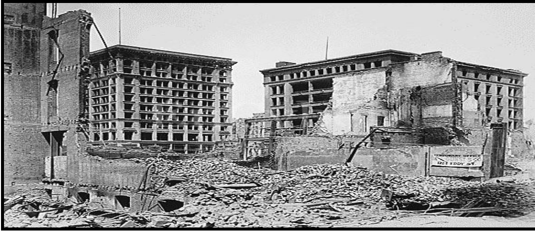
Figure 1.1 Failure of Concrete Building by Earthquake
