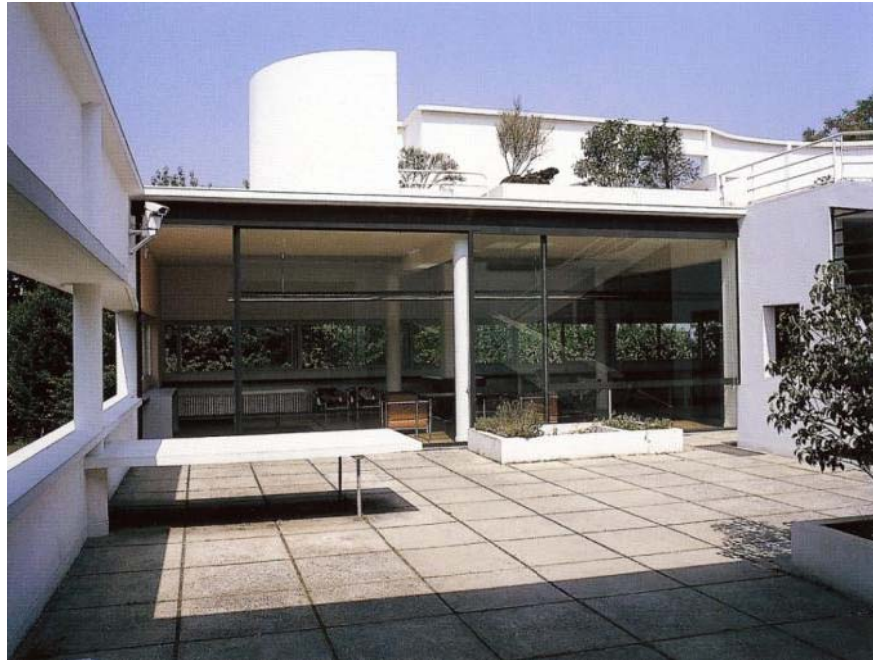
Figure F.10 View from Terrace to Salon 300
