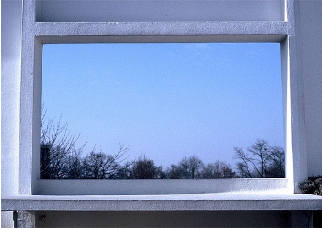
Figure F.15 Villa Savoye Window at Roof Terrace www.flickr.com
