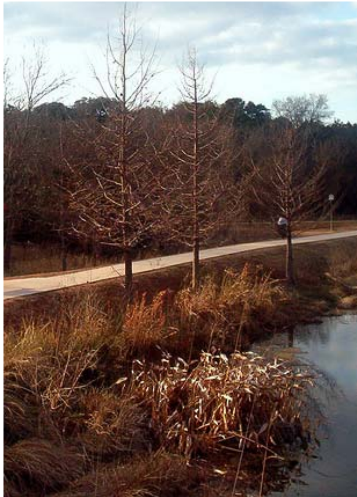
Figure 2.4 Example of a retention pond.
