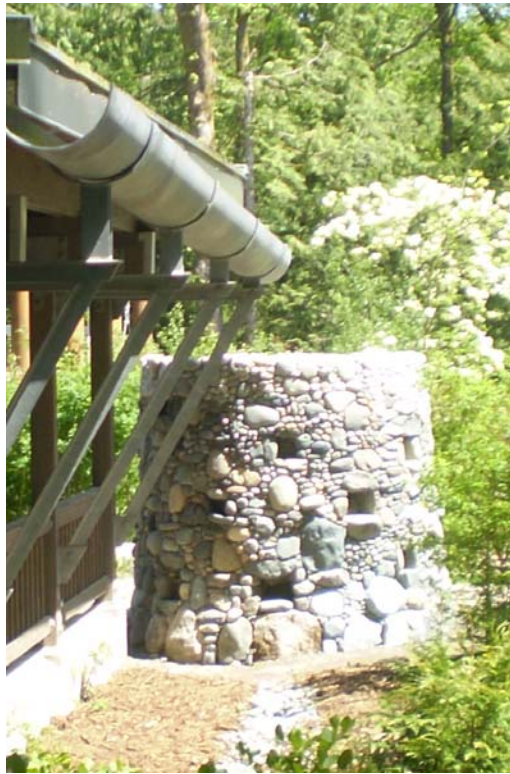
Figure 2.5 Example of rainwater harvesting at Islandwood Learning Center on Bainbridge Island off the coast of Seattle, Washington.
