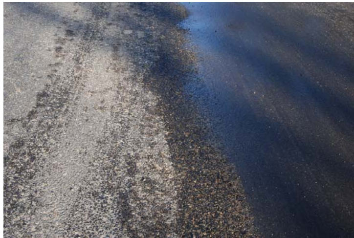
Figure 2.1 Example of permeable paving on the left versus impermeable paving on the right.
