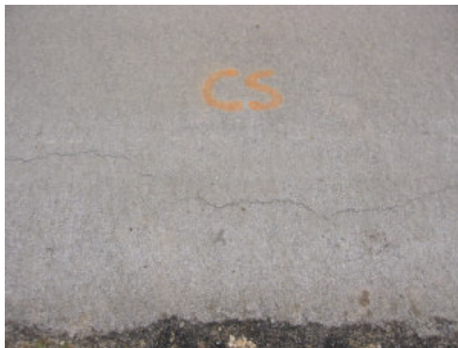
Figure 5.16 Paved shoulder on Apr 2003
