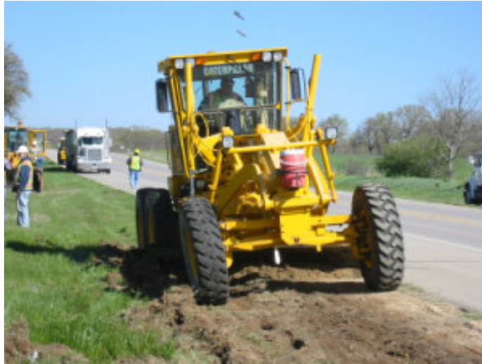
Figure 4.2 Maintainer to blade the subgrade shoulder
