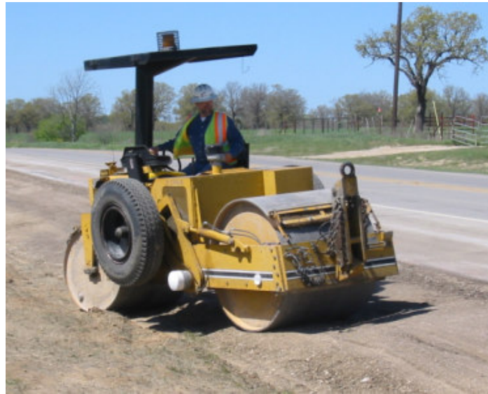
Figure 4.6 Smooth drum roller used for soil compaction
