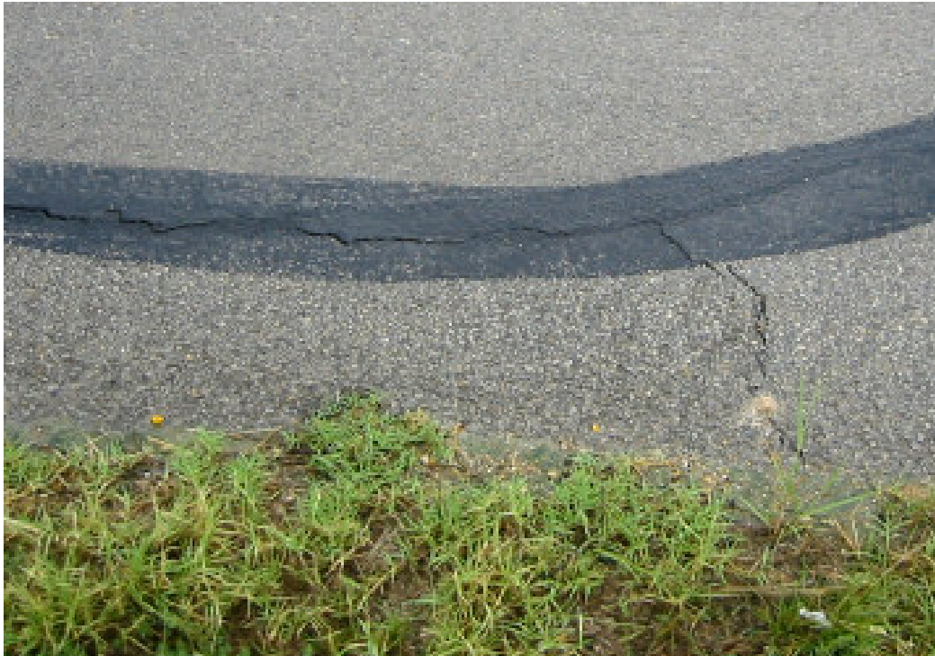
Figure 6.6 Shrinkage of the asphalt concrete
