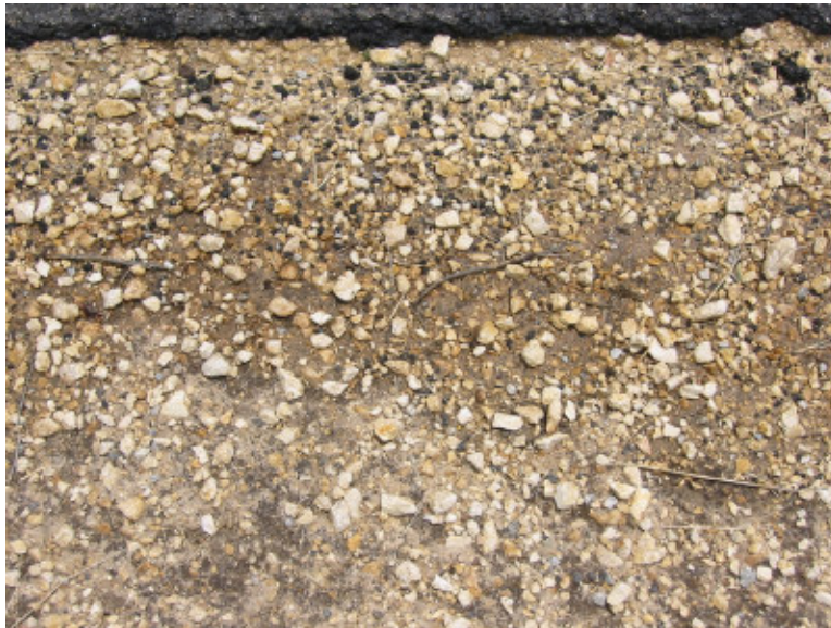
Figure 5.10 Soil surface 3 months after construction (DMC)
