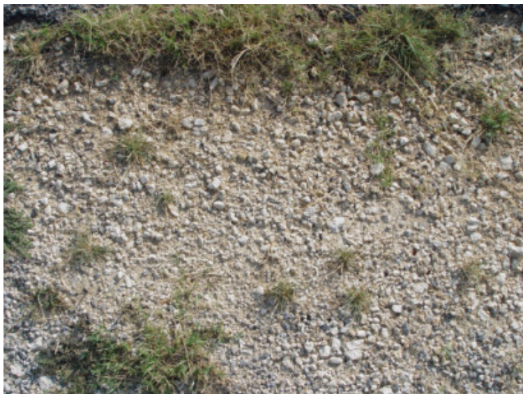
Figure 5.8 Soil surface 3 months after construction (CONTROL)
