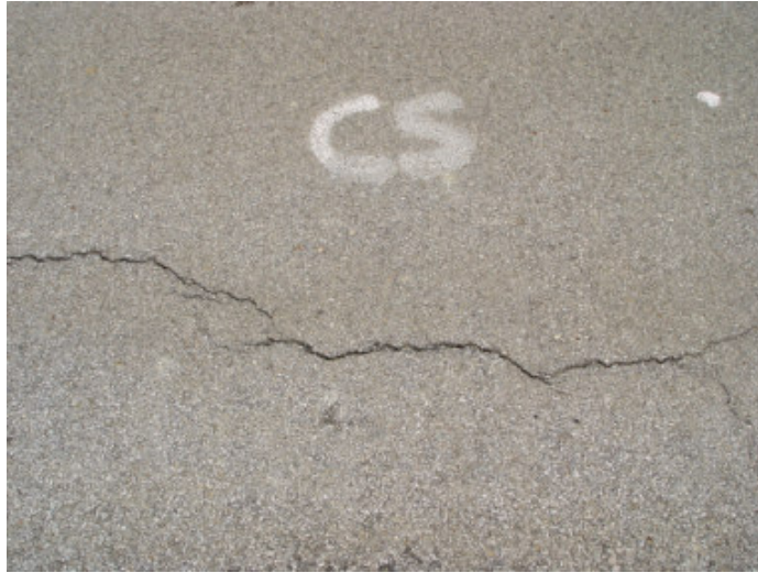
Figure 5.17 Paved shoulder on Apr 2004
