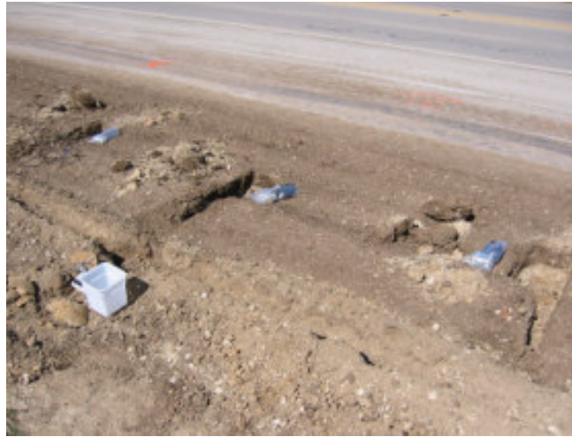
Figure 4.7 Placement of sensors in a test section
