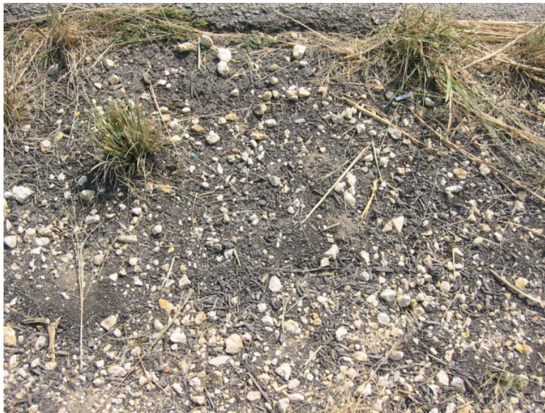
Figure 5.12 Soil surface 3 months after construction (BSC)
