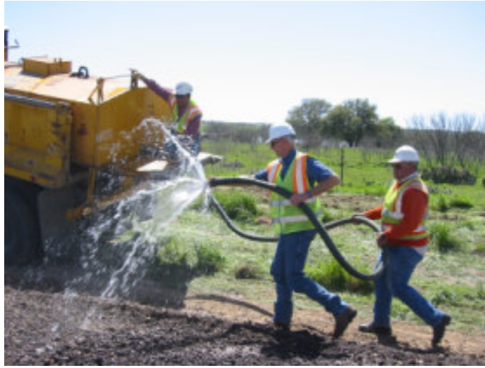
Figure 4.5 Application of water over the CMT loose mixture
