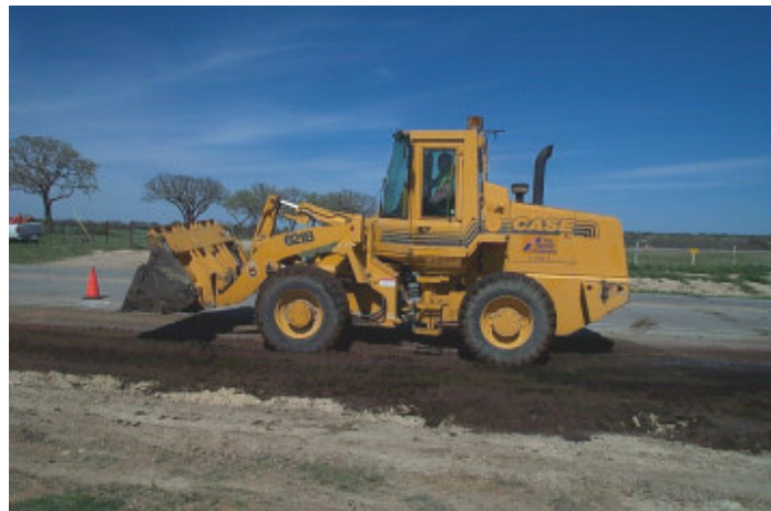
Figure 4.4 Distributing composts on the tilled test plot
