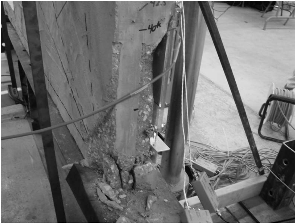
Figure 3-19 Right support of RC test specimen at 60 kip
