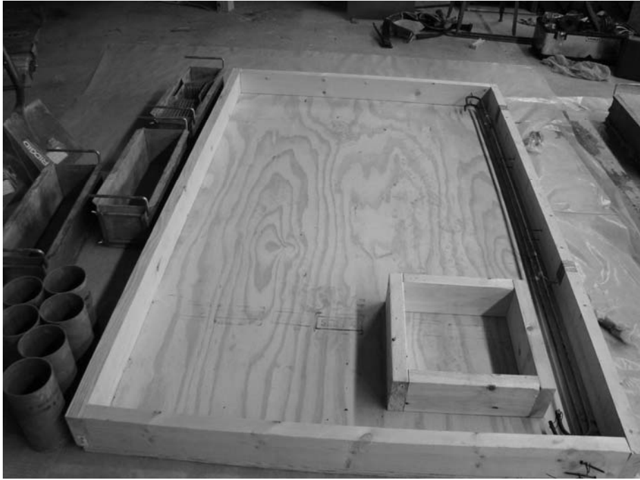
Figure 3-28 SFRC test specimen before casting
