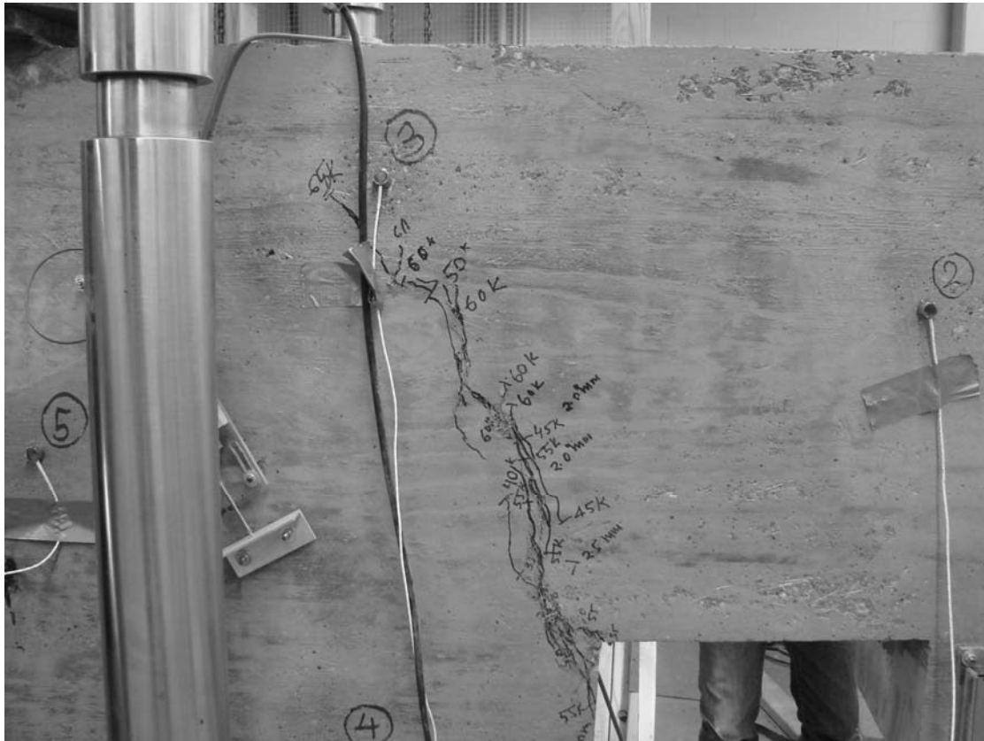
Figure 3-35 Diagonal crack of SFRC specimen at ultimate load (back face)
