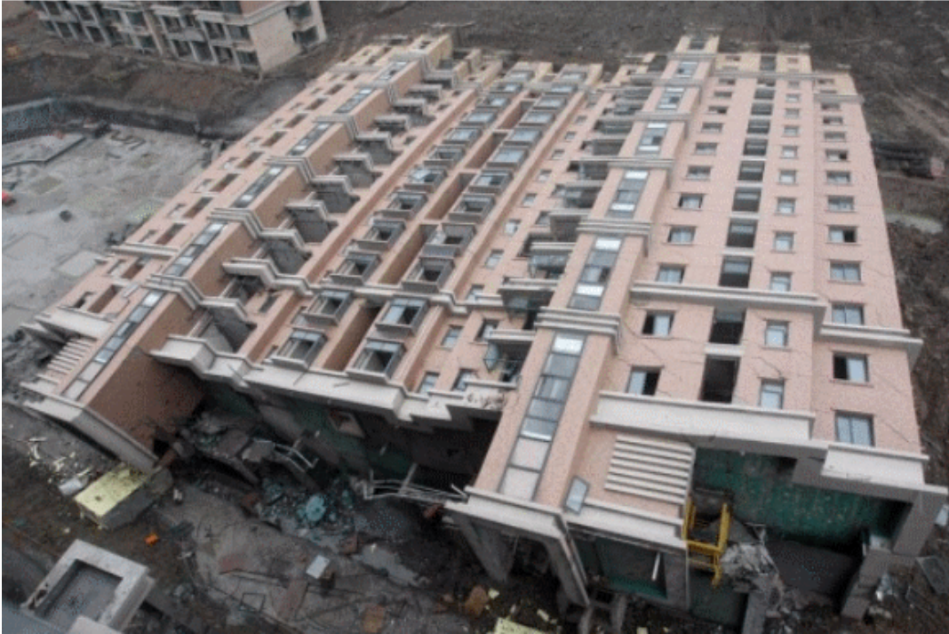
Figure 4.4 Building in Shanghai, China that collapsed in June 2009 (Cress, 2009)
