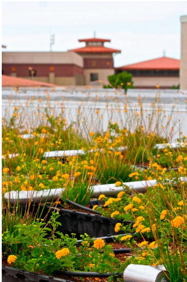
Figure 2.4 Detail of The Modular Tray System used on the Extensive Green Roof at the University of Texas at El Paso
