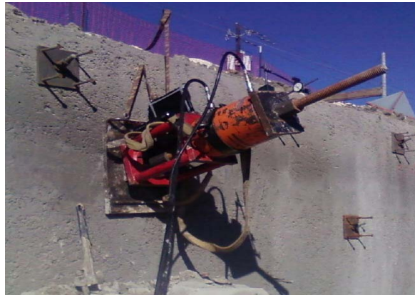
Figure 2.5: Verification testing equipment and setup (Trinity Infrastructure, Inc.).
