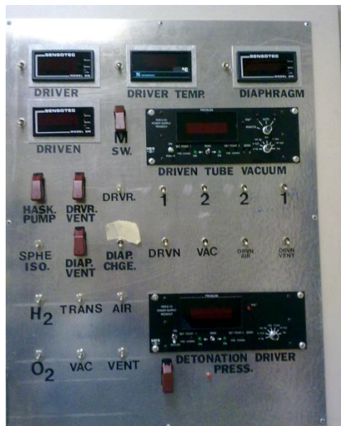
Figure A.1 Picture of control panel for UTA hypersonic shock tunnel.
