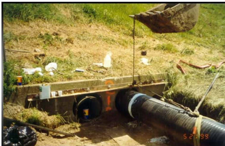
Figure 1.8 – Sliplining Installation (Source: http://www.midwestmole.com/slip-lining.php , Accessed on 10/24/2013)
