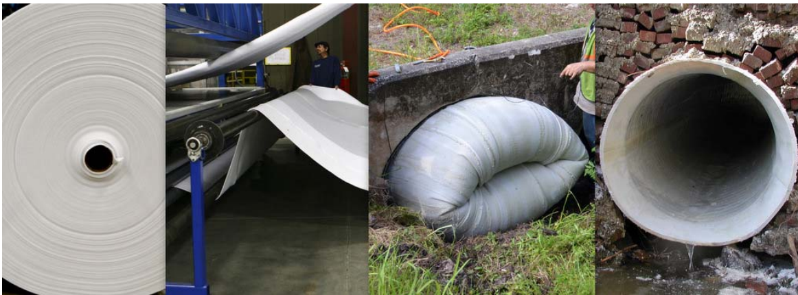
Figure 1.6 – CIPP Installation (Source: http://prod.inliner.net/Brands/Inliner-Technologies.aspx , Accessed on 10/25/2013)
