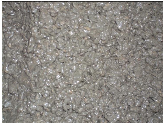
Figure E-3 Geopolymer Concrete Mix with Crumb Rubber
