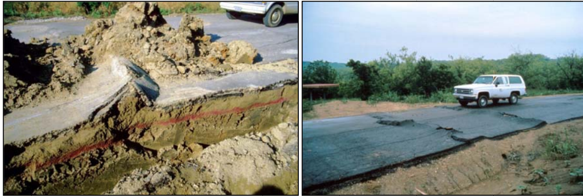
Figure 2.6 Severe Pavement Distress on Pavements close to Joe Pool Lake Dam, Texas (Talluri, 2013)
