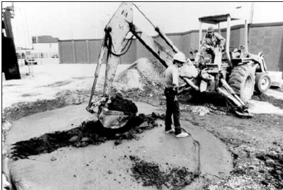
Figure 2.3 Excavating CLSM with a Backhoe (Source: ACI 229R-99, 2005)
