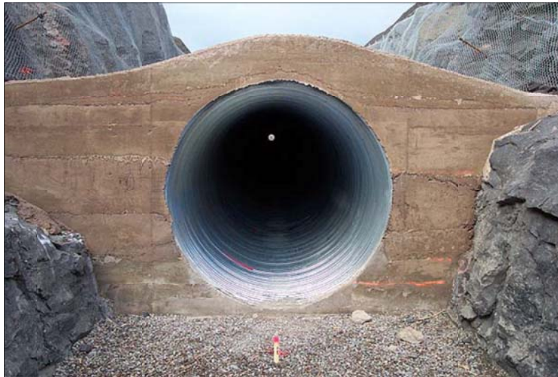
Figure 2.2 Endview of Pipeline with CLSM (Howard and Bowles, 2008)
