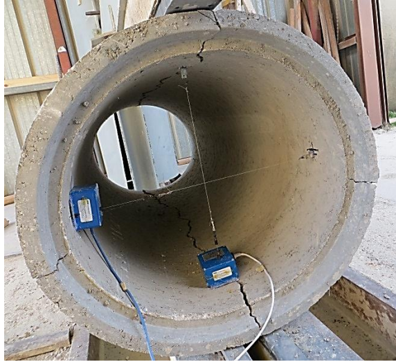
Figure 3-8 Cable Displacement Sensors (CDS) Positioning
