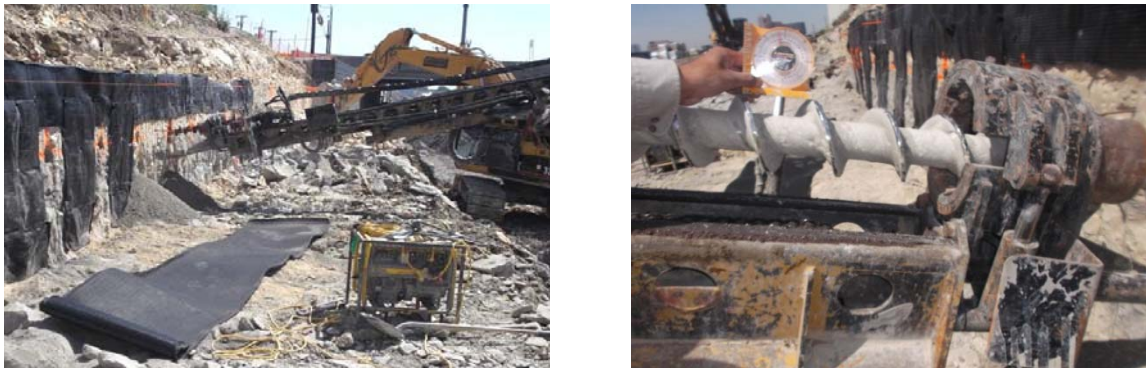
Figure 2-10 (a) Drilling operation for Rock Nail walls and (b) Detail of drilled holes inclination check prior to reinforcement placement and grout injection. QA/QC is essential. (personal pictures archive 2013)
