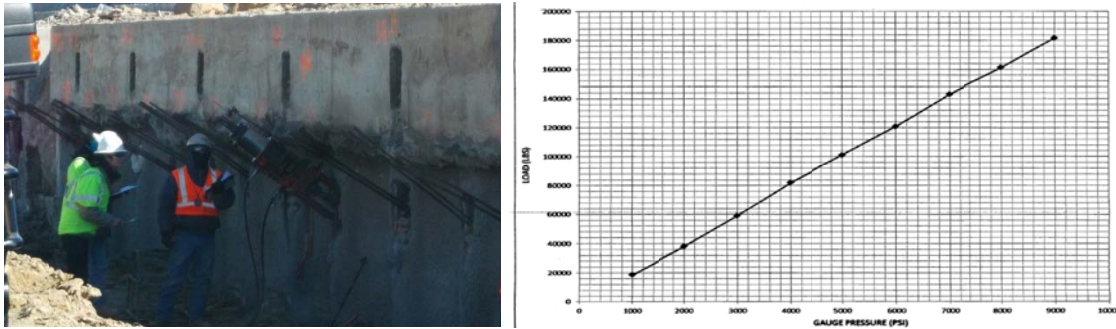
Figure 2-37 (a) Wall 3 anchor testing and (b) load-pressure curve (archive 2014)
