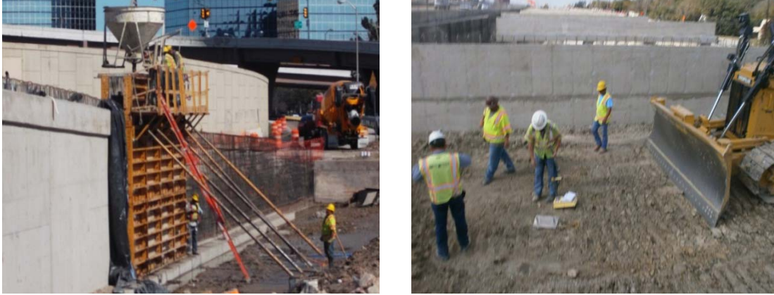
Figure 2-30 (a) Cast in place wall placement and (b) subgrade preparation (archive 2013)
