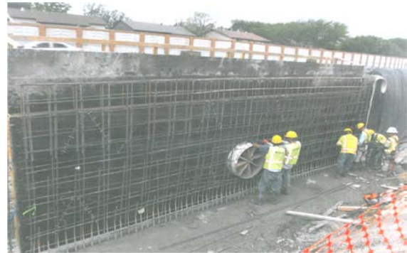
Figure 2-13 (a) Rebar cage in drill shaft prior to concrete placement. (b) Rebar placement for cantilever cast in place wall stem. (personal pictures archive 2011)
