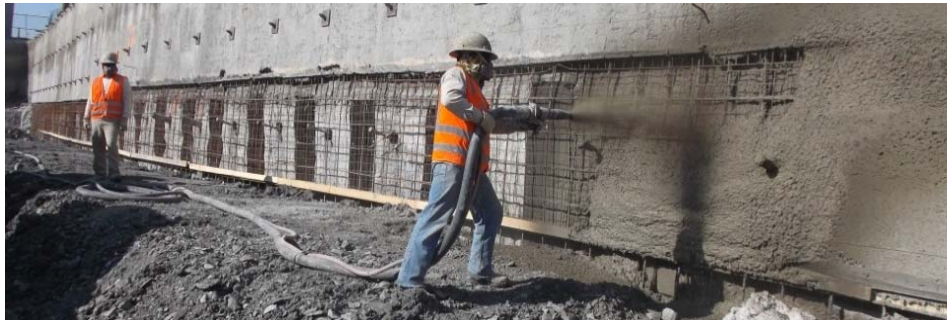
Figure 2-17 Nozzle operator placing shotcrete in rock nail wall (wet) (personal archive 2013)
