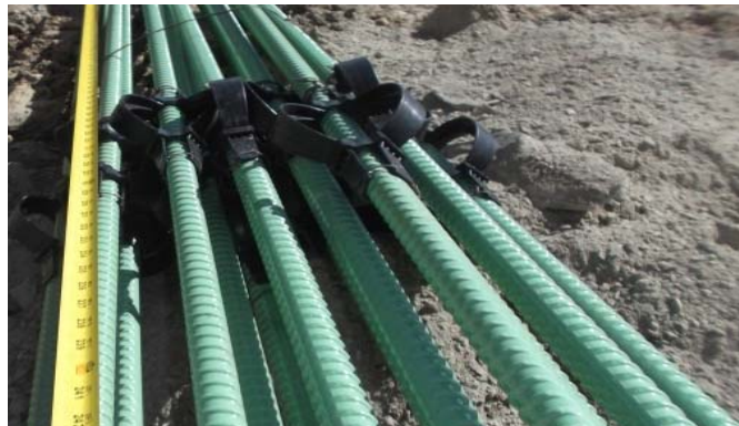
Figure 2-33 Epoxy coated protection for soil/rock nail bars in Wall 2 (archive 2013)
