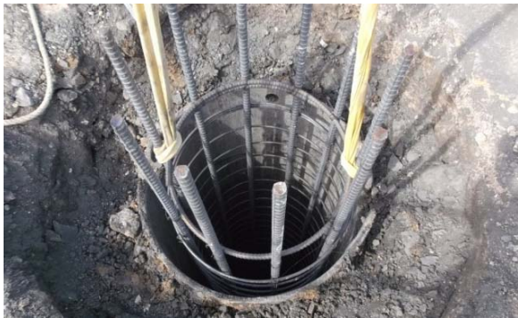
Figure 2-13 (a) Rebar cage in drill shaft prior to concrete placement. (b) Rebar placement for cantilever cast in place wall stem. (personal pictures archive 2011)
