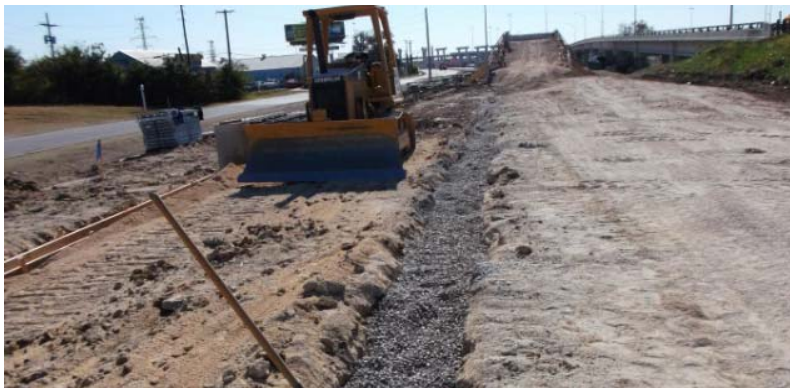
Figure 2-8 Underdrain for MSE Wall drainage and subgrade preparation (personal archive 2013)
