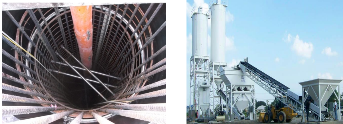
Figure 2-19 (a) Detail of tremie tube inside of rebar cage to place the concrete (avoid segregation and soil intrusion) and (b) concrete Batch Plant (personal archive 2011 and www.gulfatlanticequipment.com )
