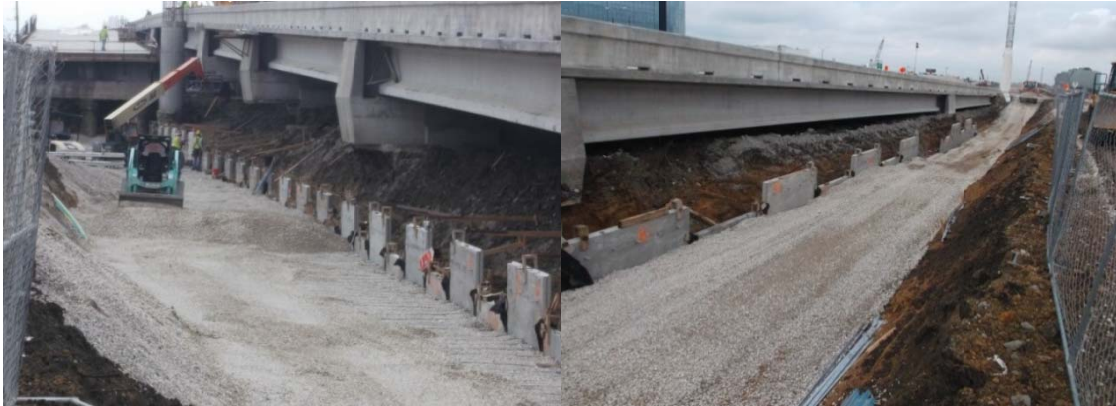
Figure 2-20 Backfilling operation in MSE Wall. (personal pictures archive 2013)
