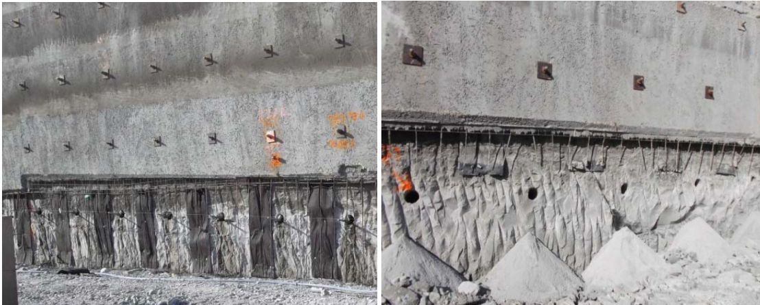
Figure 2-31 Rock Nail drilling and drainage operations (personal archive 2013)
