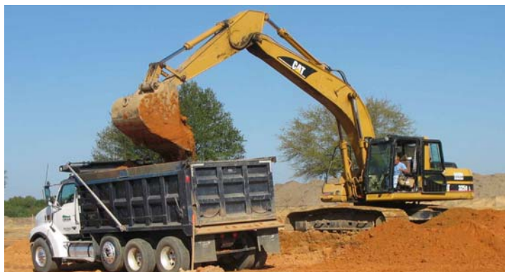
Figure 2-12 Hydraulic hoe loading spoils in a rigid frame dump truck. (logansitework.com)
