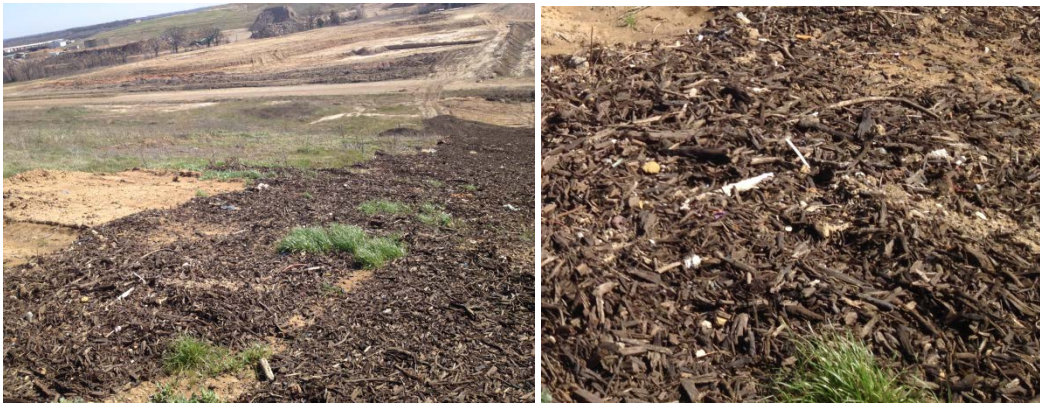
Figure 4.36 Mulch Cover on the Slopes of the City of Denton Landfill
