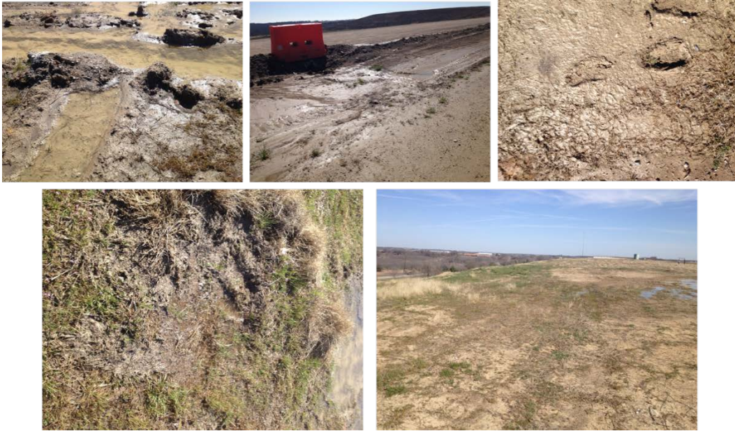
Figure 4.30 Cover Soil Condition during the Methane Emission Monitoring in Dec'13 and Jan'14
