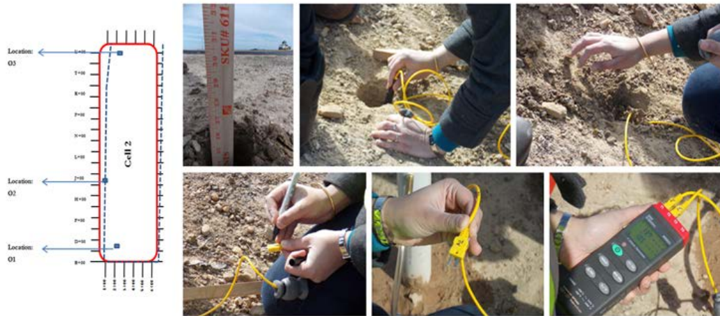
Figure 3.11 Locations, Installation and Monitoring of Soil Temperature at the Cover
