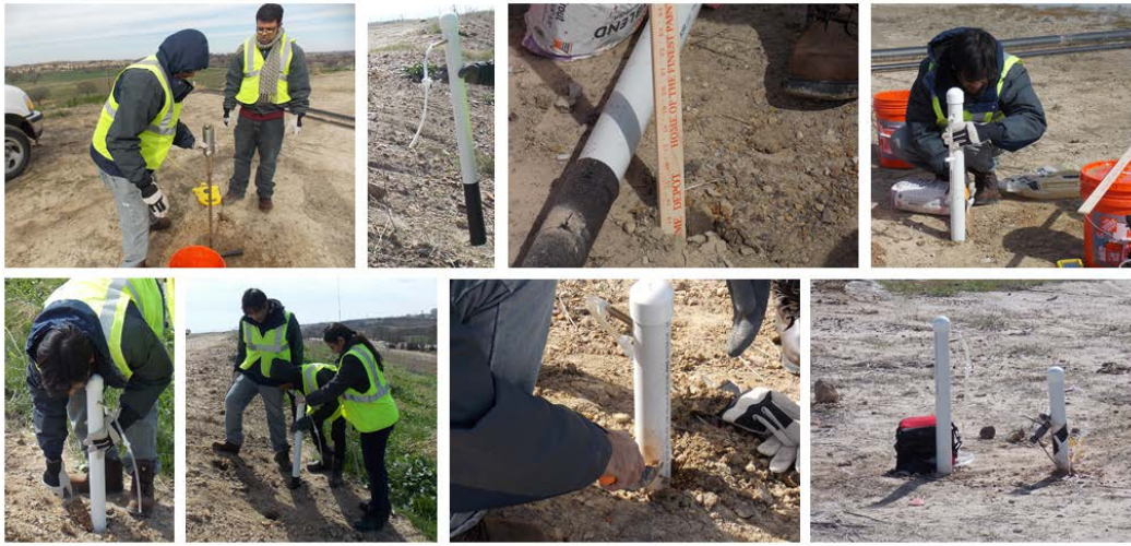
Figure 3.19 Oxidation Pipe Installations
