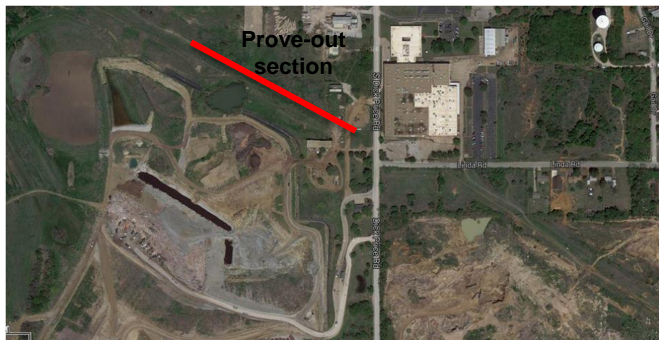
Figure 2-1 Aerial view of the prove-out section and site location
