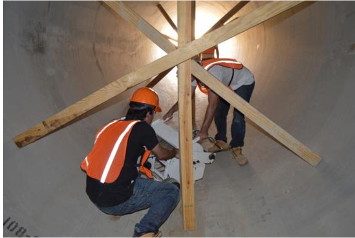
Figure 2-20 Movement of instrumentation for placement within the pipeline
