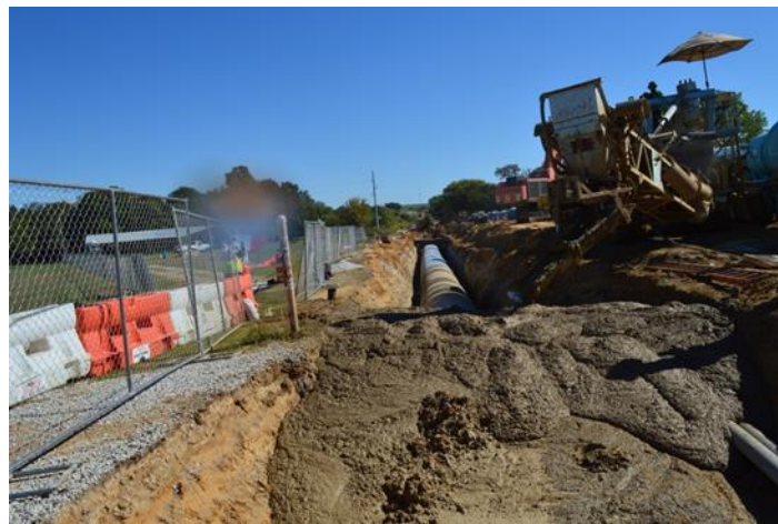
Figure 2-40 Sample CLSM produced by the automated travelling batch plant
