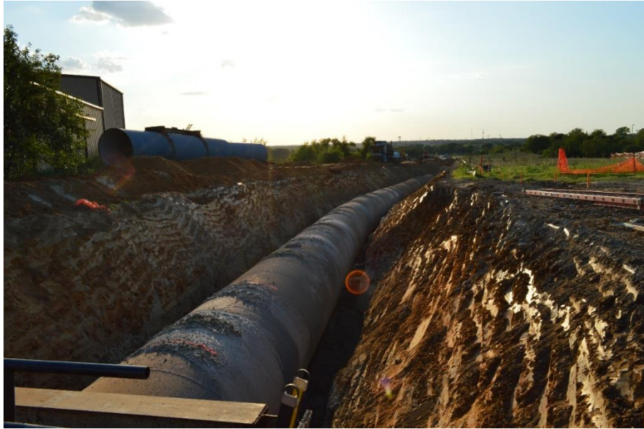
Figure 2-4 Placement of pipeline within trench
