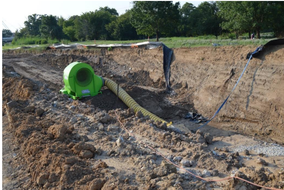
Figure 2-6 Blower unit used in the prove-out section
