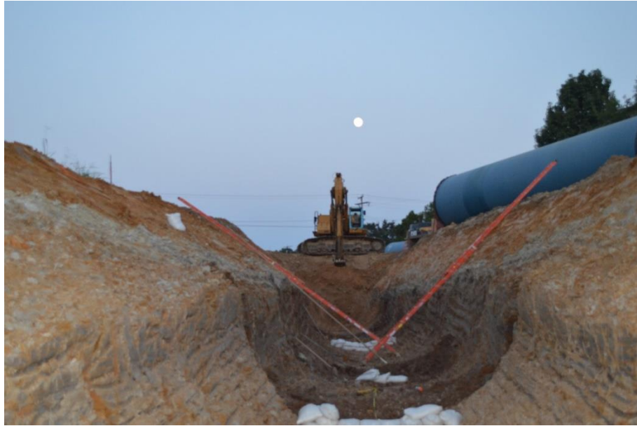
Figure 1-5 Trench configuration used in the section J of IPL
