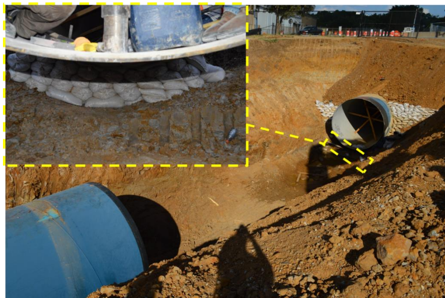
Figure 1-3 Sandbag placement beneath pipe
