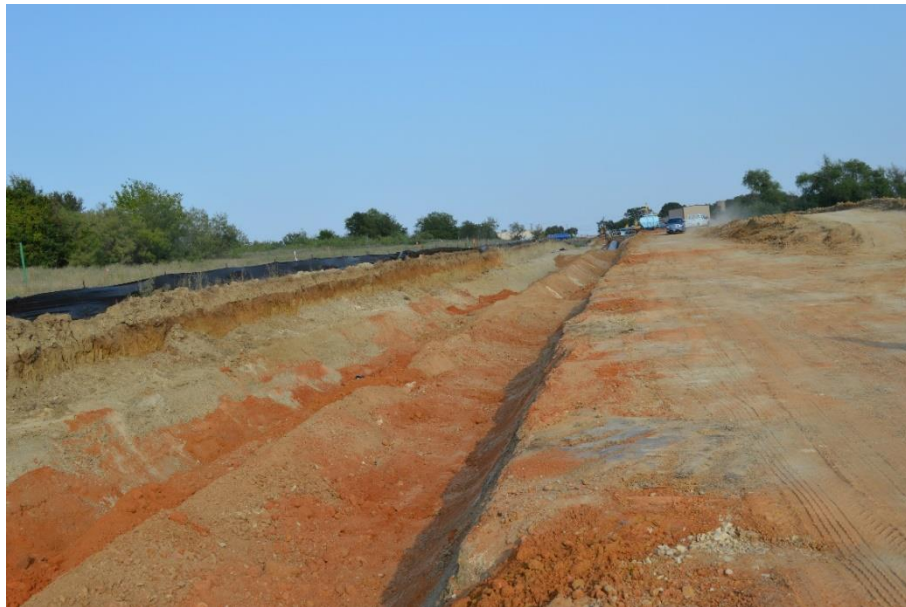
Figure 1-4 Backfilling of prove-out section using native soil
