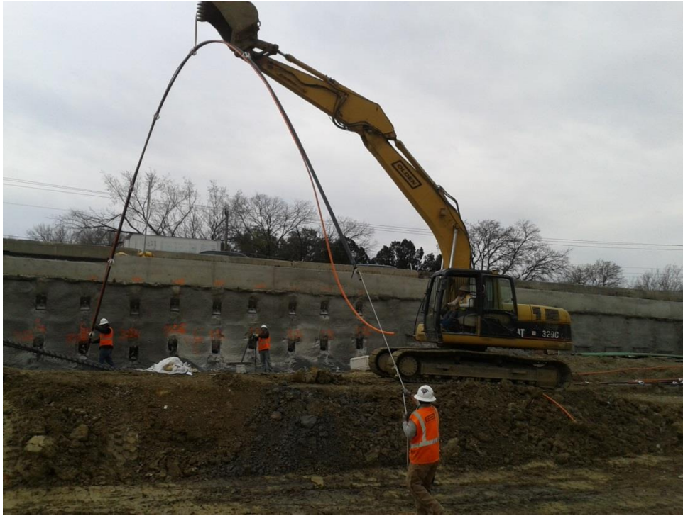
Figure 2.21 Steel bar tendon insertion
