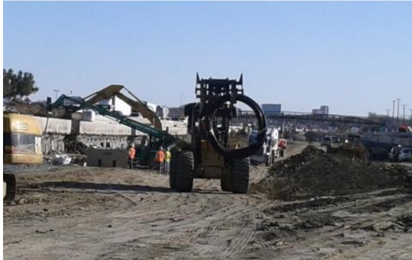
Figure 2.15 Loader handling a strand anchor (Personal picture, January 13th, 2014).
