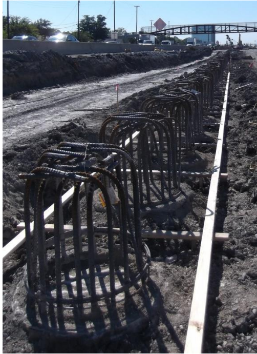
Figure 2.10 Preparation of drilled shaft for construction of cap beam (January 10 th , 2014)
