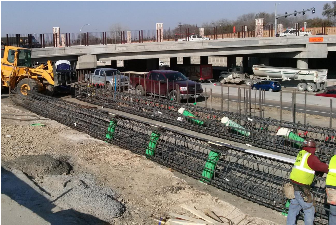
Figure 2.5 Trumpet installation on drilled shaft reinforcing steel
