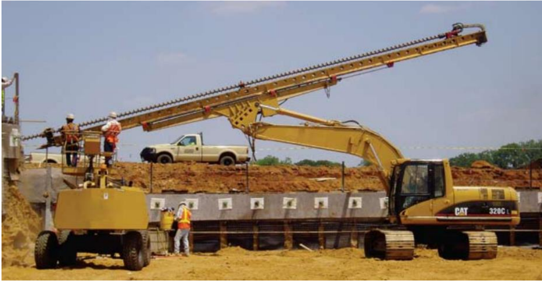
Figure A.5 Excavator mounted drill (HEM-40ED Soil Nailing Drill, TEI Rock Drills)
