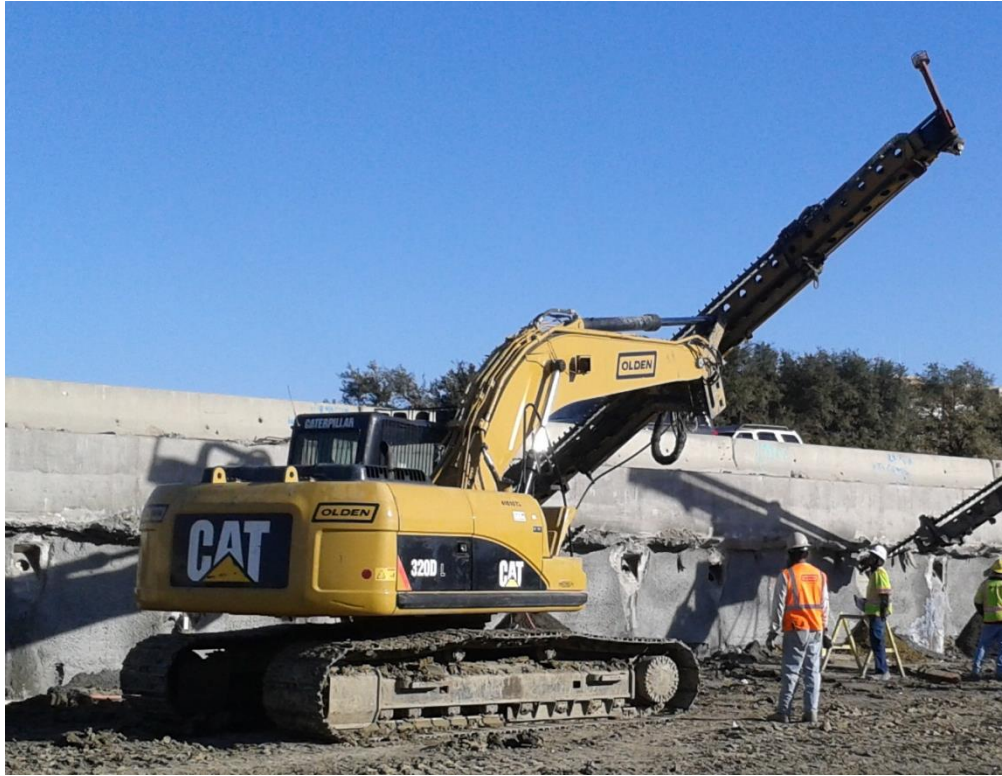
Figure 2.13 CAT 320D with 25 feet excavator mounted drill
