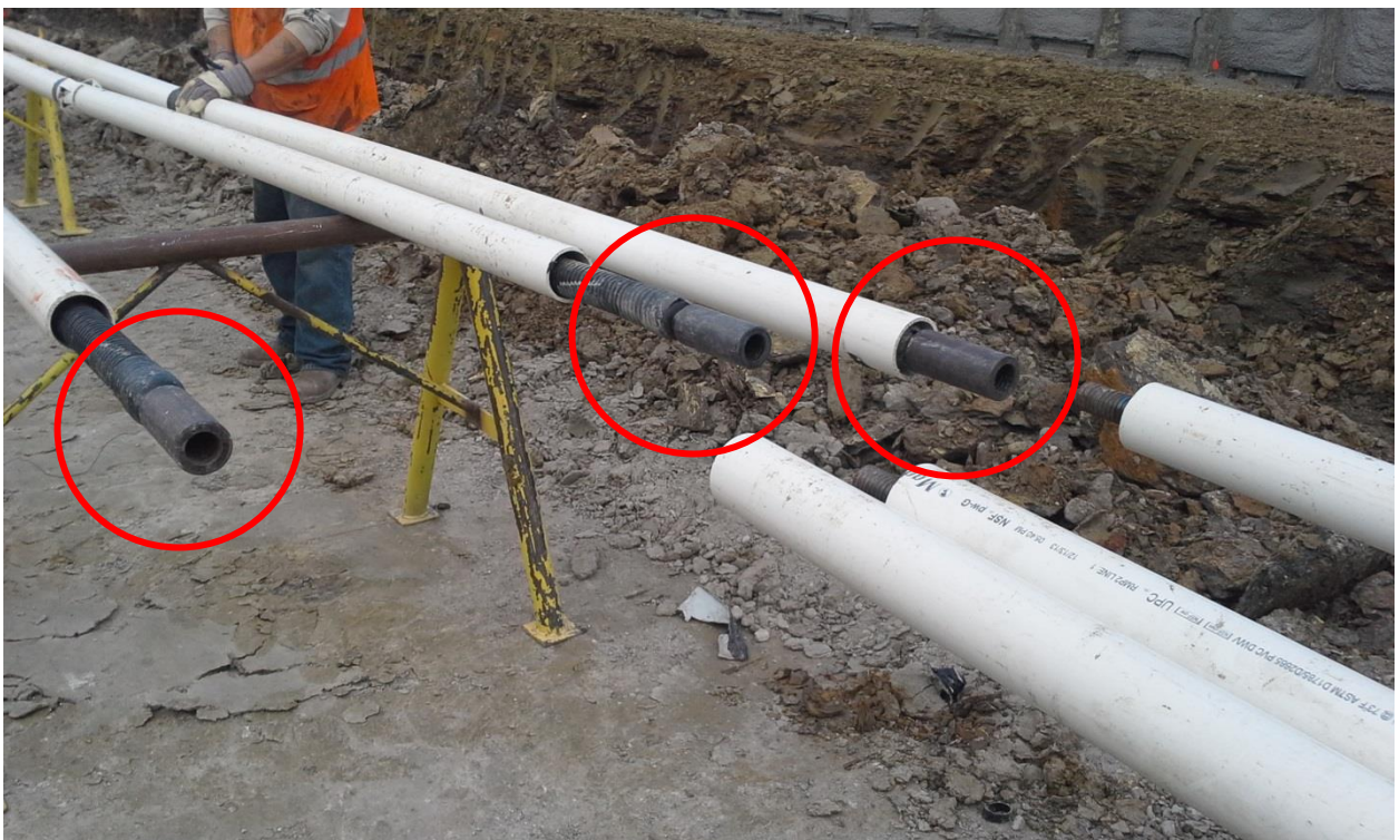
Figure 2.17 Coupler installation
