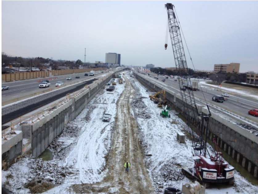
Figure 1.1 Overview of the retaining walls of the "IH-635 Managed Lanes Project."
