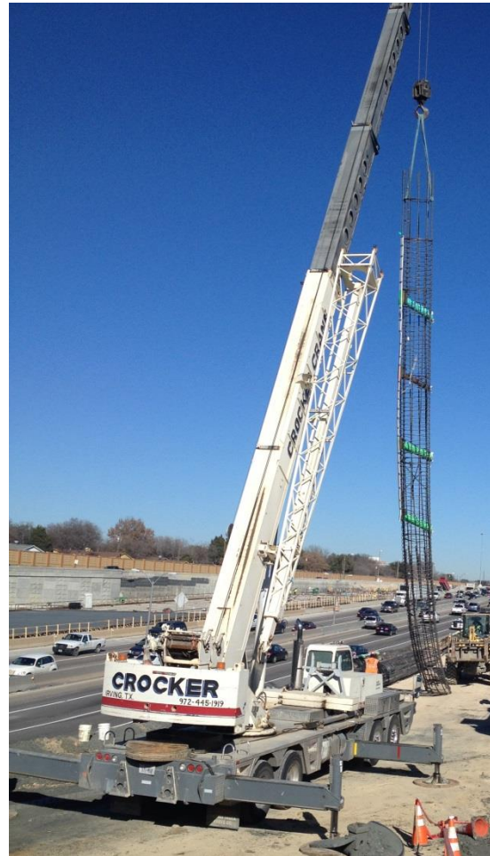
Figure 2.9 Crane picking up reinforcing steel (Personal picture, January 12 th , 2014).
