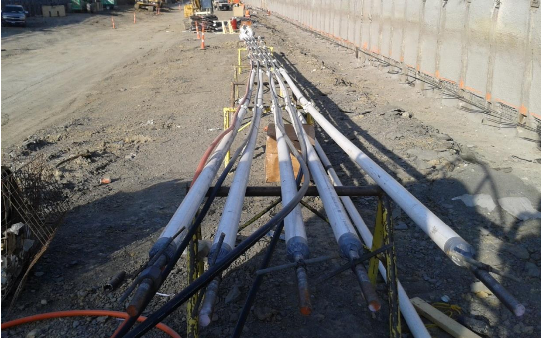
Figure 2.20 Steel bar tendons preparation
