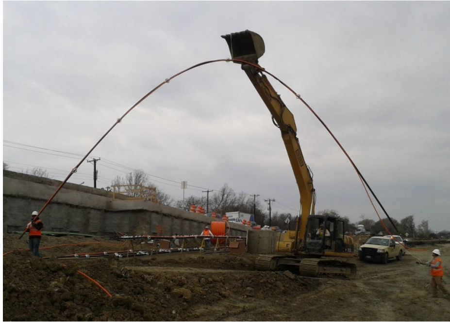
Figure A.3 Excavator handling a 60 feet long steel bar anchor
