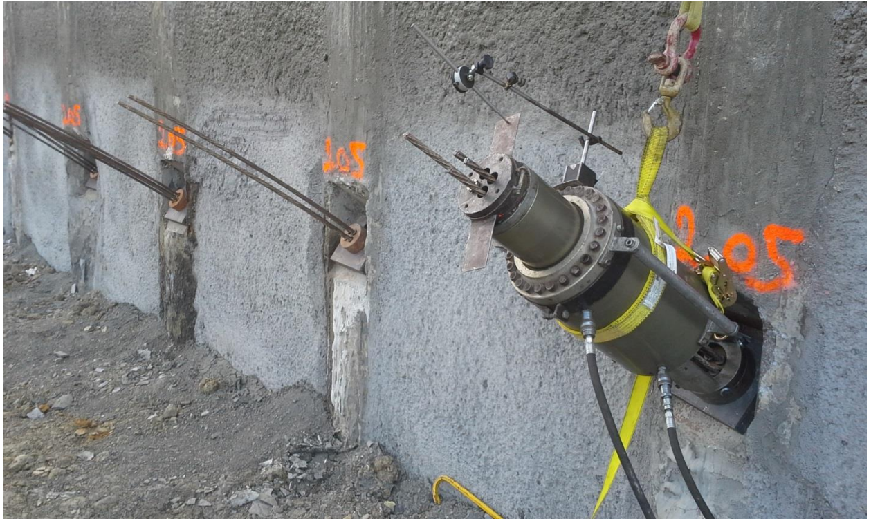
Figure 2.22 Testing a strand anchor (Personal file, February 20 th , 2014).
