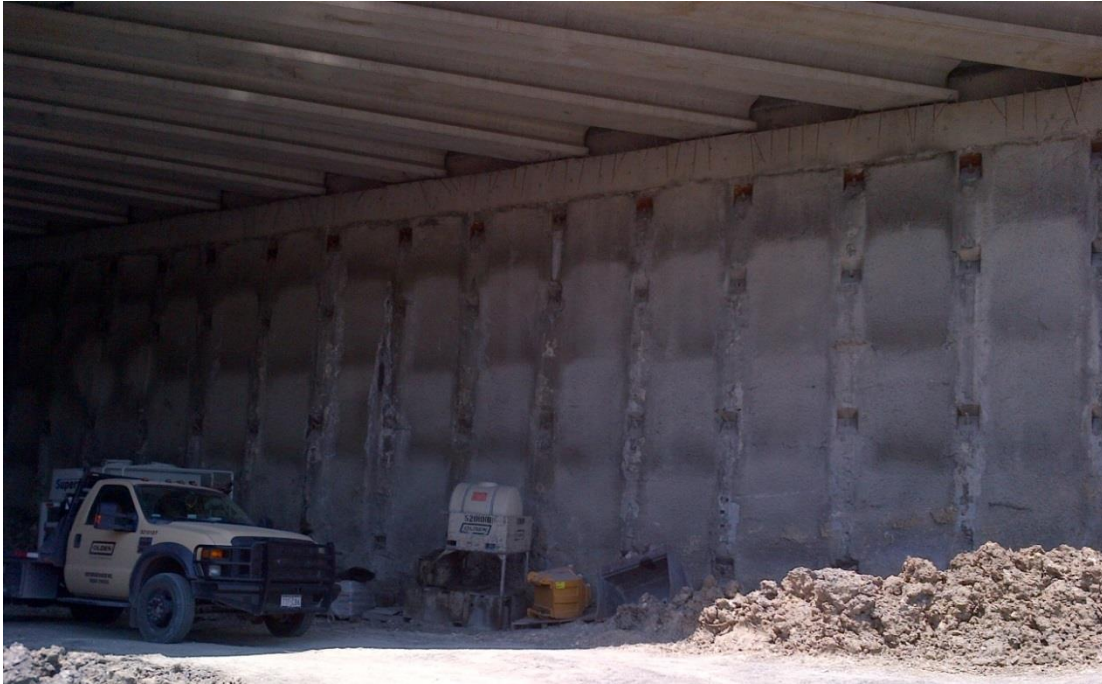
Figure A.16 Location 1 above bridge abutment
