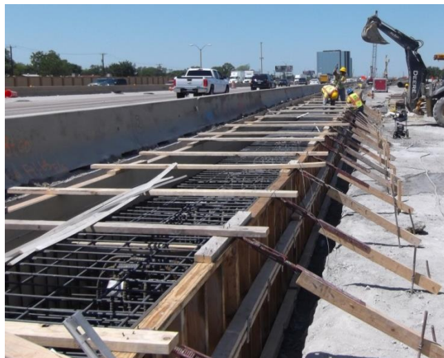
Figure 2.11 Cap beam ready to be poured (Personal file, July 18 th , 2013).
