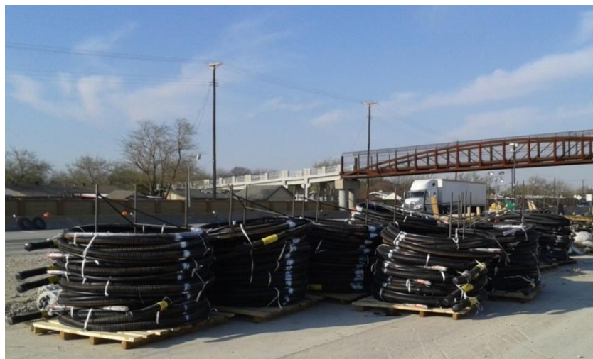
Figure 2.16 Storage area for strand tendons (Personal file, March 24 th , 2014)
