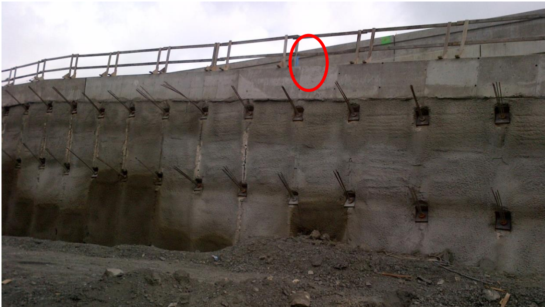
Figure A.17 Location 2
