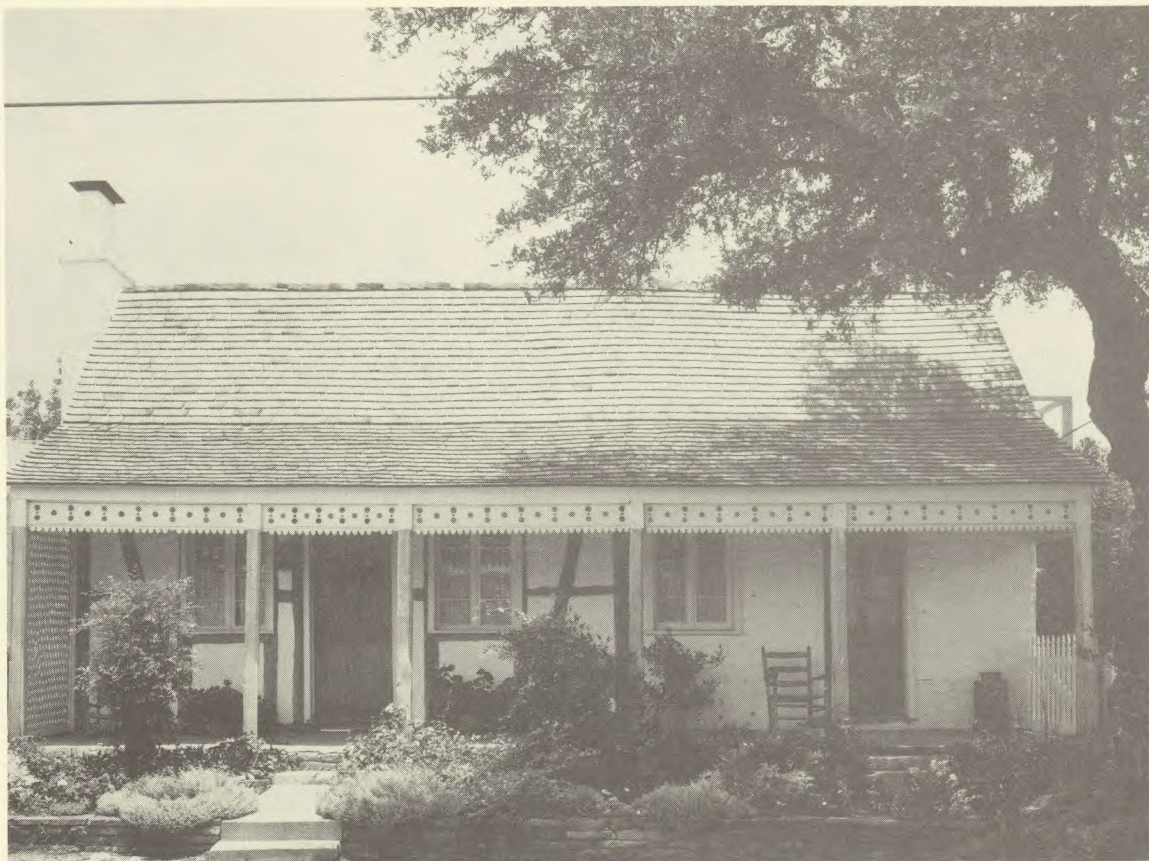
Roberta Smith House, Fredericksburg. Included in Fredericksburg Historic District, 1970. Representative of pioneer German Fachwerk construction.
