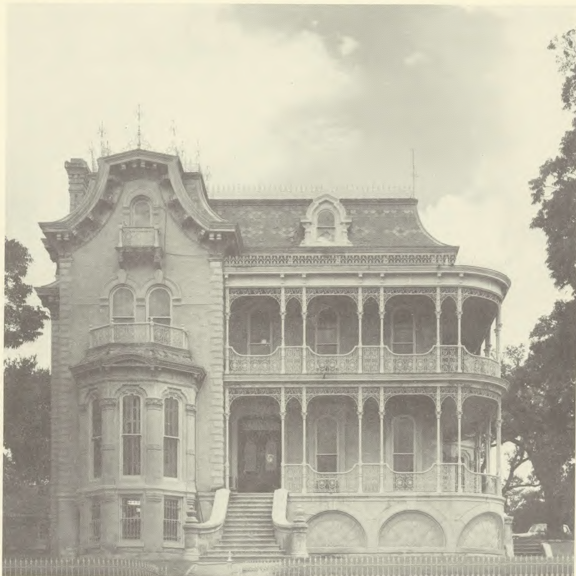
John Bremond House, Austin. Included in Bremond Block Historic District, 1970. A Second Empire mansion with a Mansard roof and outstanding cast iron decorative detail.
