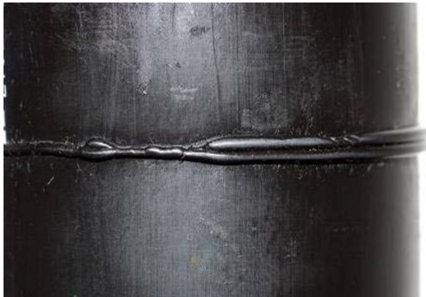
Figure 2.19 Butt Fusion Failure Due to Contamination of Material (PPI, 2008)
