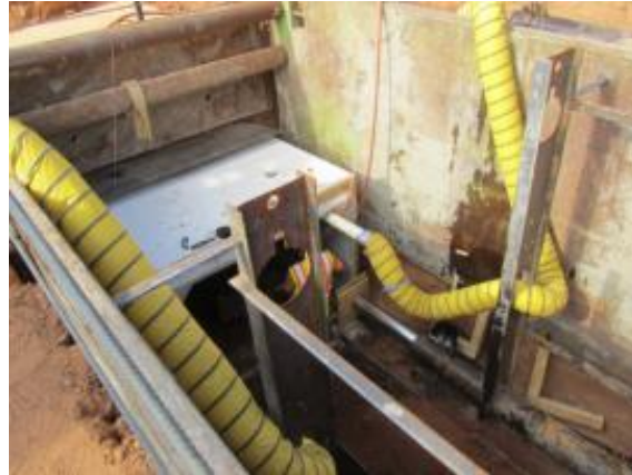
Figure 1-12 Air Supply Lines (Tavakoli, 2012)
