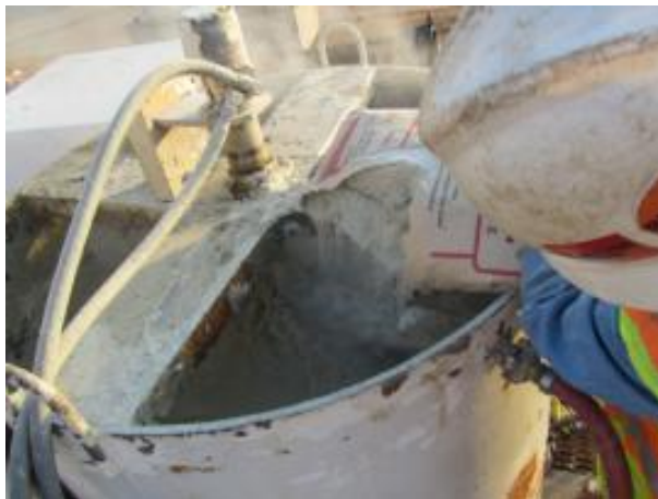
Figure 1-11 Bentonite Lubricant Preparation (Tavakoli, 2012)
