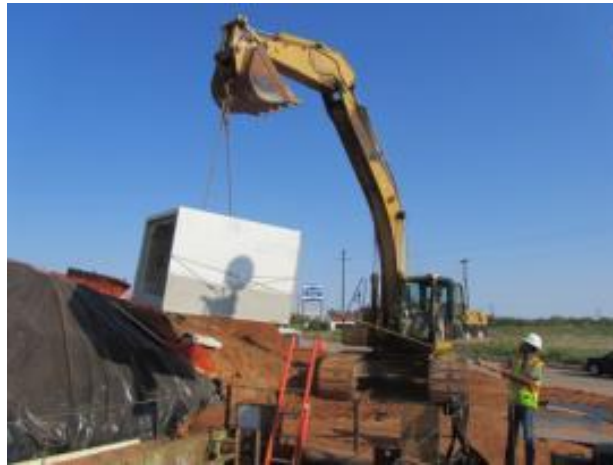
Figure 1-8 Excavator Hoists a Box Section from the Stockpile (Tavakoli, 2012)
