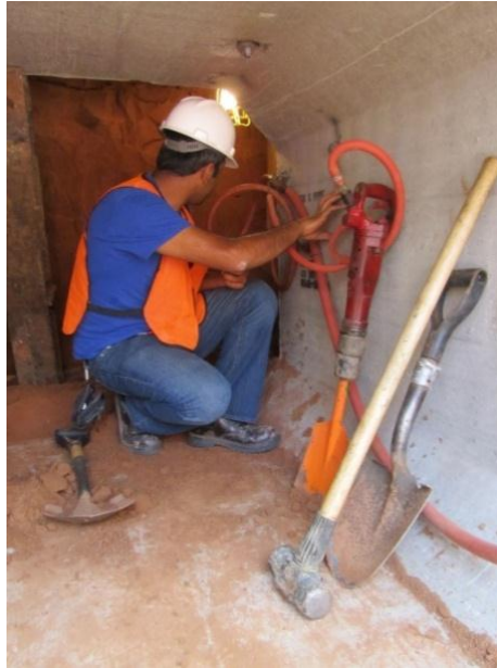
Figure 1-6 Box Jacking (BJ) Operation with Hand Mining Excavation
