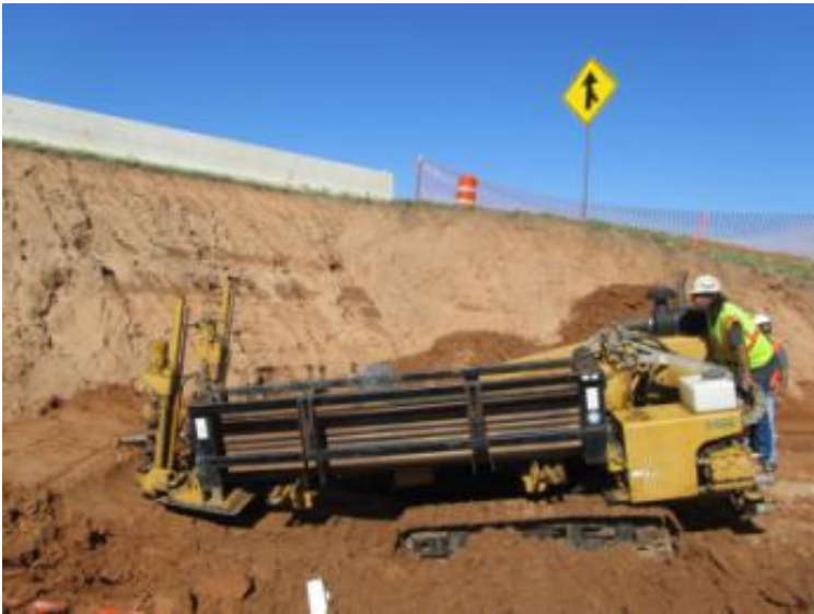
Figure 4-9 HDD Rig Set to Drill Hole (Tavakoli, 2012)
