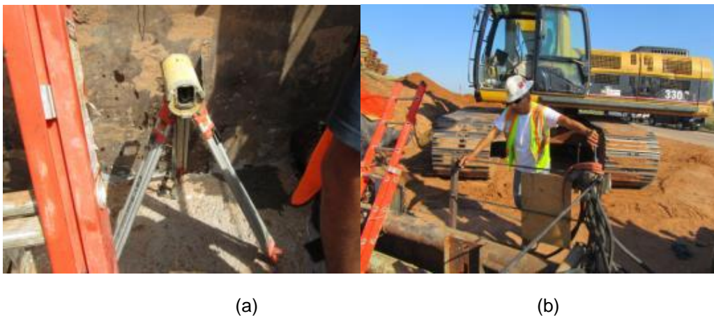
Figure 1-13 a) Laser for Alignment and b) Jacking Control Handle (Tavakoli, 2012)
