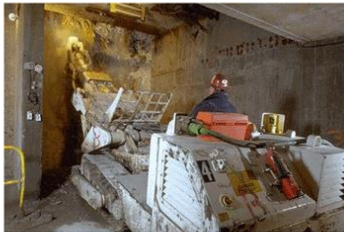
Figure 1-7 Box Jacking (BJ) Operation with Roadheader Excavation
