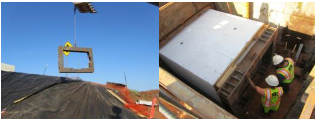
Figure 1-9 Excavator Placing Jacking Frame into Launch Shaft (Tavakoli, 2012)
