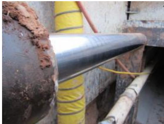
Figure 1-15 Pushing Box by Hydraulic Jacks (Tavakoli, 2012)
