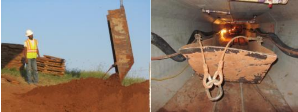
Figure 1-14 a) Excavator Unloads Spoil Cart, b) Empty Spoil Cart (Tavakoli, 2012)
