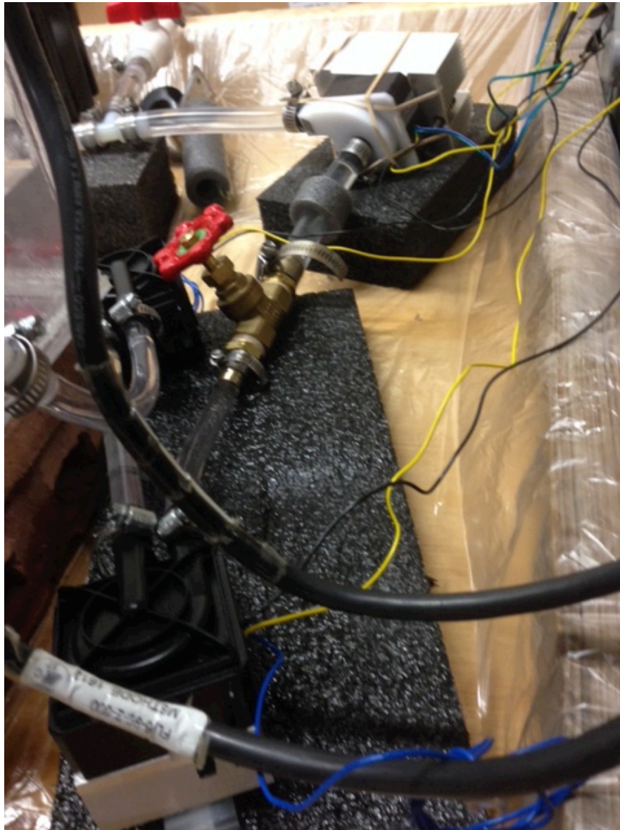
Figure 4-18: Three fans placed in series on the outlet side of the apparatus. Fan sinks are seen attached using rubber bands to prevent overheating.
