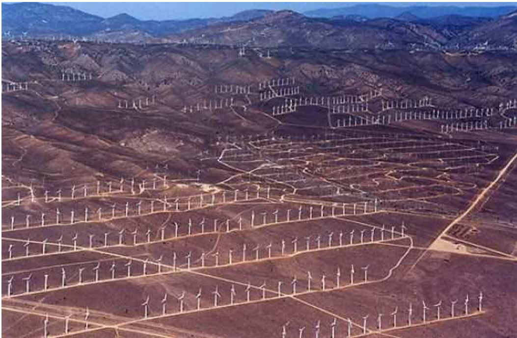
Figure 2-4 Tehachapi Wind Resource Area in California [18]
