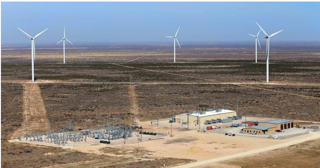
Figure 2-3 Notrees Battery Storage Project in west Texas [14]
