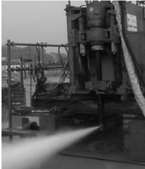
Figure 2.4 High-pressure injections (Brinkgreve R.B.J (2006).
