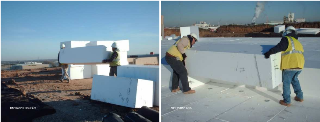
Figure 4.5 Geofoam removal and installation
