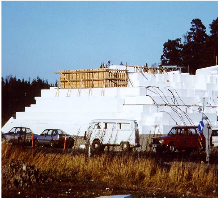
Figure 2.29 Abutment construction on EPS embankment at Lokkeberg Bridge (Frydenlund and Aaboe, 2001)
