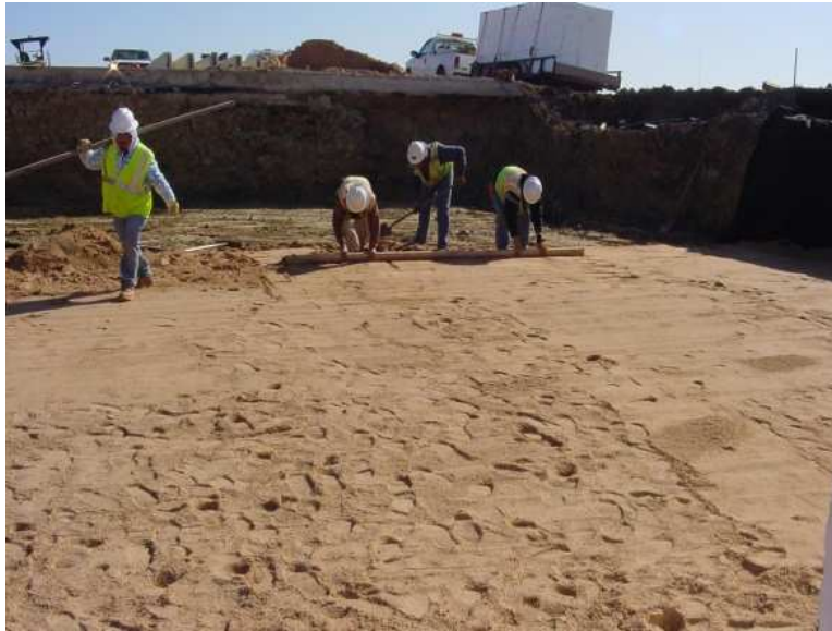
Figure 4.3 Compaction of sand leveling layer
