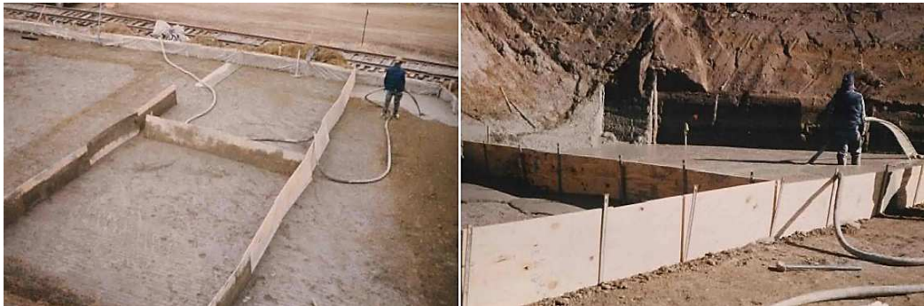
Figure 2.32 Foamed concrete filled in a construction site (NYDOT, 2013)
