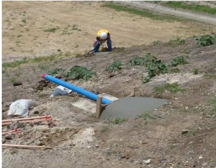
Figure 4.15 Cast-in-place concrete base
