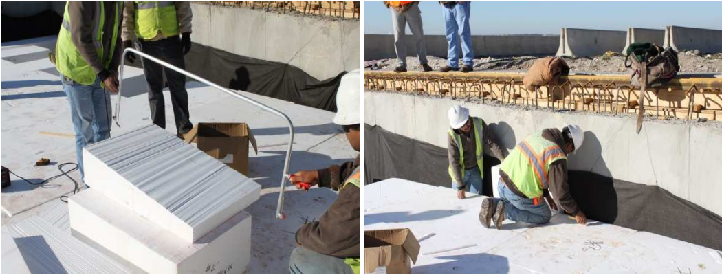
Figure 4.6 Geofoam's shape adjustment for filling in narrow space
