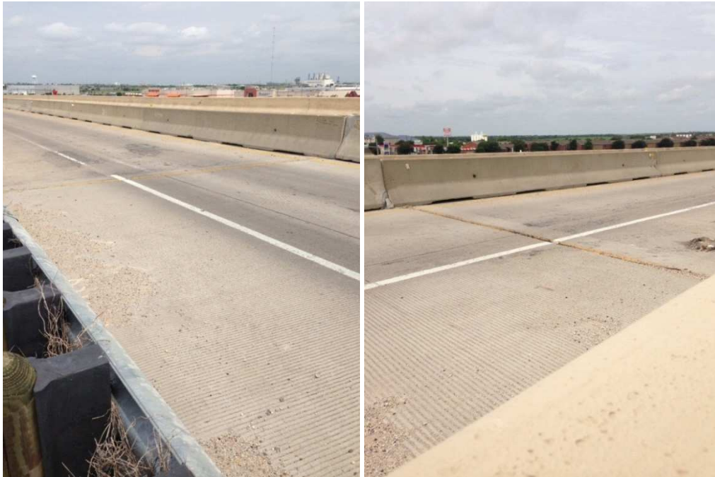
Figure 5.1 Bridge approach slab constructed on the EPS geofoam layer
