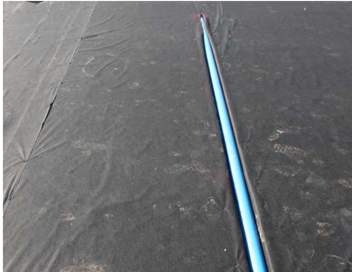
Figure 4.13 Inclinometer casing placed in prepared trench
