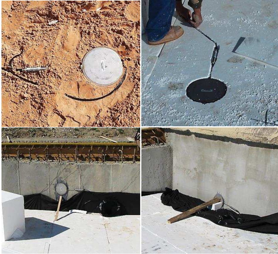
Figure 4.18 The pressure cells installed in the test embankment
