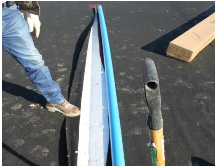
Figure 4.12 Trench prepared for installing the inclinometer casing
