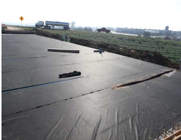
Figure 4.14 Backfilled trenches and covering geomembrane
