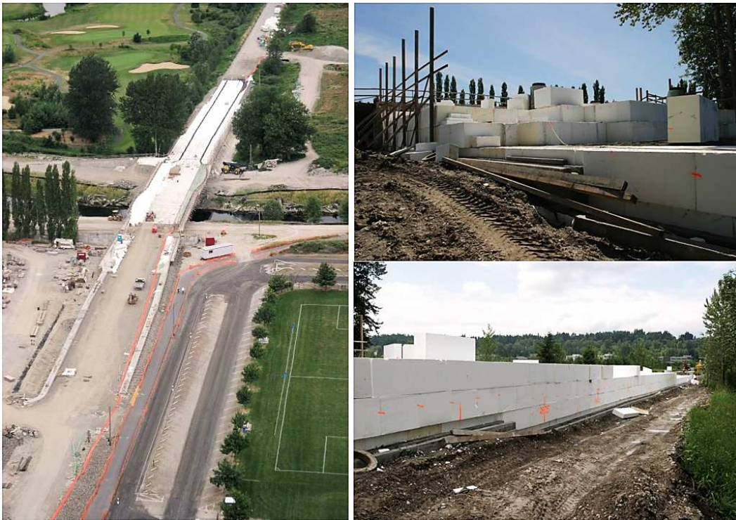
Figure 2.30 Geofoam replacement for York Bridge embankment (Dusenberry and Bygness, 2006)
