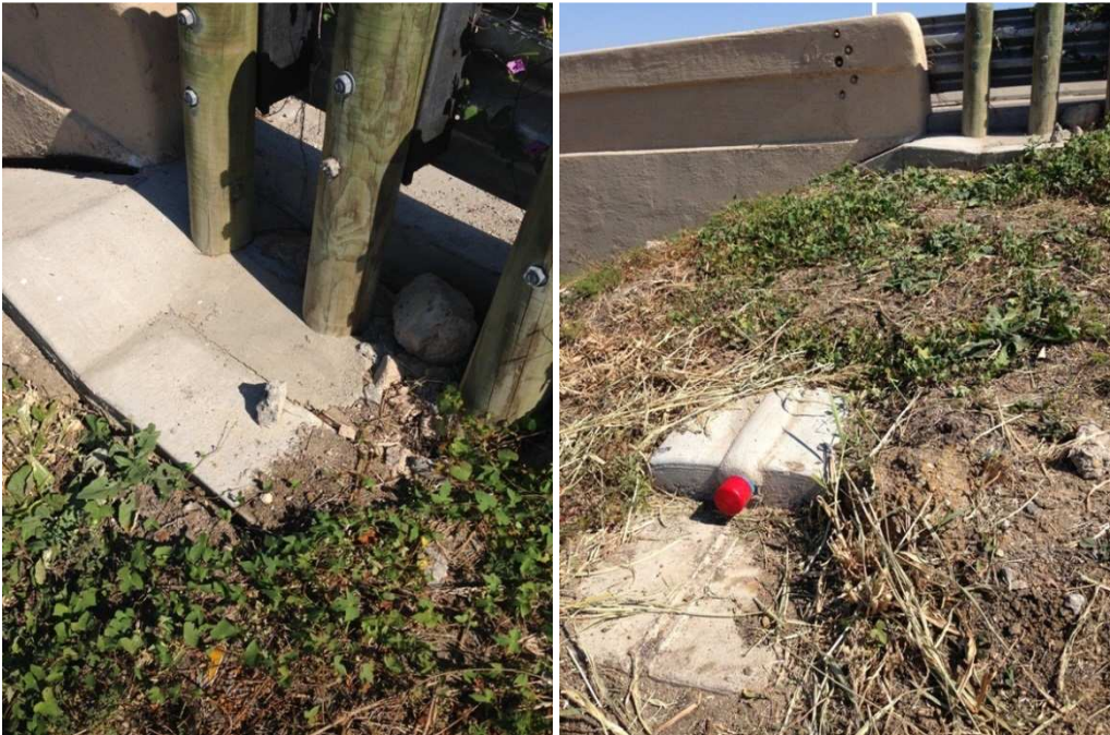
Figure 5.4 HI #2 inclinometer casing after repairing
