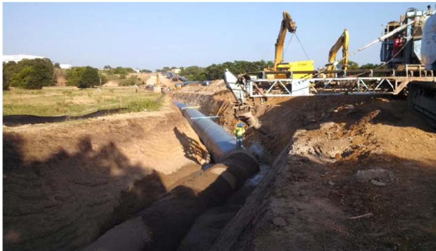
Figure 5-2 Construction of the water pipeline at Line J
