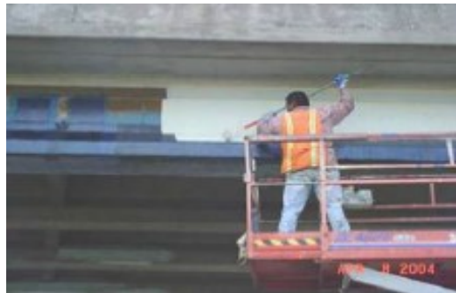
Figure 2-13 Top coat application (Image Courtesy: TXDOT)
