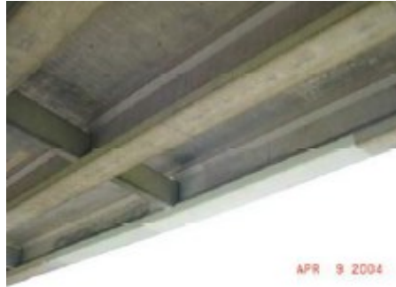
Figure 2-14 Completed CFRP repair (Image Courtesy: TXDOT)
