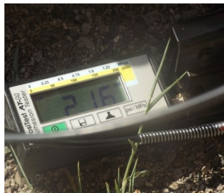
Figure 4-11 Failure stress observed after pull off test
