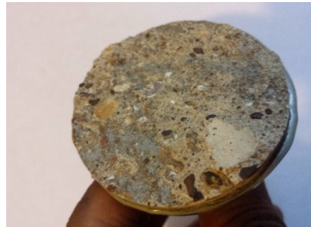
(b) Failure Mode G in sample 2
