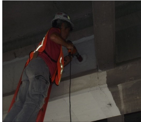
Figure 5-7 Core drilling on girder 4 (sample 1), Bridge 2
