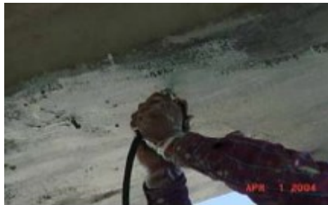
Figure 2-8 Epoxy injection in to the cracks (Image Courtesy: TXDOT)
