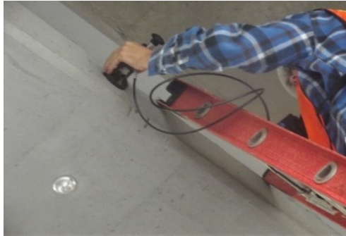
Figure 5-17 Pull-Off test on (sample 1), girder 3, Bridge 4
