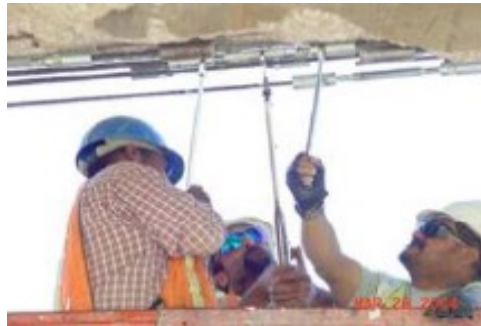
Figure 2-4 Tensioning of spliced strands (Image Courtesy: TXDOT)
