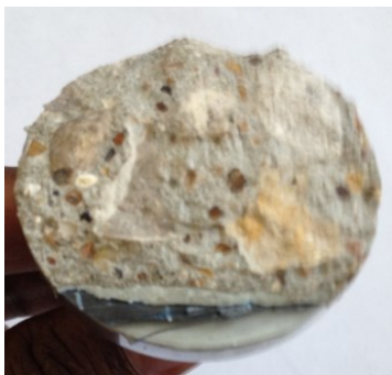
(a) Failure Mode G in sample 1
