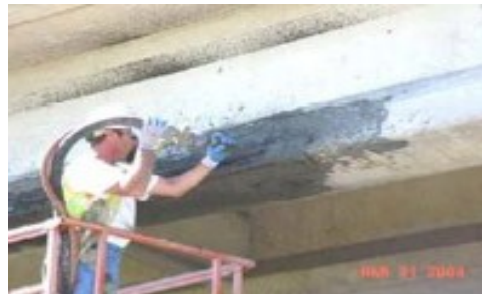
Figure 2-7 Shotcreting (Image Courtesy: TXDOT)
