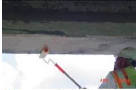
Figure 2-9 Application of primer (Image Courtesy: TXDOT)
