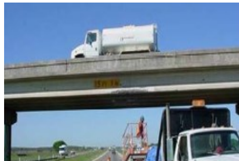
Figure 2-5 Preloading of the beam before repair (Image Courtesy: TXDOT)
