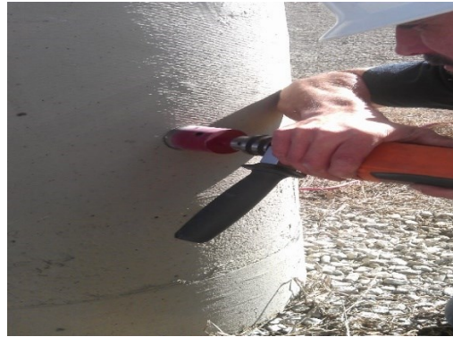
Figure 5-29 Core drilling (sample 3) in column 1, Bridge 7
