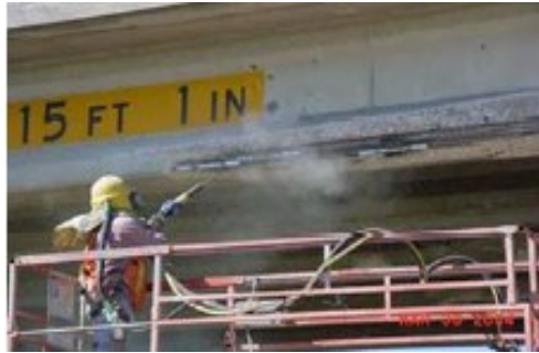
Figure 2-6 Sandblasting to clean the repair areas (Image Courtesy: TXDOT)
