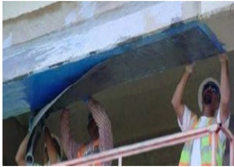
Figure 2-11 First Layer of FRP application (Image Courtesy: TXDOT)
