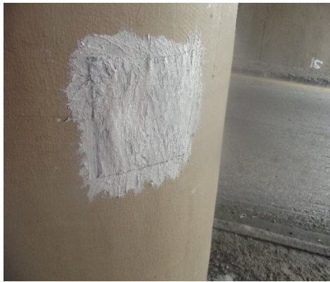
Figure 4-13 Repaired sections after Pull- Off test
