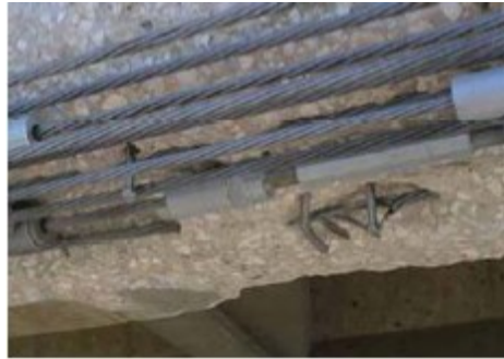
Figure 2-3 Installed steel pins in repair areas (Image Courtesy: TXDOT)
