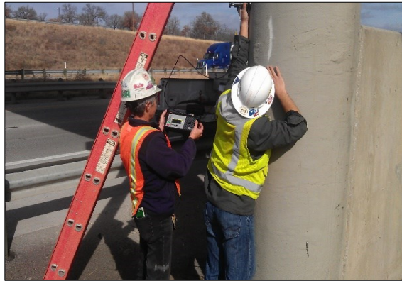
Figure 5-30 Pull-Off test on sample 1 in column 1, Bridge 7
