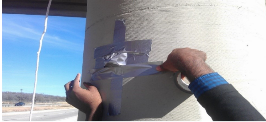
Figure 4-8 Glue tape attached to hold the dolly in place
