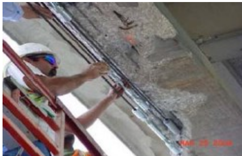
Figure 2-2 Splicing of prestressed strands (Image Courtesy: TXDOT)
