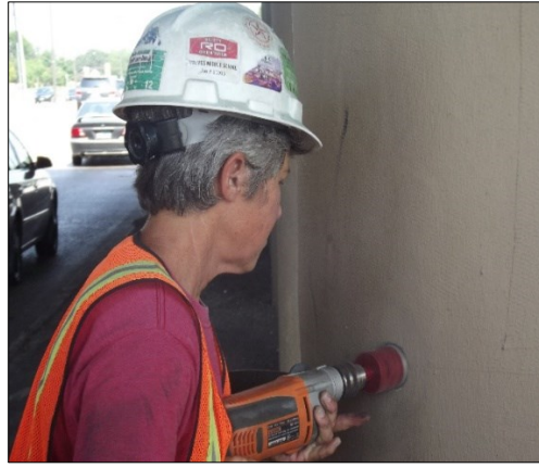
Figure 5-12 Core drilling (sample 1) in column 1, Bridge 3
