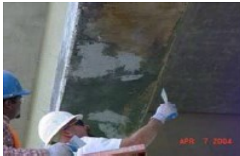
Figure 2-10 Application of epoxy (Image Courtesy: TXDOT)
