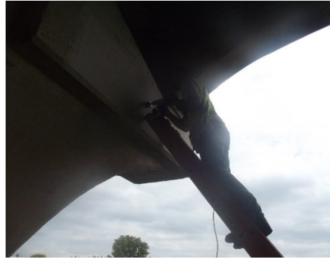
Figure 5-20 Core drilling on pier cap (sample 1), Bridge 5
