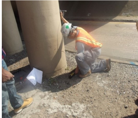
Figure 4-10 Performing pull off test on a loading fixture
