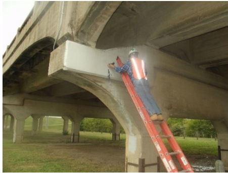
Figure 5-21 Pull-Off test on pier cap (sample 1), Bridge 5
