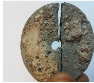
(c) Failure of core in sample 3
