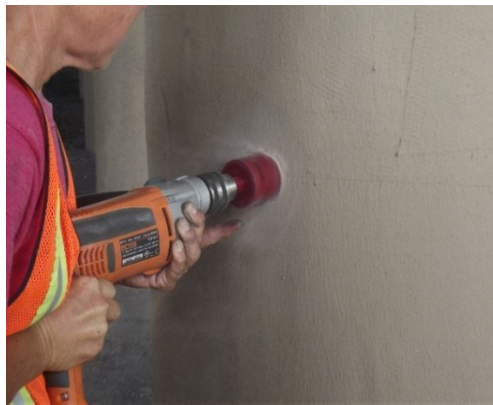
Figure 4-2 Core drilling using diamond core drill
