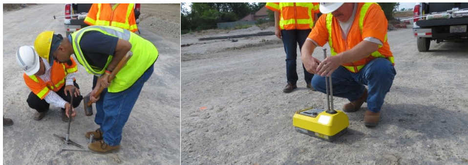
Figure 3.13: Nuclear Density Gauge Test Photos
