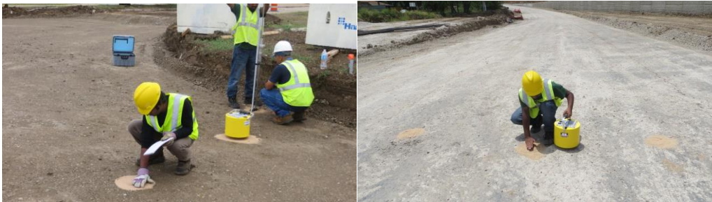
Figure 3.12: Geogauge Test Photos
