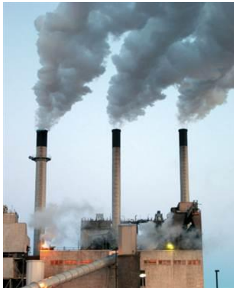
Figure 1-4 coal burning power plant (USGS)
