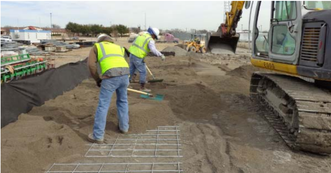
Figure 3-8 Backfill placement
