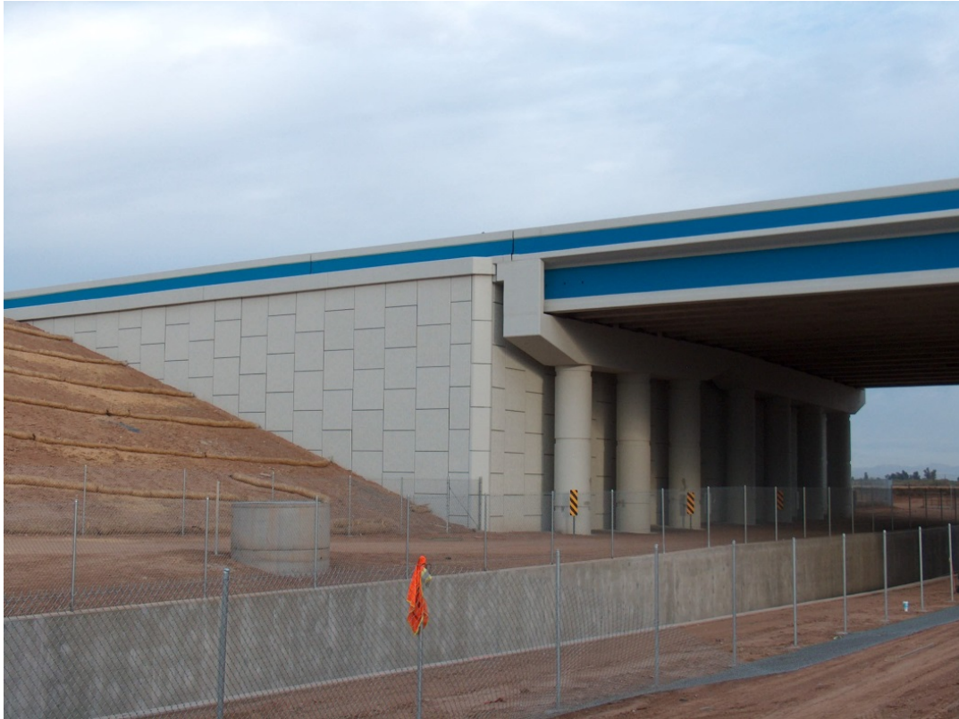
Figure 2-19 Completed 2-Stage MSE structure
