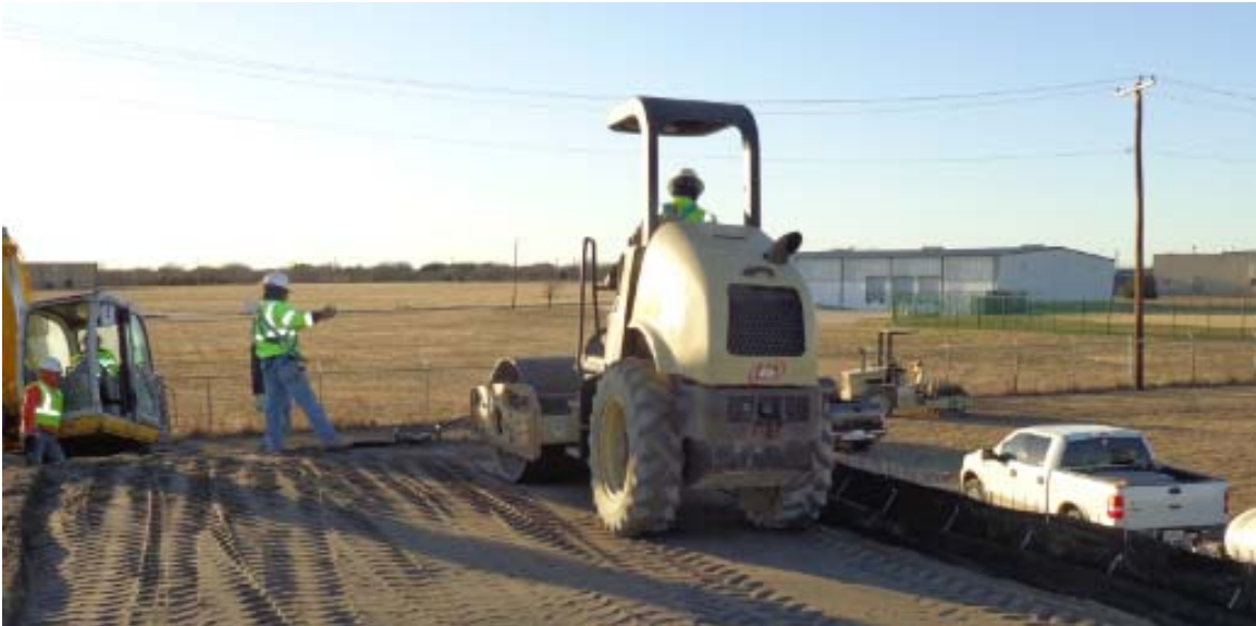
Figure 3-10 Sand backfill compaction – smooth drum rolling
