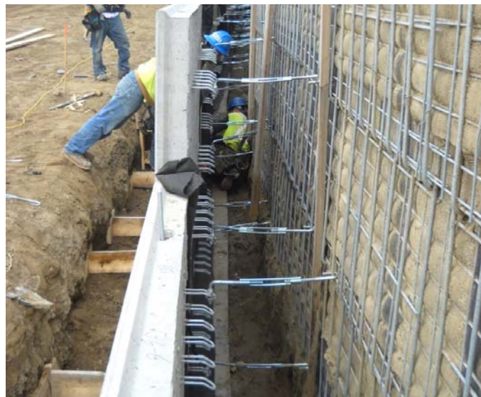
Figure 2-16 Stage-2 horizontal connection elements
