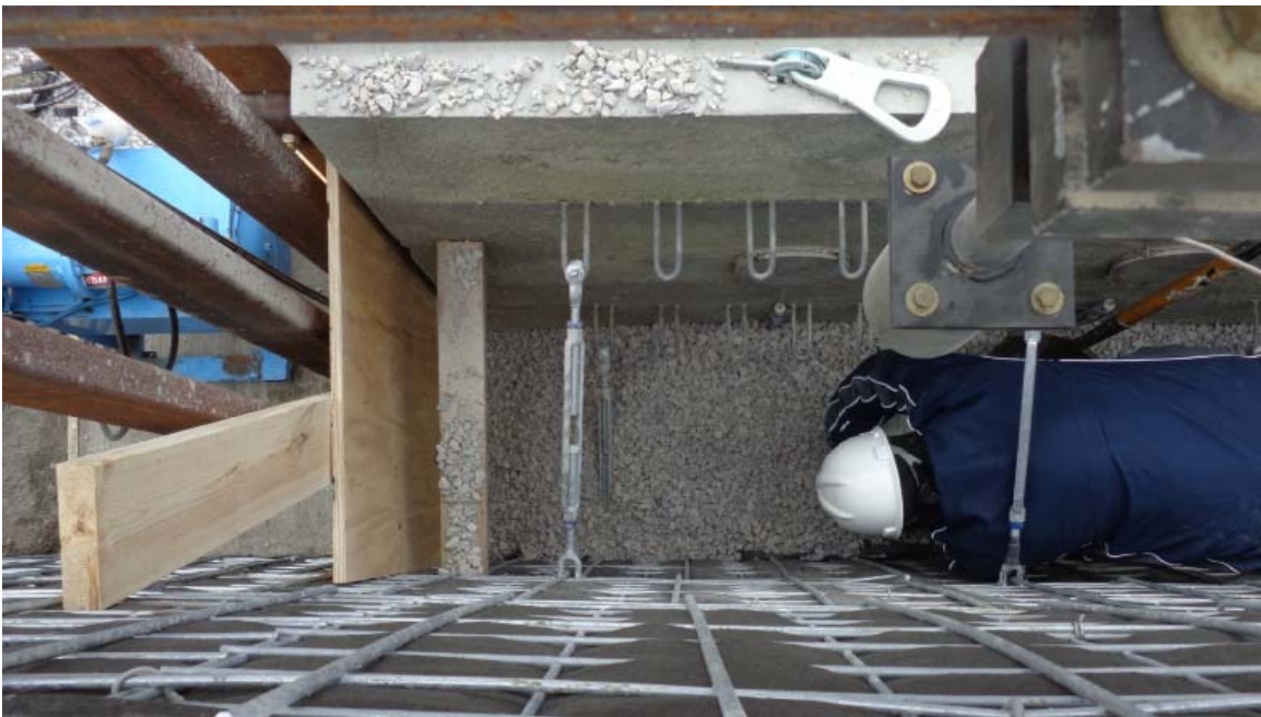
Figure 3-23 Placement of cavity fill
