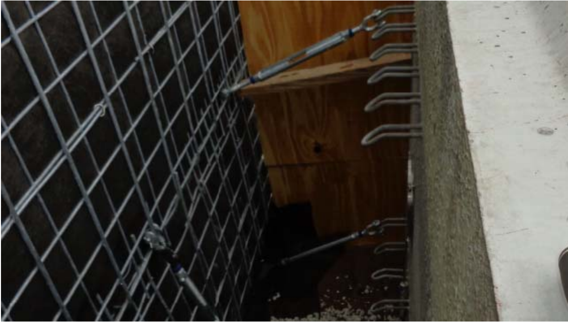
Figure 3-22 Turnbuckle attached to Stage-1 and Stage-2
