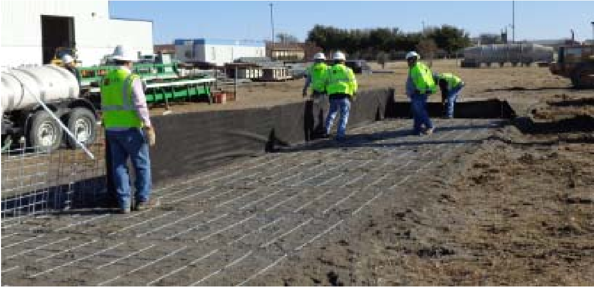
Figure 3-7 Facing geotextile placement
