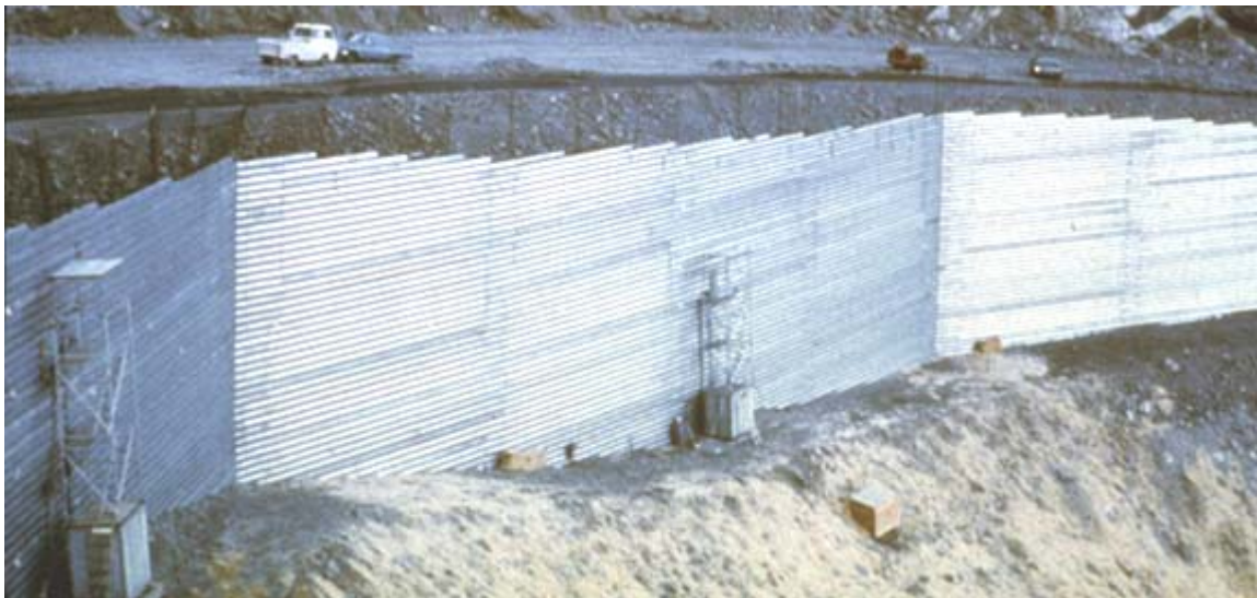
Figure 1-2 First reinforced earth wall constructed in United States (NCHRP 1987)
