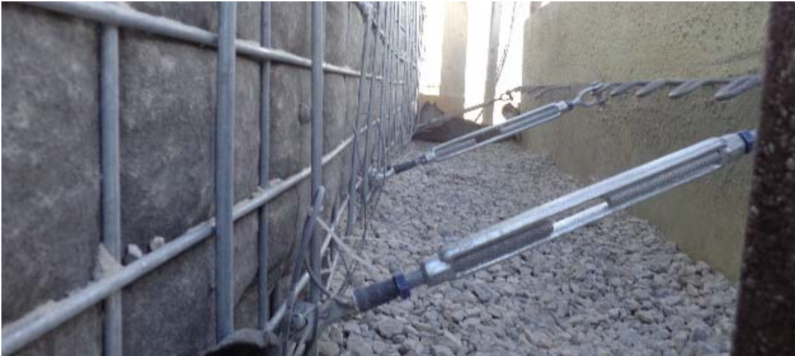
Figure 3-24 Top turnbuckle and cavity fill
