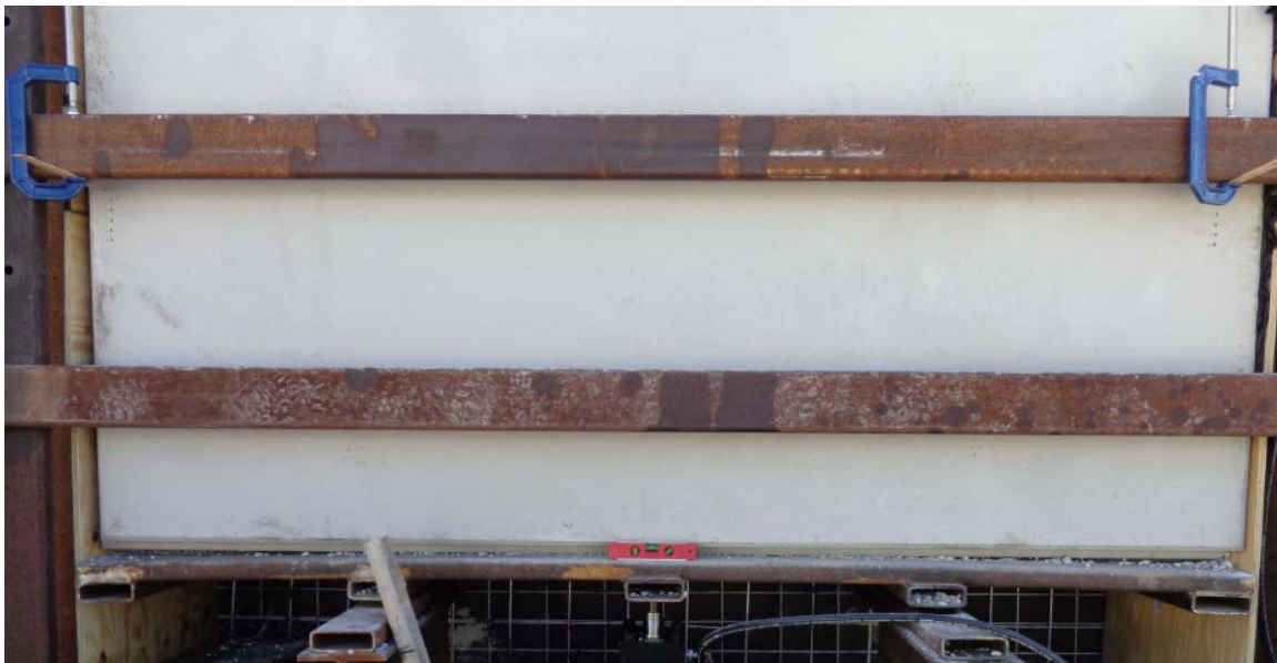
Figure 3-21 Placement of SCP with safety beams
