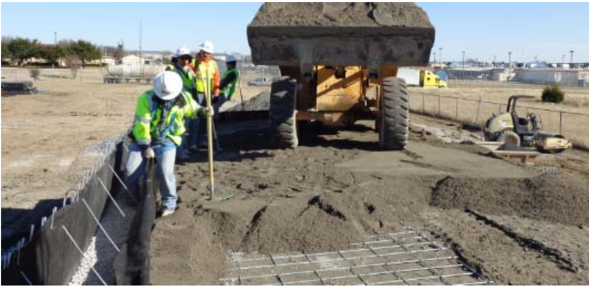
Figure 3-12 Interface geotextile separation
