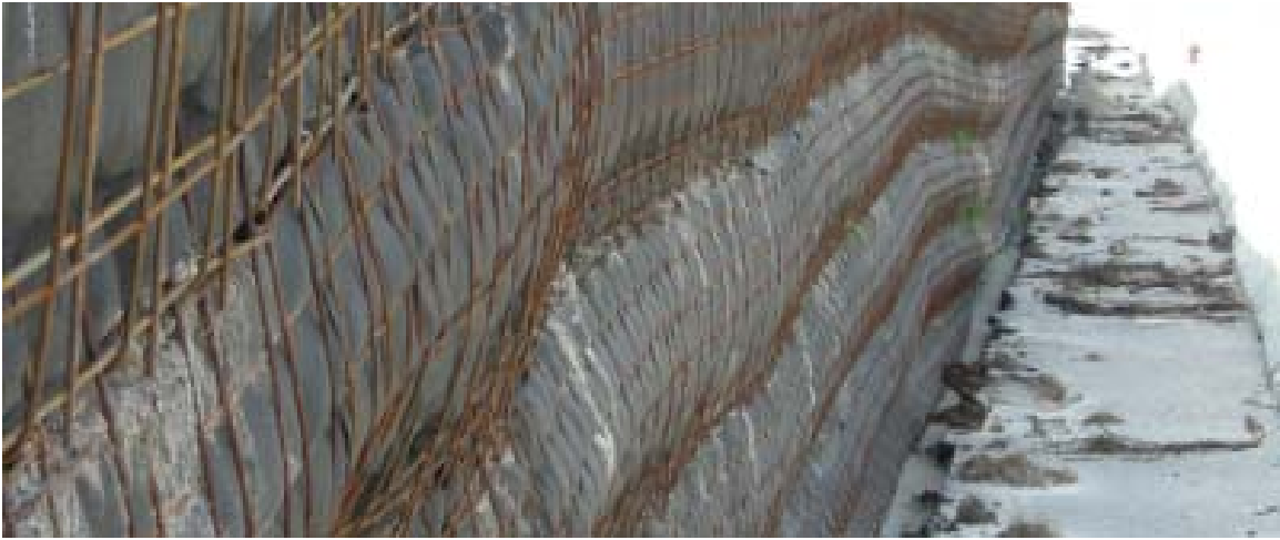
Figure 4-3 Stage-1 bulging at face of welded wire wall
