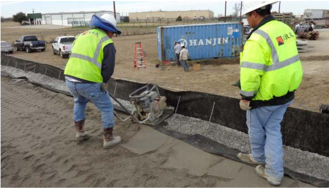
Figure 3-13 Facing rock compaction – plate compactor
