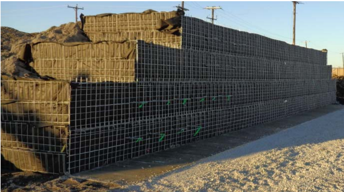
Figure 3-14 Finished Stage-1 MSE wall
