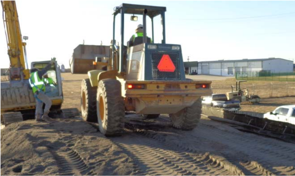
Figure 3-9 Sand backfill compaction – wheel rolling
