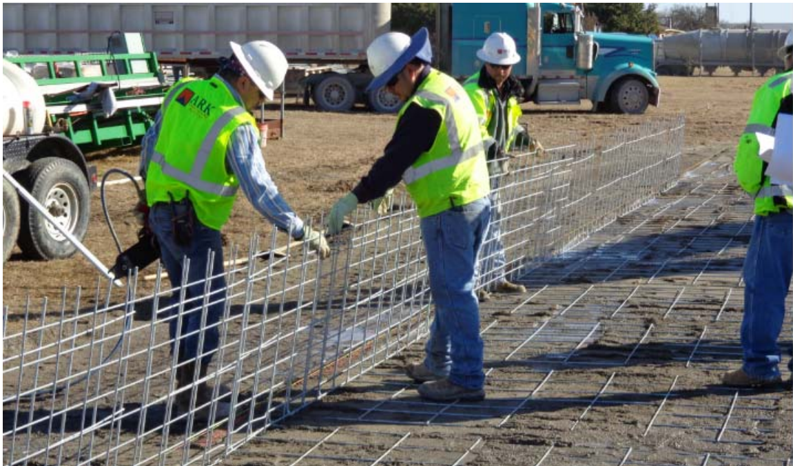
Figure 3-6 Stage-1 MSE wall construction
