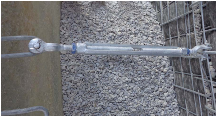
Figure 3-20 Jaw- & Jaw Turnbuckle attached to 2-Stage structure
