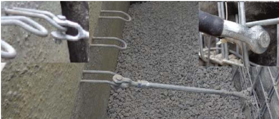
Figure 4-5 Jaw & Jaw turnbuckle installed in field
