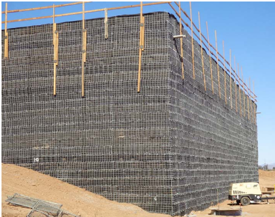
Figure 2-15 Stage-1 flexible faced MSE structure
