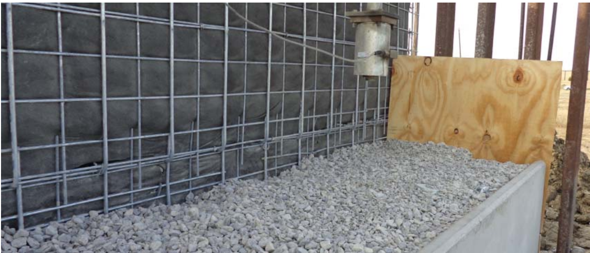
Figure 3-25 Final level of cavity fill
