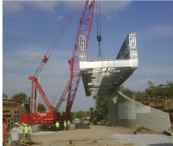
Figure 6 - Acrow Bridge Crane Pick
