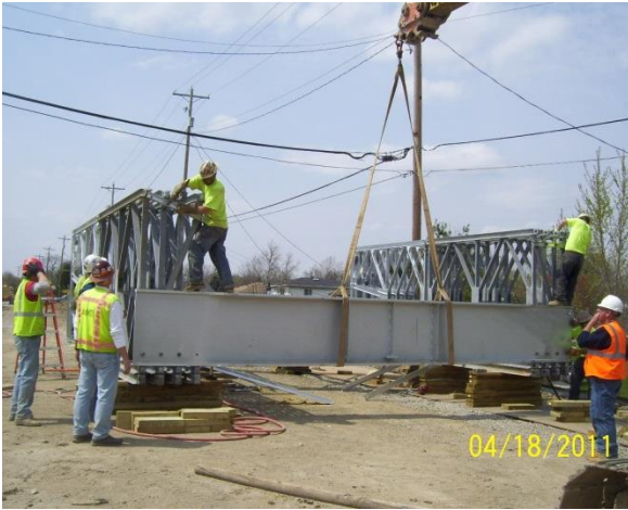
Figure 5 - Acrow Bridge Assembly
