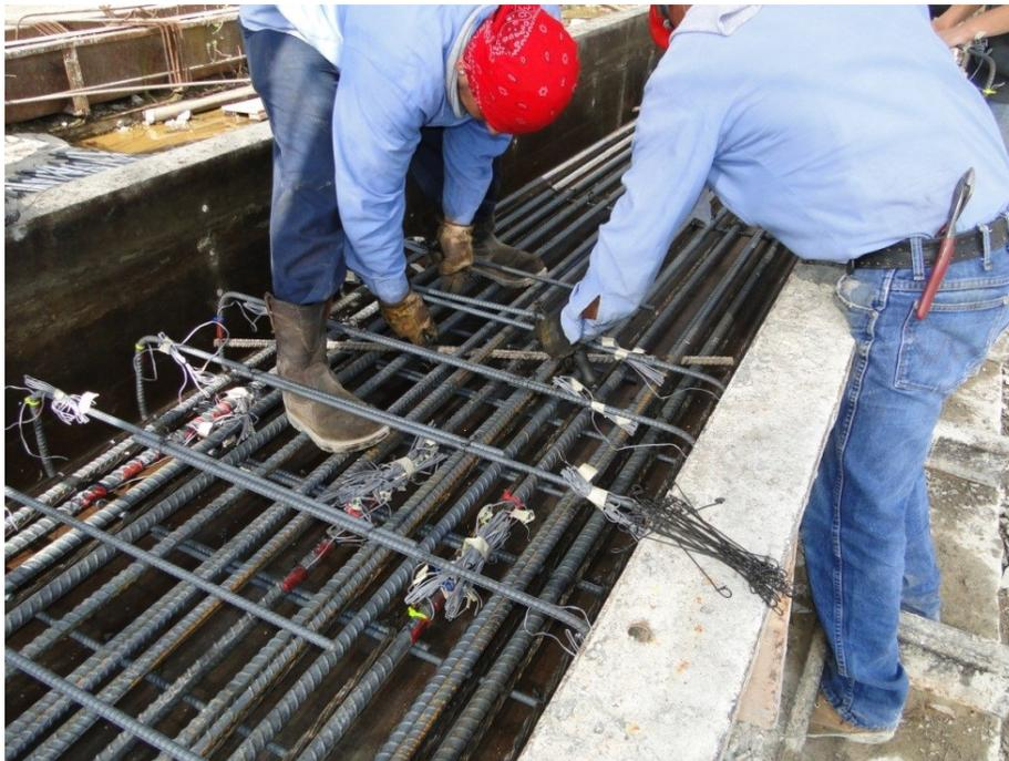
Figure 253. Placing of strain gauged stirrups
