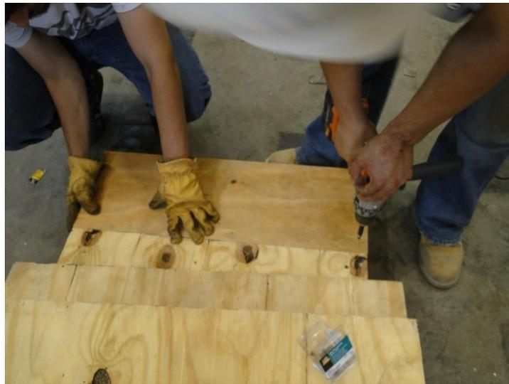
Figure 64. Drilling extension piece to modified column formwork
