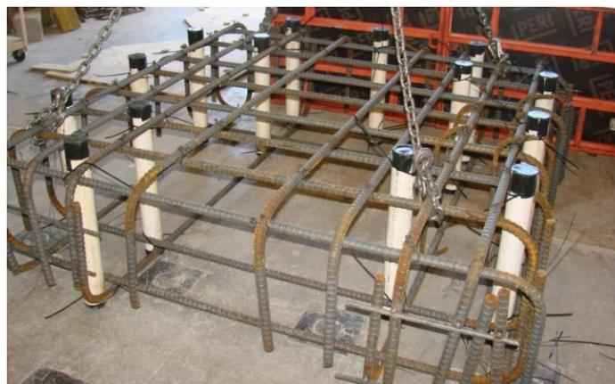
Figure 58. Loading block cage and formwork
