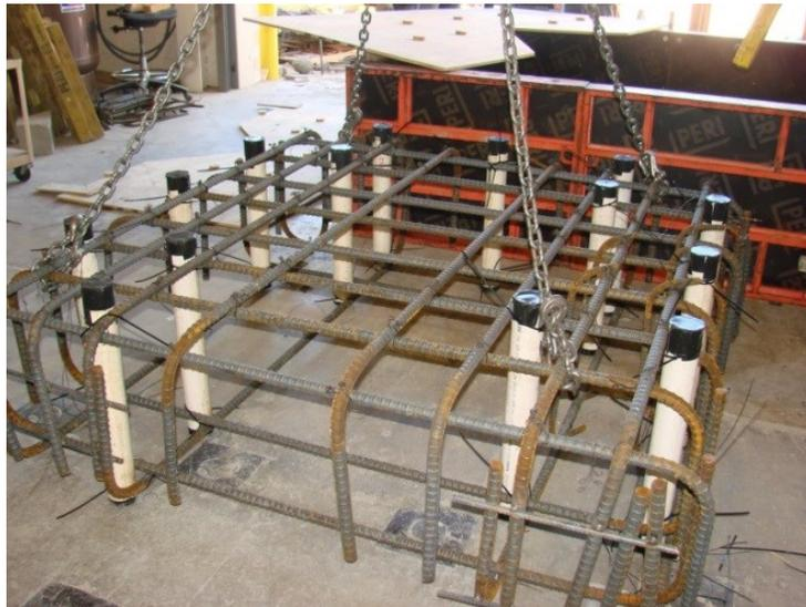
Figure 165. Loading Block Cage and Formwork
