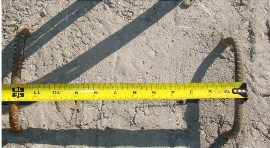
Figure 167. Spacing of horizontal shear reinforcement
