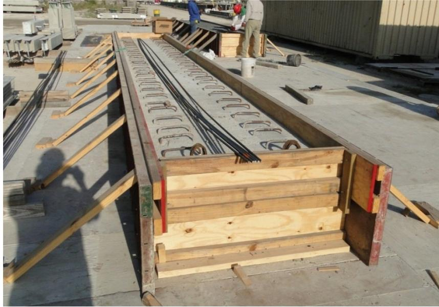
Figure 268. Slab beam and CIP formwork
