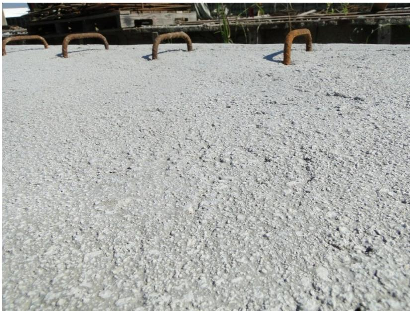
Figure 296. Surface finish on slab beam having conventional concrete
