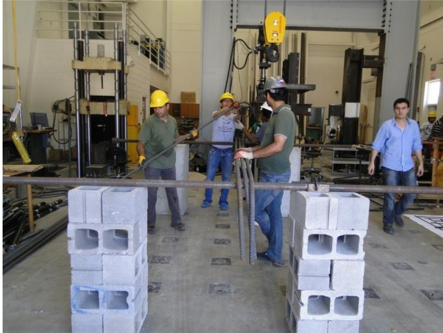
Figure 36. Placement of top layer of longitudinal bars
