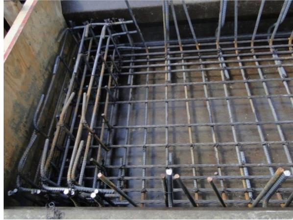
Figure 239. End mat reinforcement
