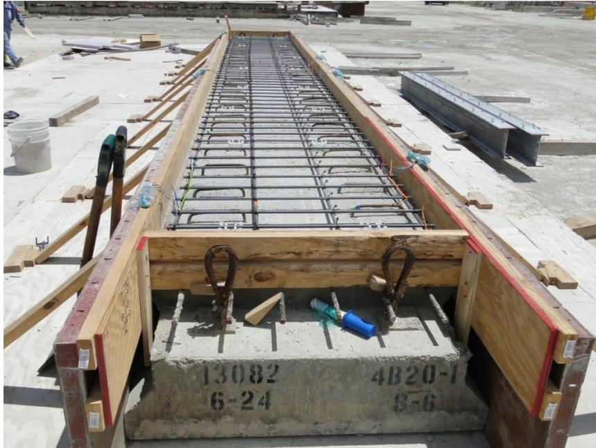
Figure 270. Box beam with CIP reinforcement
