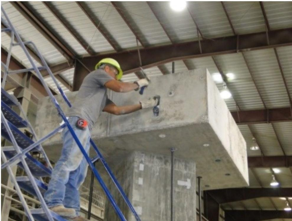
Figure 143. Placing chokers for lifting
