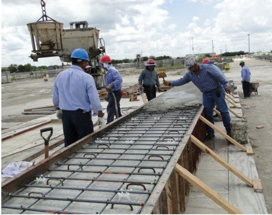
Figure 276. CIP casting
