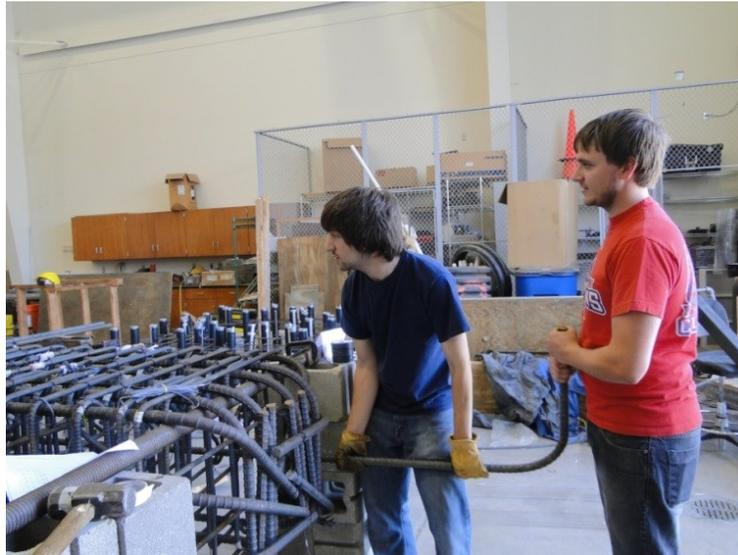
Figure 49. Inserting the side longitudinal reinforcement
