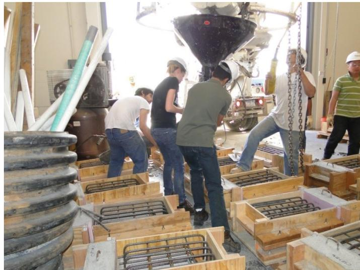
Figure 215. CIP caging and formwork
