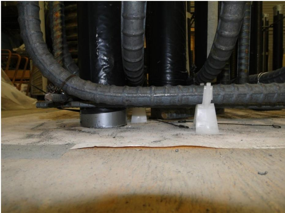
Figure 28. Chairs underneath bottom block for 1 ½ inch cover
