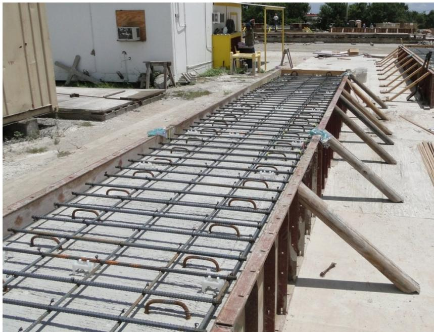
Figure 271. Slab beam with CIP reinforcement
