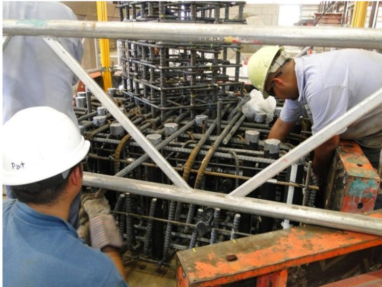
Figure 71. Placement of bottom block reinforcement through column cage
