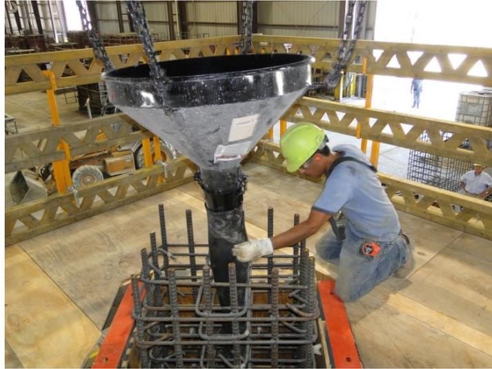
Figure 114. Placement of funnel
