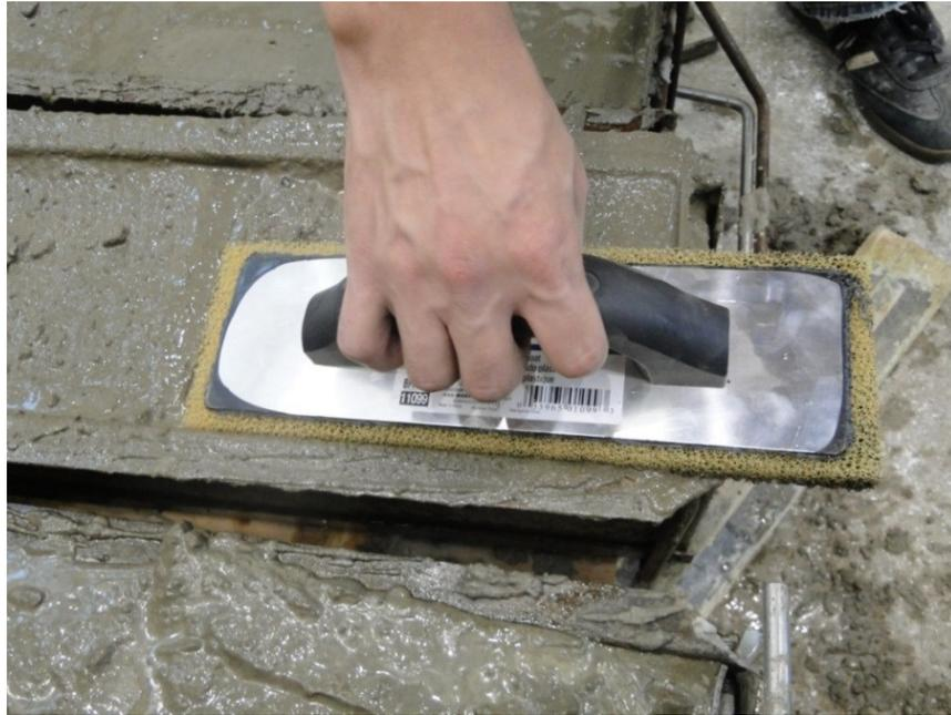
Figure 201. Surface preparation using a sponge float
