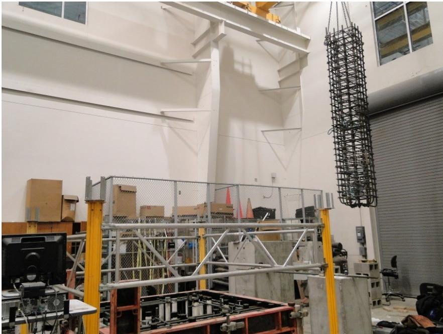
Figure 160. Placing of the Column Cage into the Footing Block
