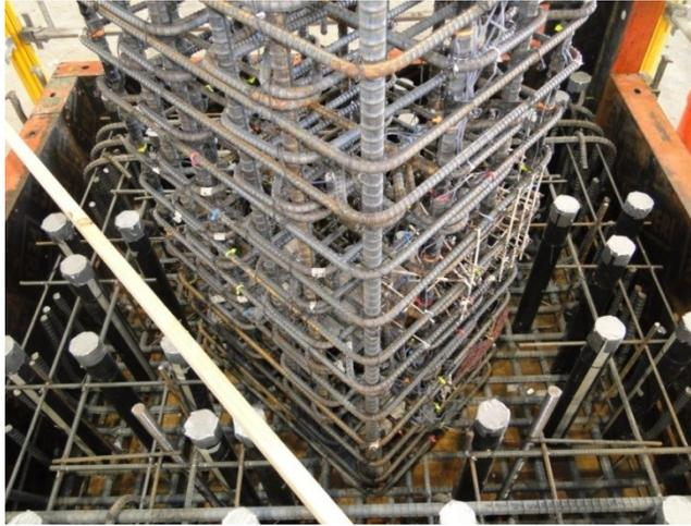
Figure 70. Placing the column cage at 45°
