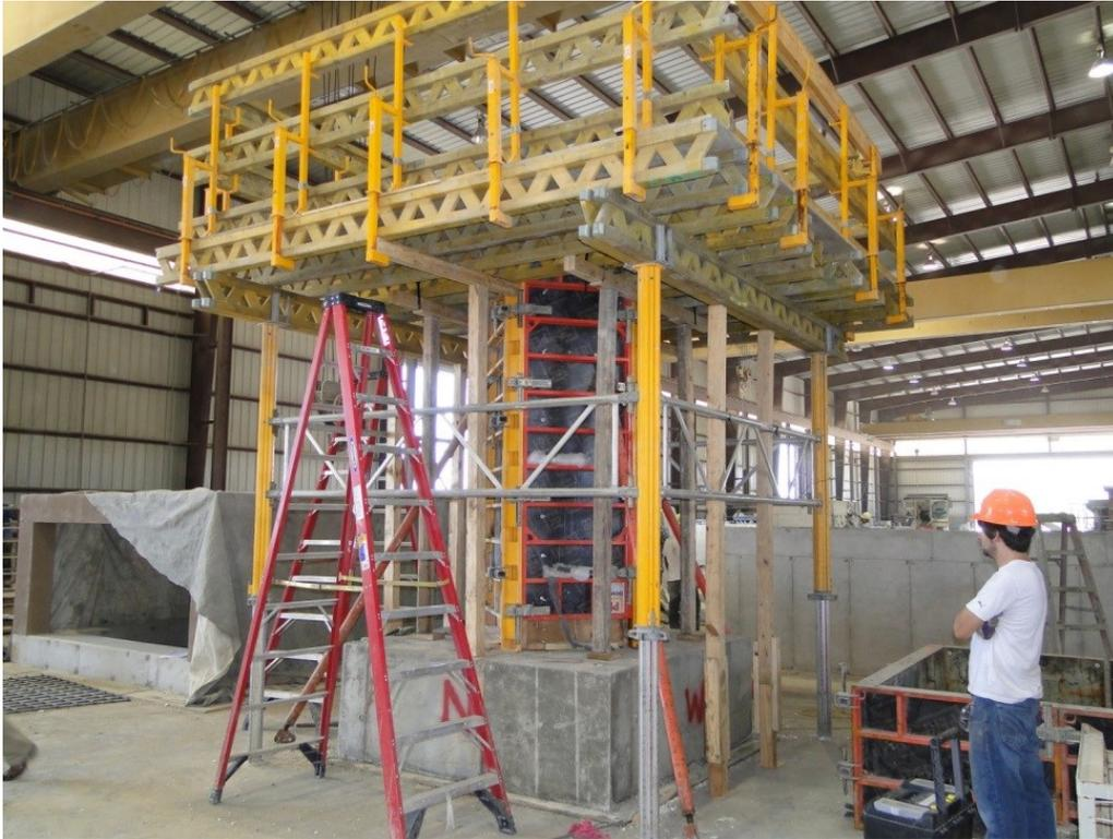
Figure 120. Removal of bottom block formwork
