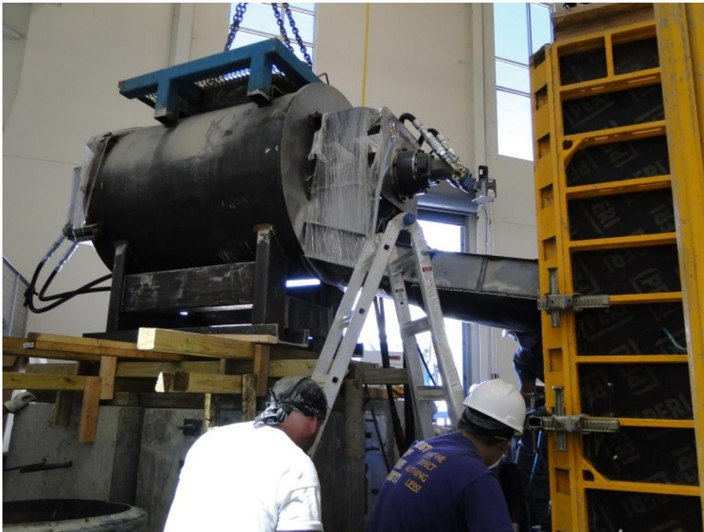
Figure 179. Elevated Mixer ready for pouring
