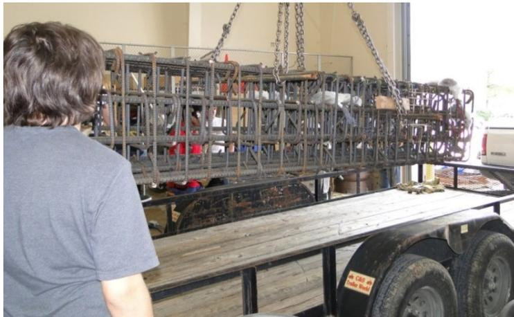
Figure 67. Shipping of column cage
