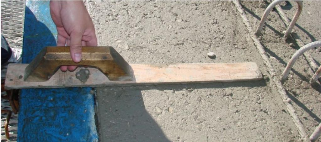
Figure 169. Application of wood float finish
