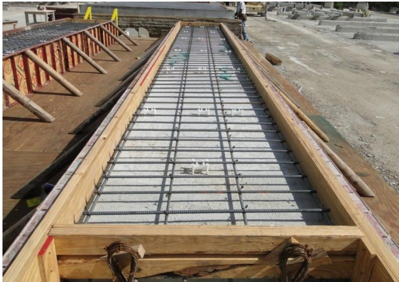
Figure 272. Slab beam without shear reinforcement and CIP reinforcement
