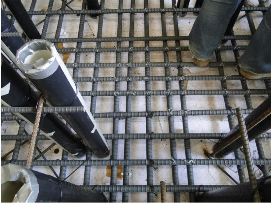
Figure 27. Bottom of Cage tied in a crisscross pattern
