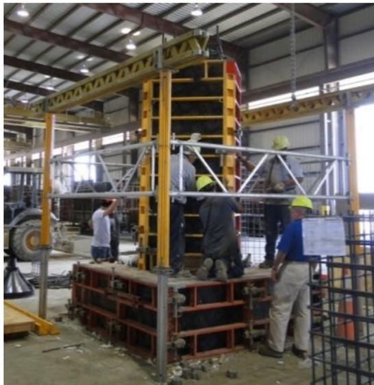
Figure 93. Placing of second formwork panel
