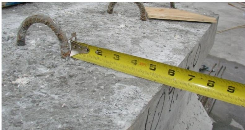
Figure 173. Horizontal shear reinforcement details
