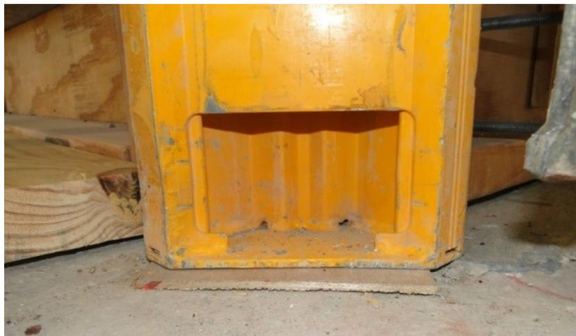
Figure 107. Inserting small wooden pieces to prevent leaking
