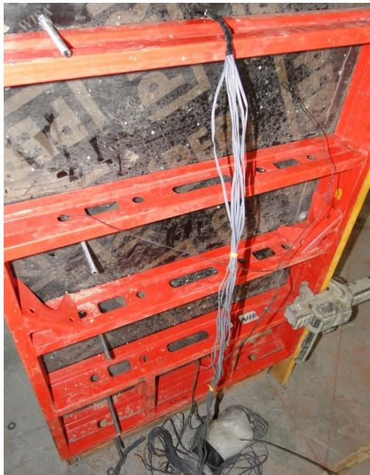
Figure 97. Passing strain gauge wires through the column panel
