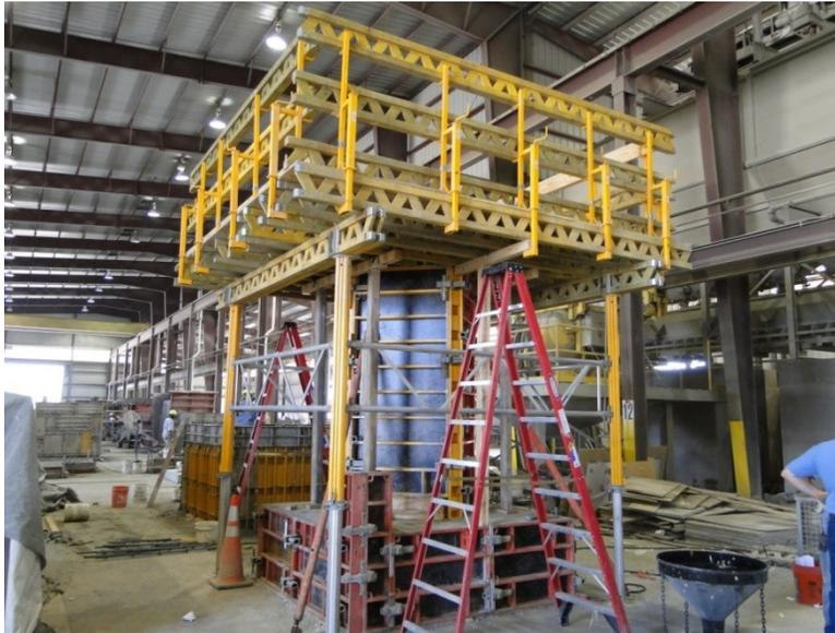
Figure 108. Placement of deck railing
