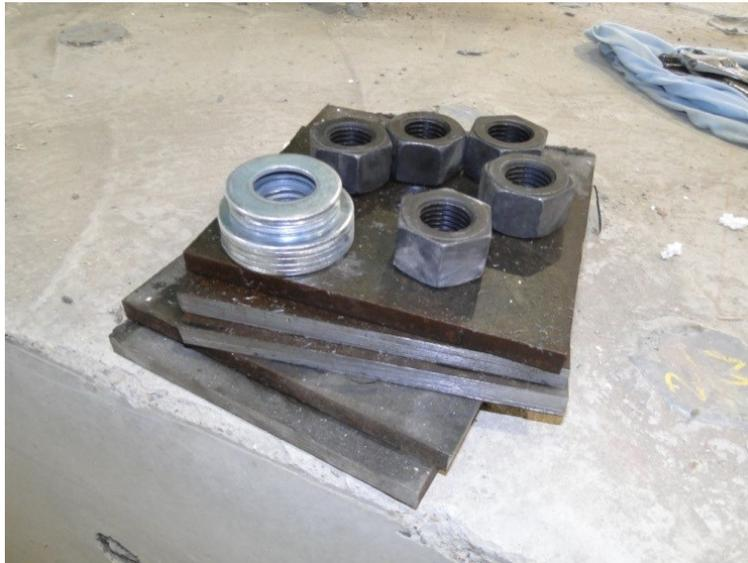
Figure 139. Post tensioning plates, nuts and washers
