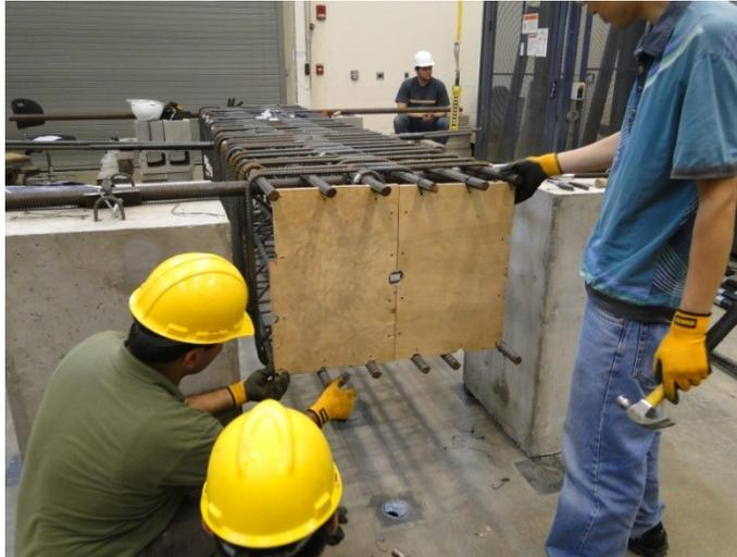
Figure 44. Two halves of template at the top of the column cage
