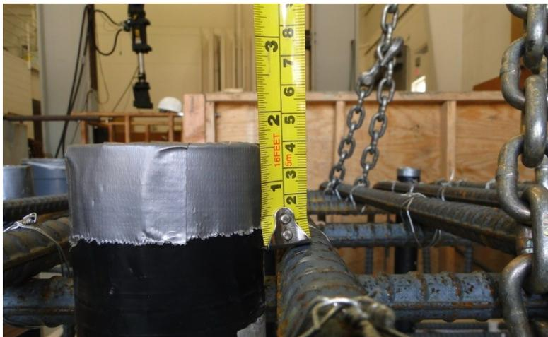
Figure 59. Checking concrete cover
