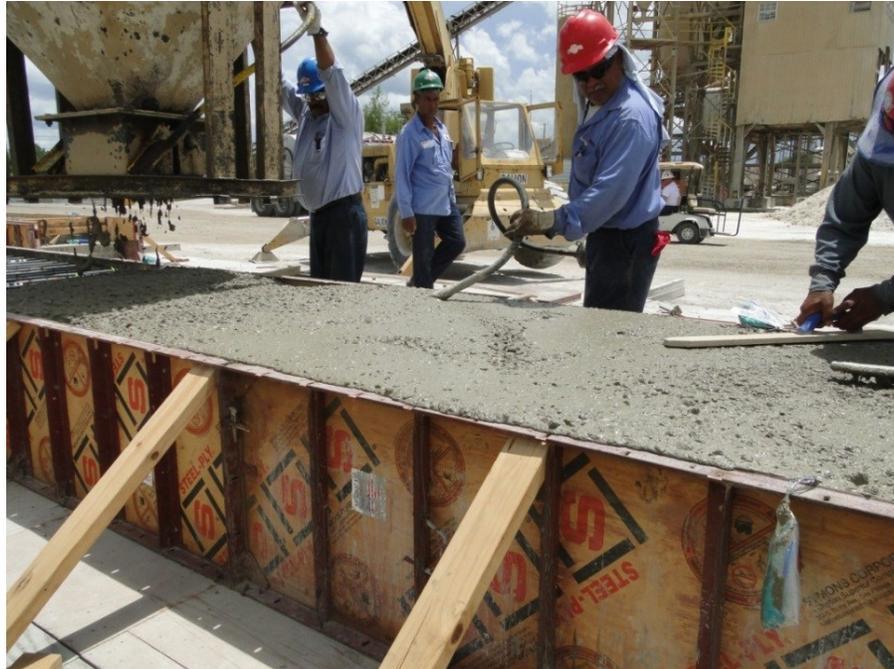
Figure 275. Vibrating and wood float finishing
