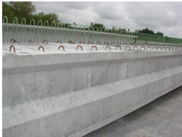
Figure 172. Finished box beam
