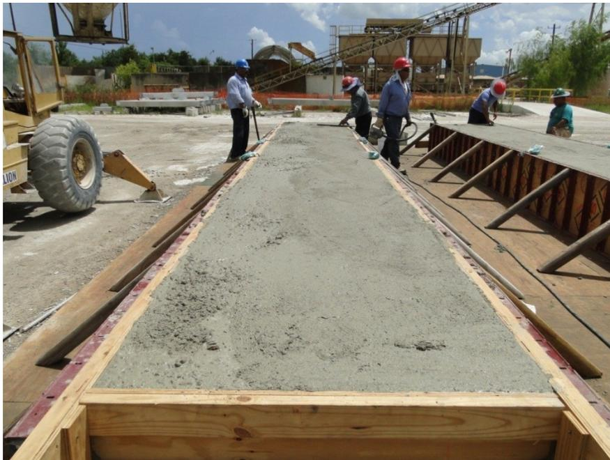
Figure 279. Finished CIP surface
