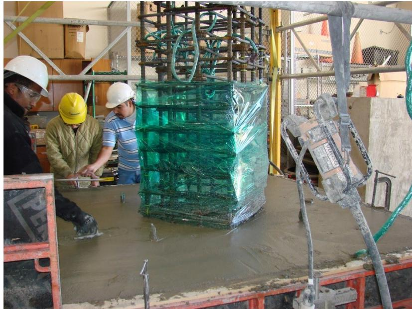
Figure 163. Finishing of bottom block surface
