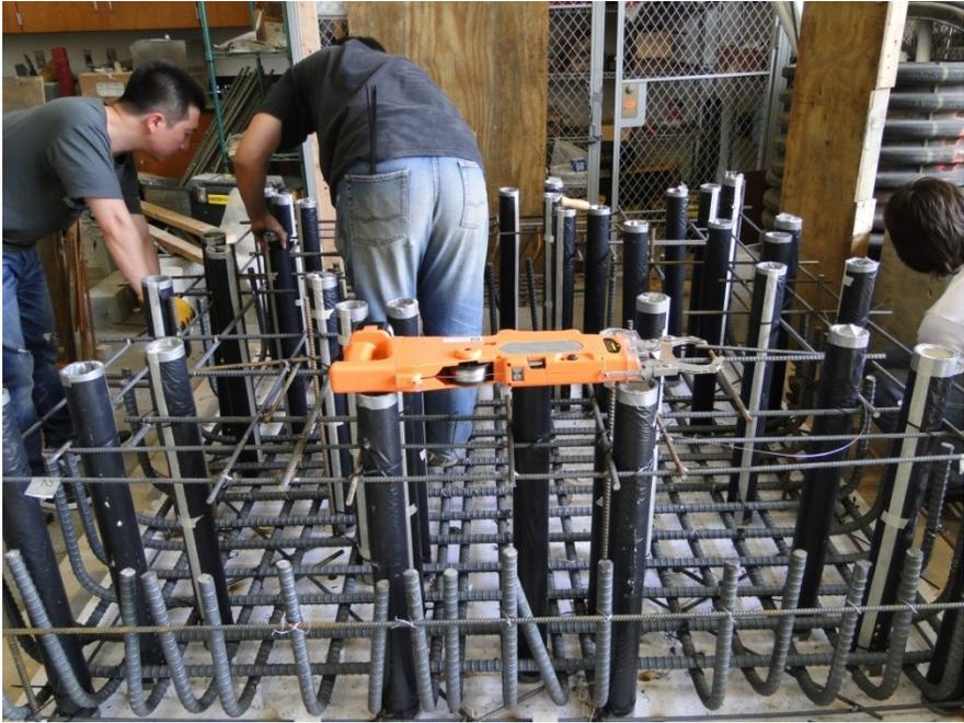
Figure 26. placement of second layer of bottom reinforcement
