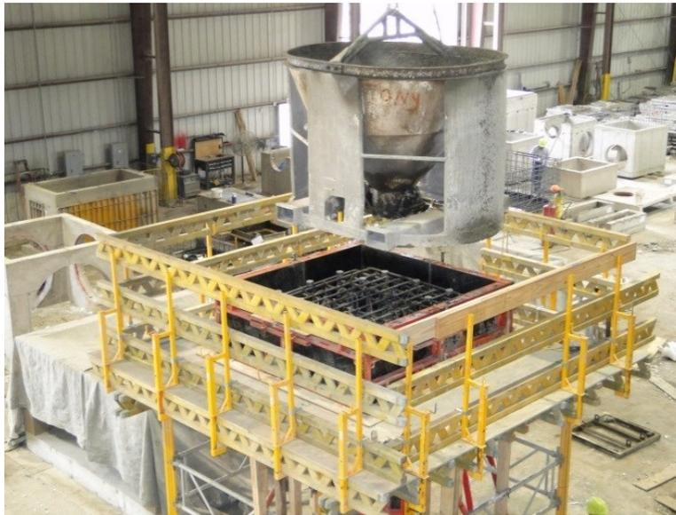
Figure 129. Lifting bucket above column
