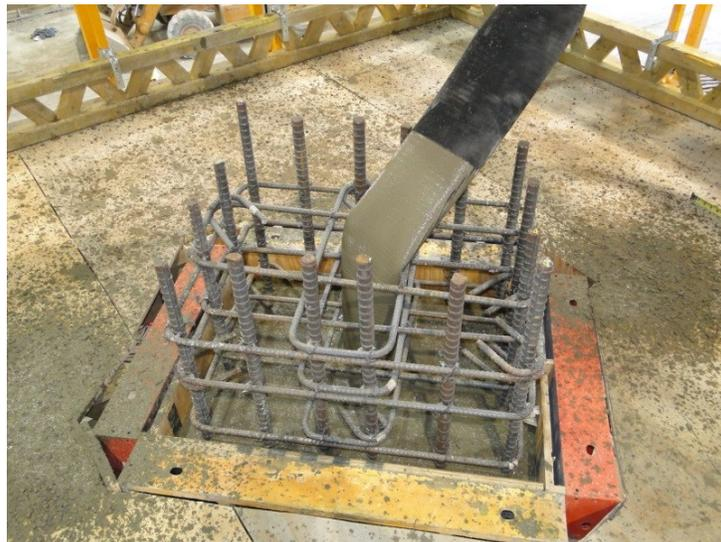
Figure 115. Column Casting
