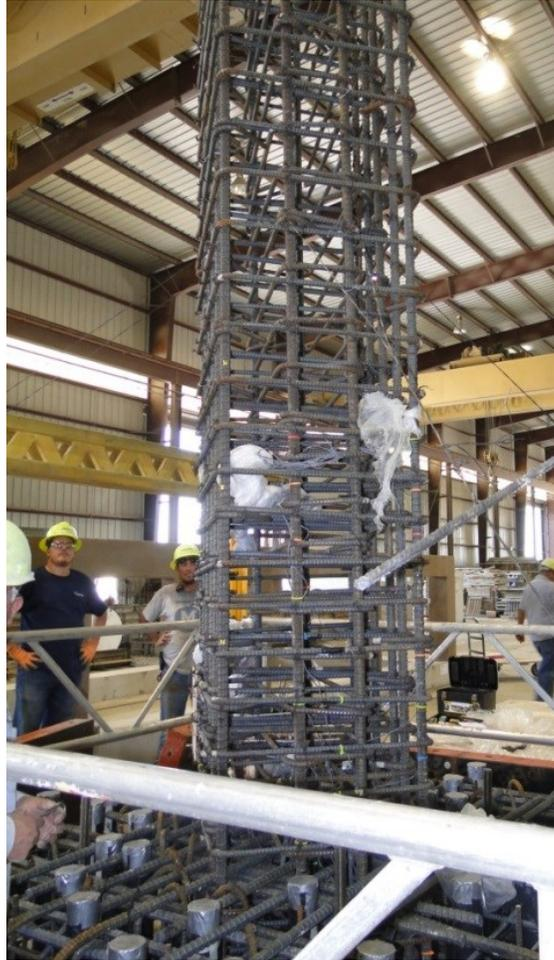
Figure 72. Leveled column cage
