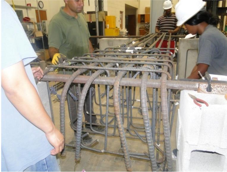
Figure 37. Placing of transverse reinforcement
