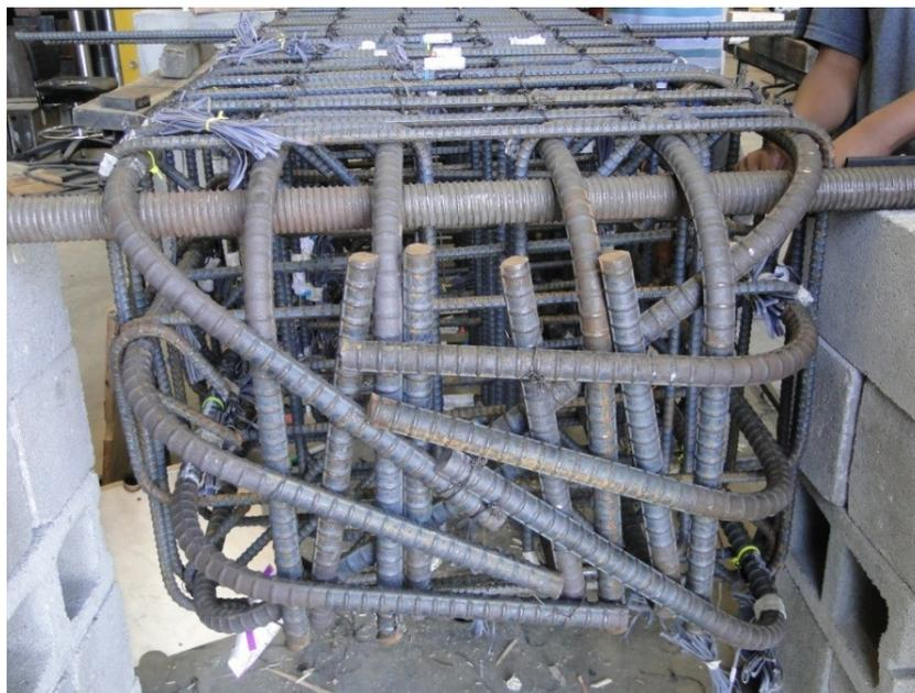
Figure 50. Tied longitudinal reinforcement at the base of the column cage
