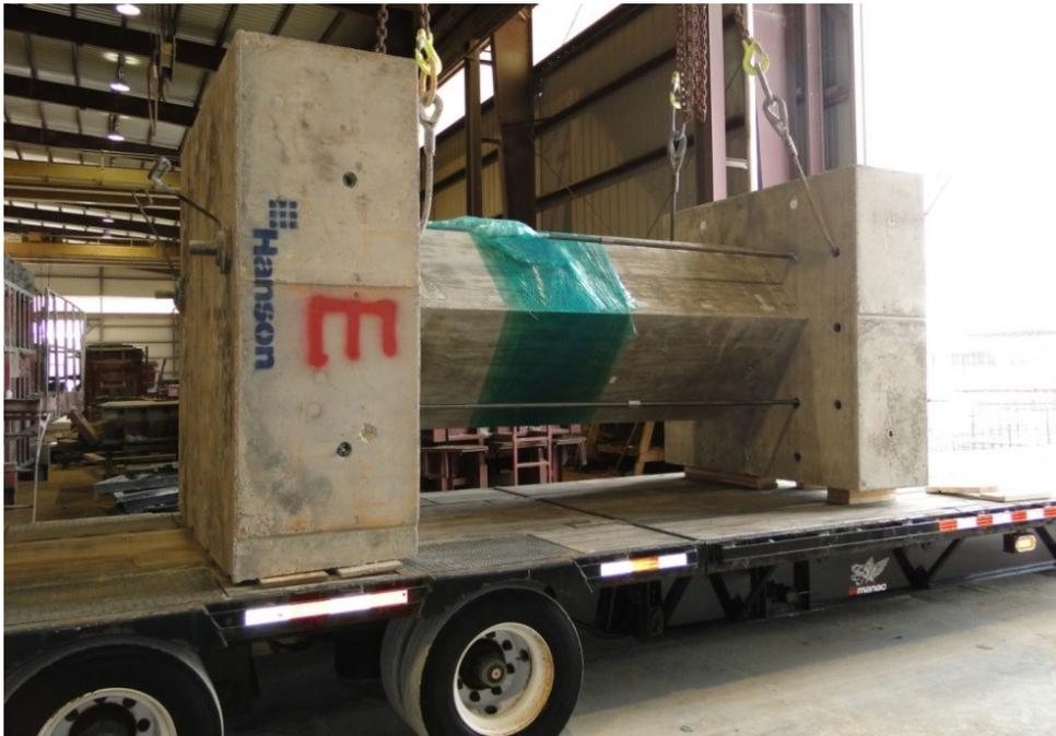
Figure 155. Setting column on flatbed truck
