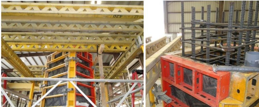
Figure 101. Column formwork construction
