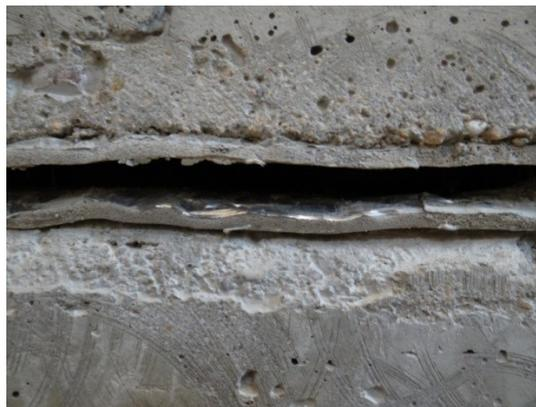
Figure 329. Separation between CIP slab and precast beam
