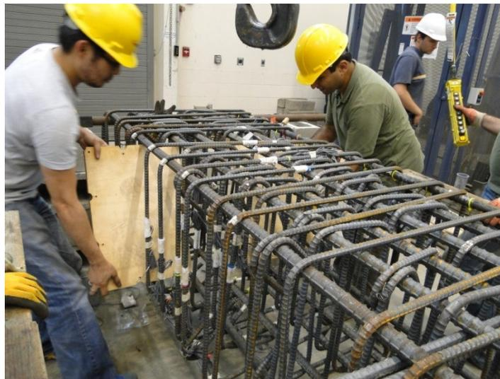
Figure 45. Template placement near the base of the column cage
