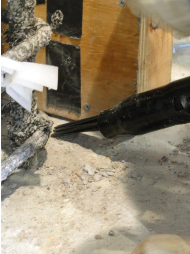
Figure 98. Chipping off top concrete layer
