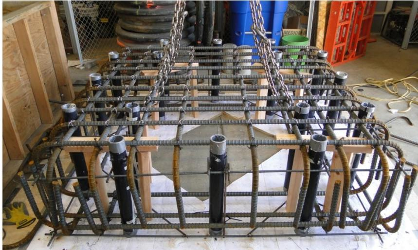
Figure 58. Placing top layer of reinforcement
