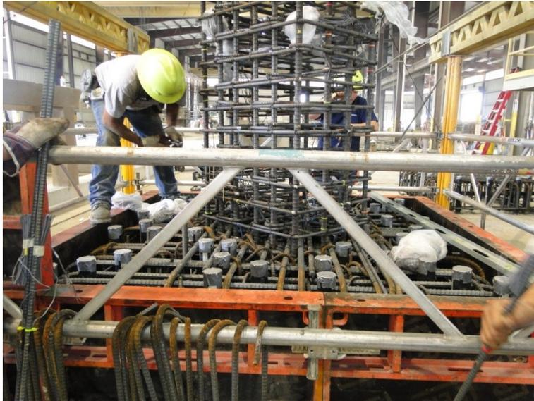
Figure 73. Placement of shear reinforcement
