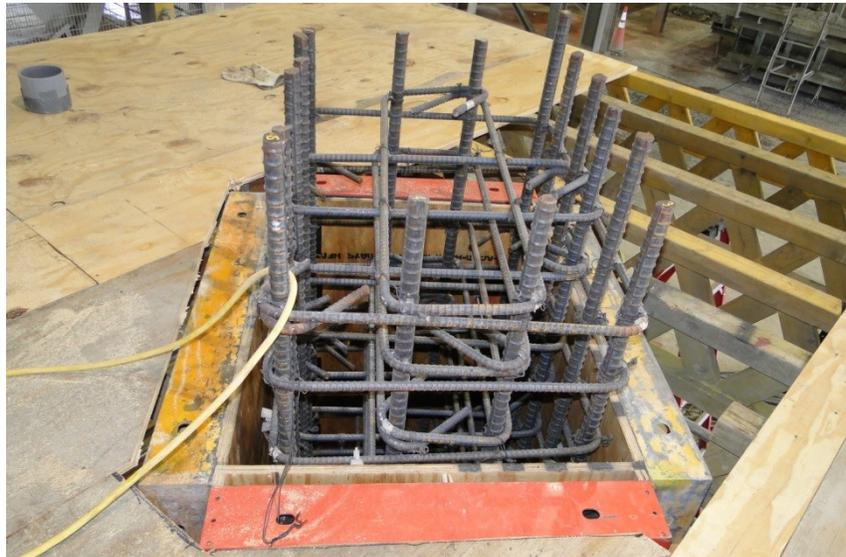
Figure 103. Raising frame flush with the top of the column formwork
