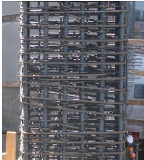
Figure 51. Typical confinement reinforcement used in normal strength columns for RC moment frames (photo courtesy of Dr. Shih-Ho Chao)
