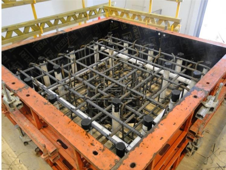
Figure 166. Top block cage and formwork
