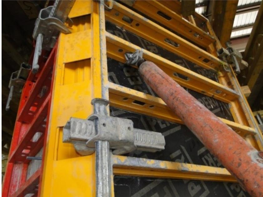
Figure 104. Attaching lateral supports
