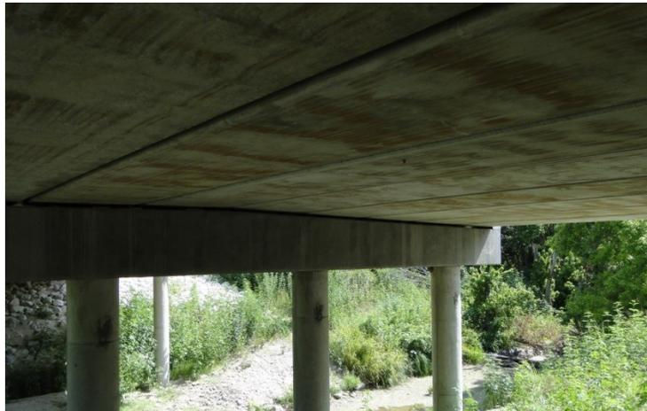
Figure 186. Girder spacing according to TxDOT practice
