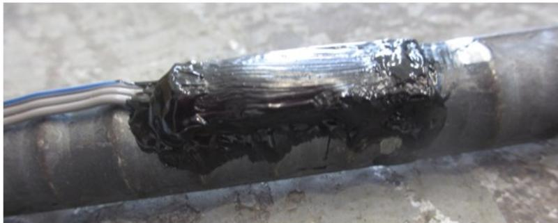
Figure 42. Liquid electrical tape application
