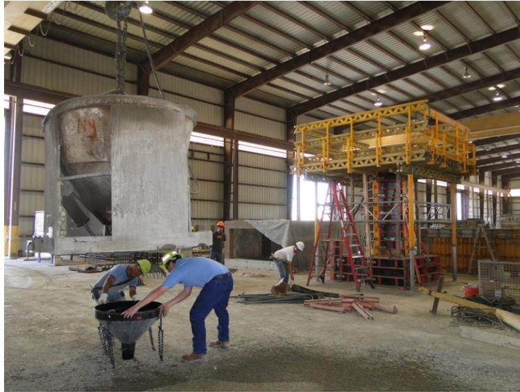
Figure 112. Attaching the funnel and “elephant trunk”
