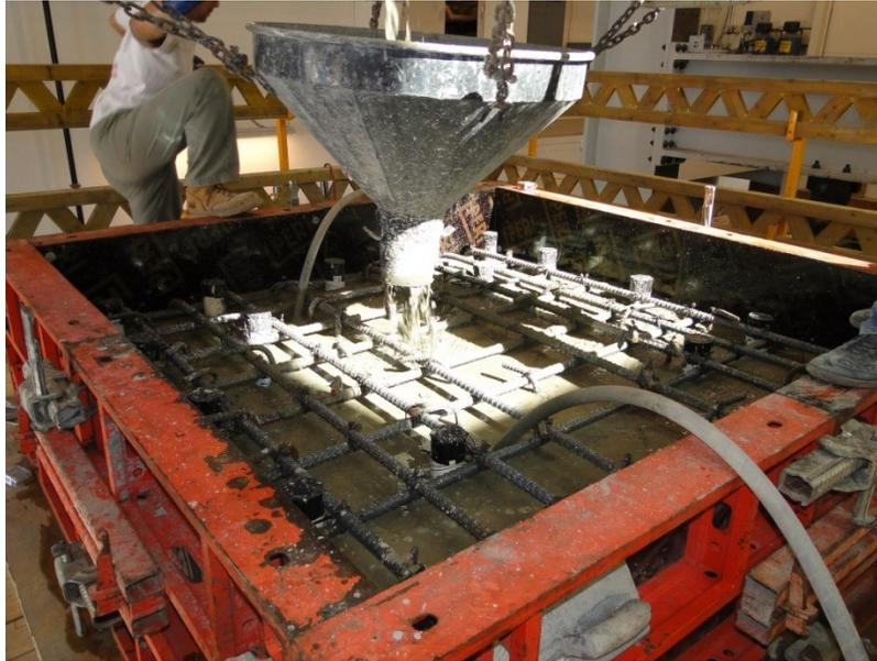
Figure 168. Casting of loading block
