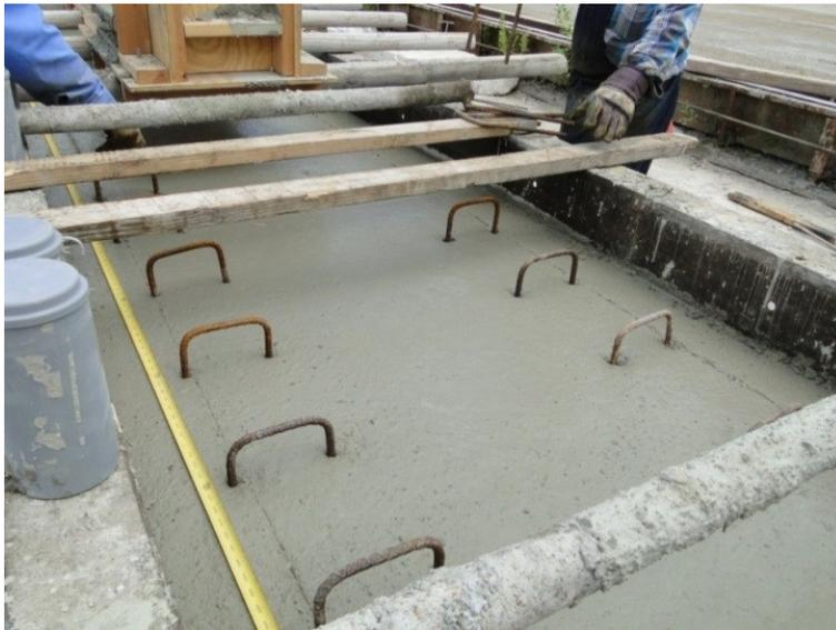
Figure 294. Placing of horizontal shear reinforcement
