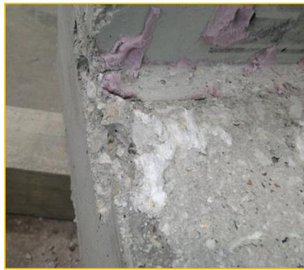
(b) Concrete fracture near interface
