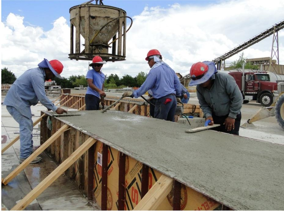
Figure 278. Finishing of CIP part of specimens
