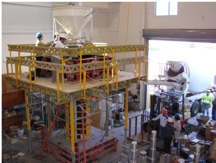
Figure 167. Final Column and Loading Block Casting
