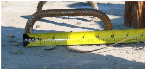
Figure 168. Horizontal shear reinforcement details
