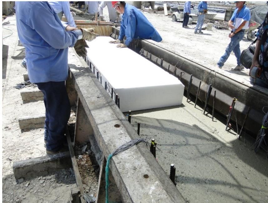
Figure 242. Placement of the Styrofoam
