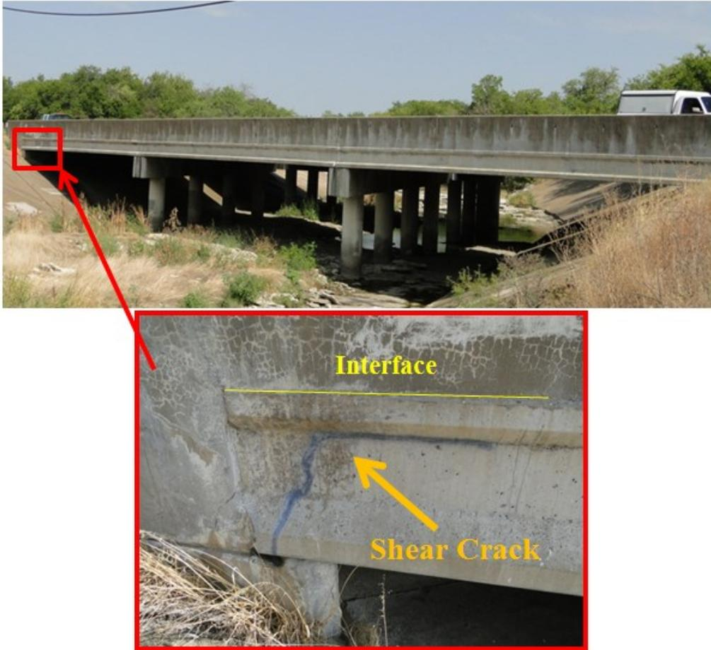
Figure 165. Shear cracks observed at the South-West end of the Long Ave. Bridge
