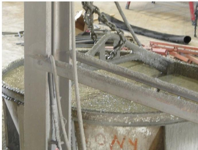
Figure 111. Pouring concrete into bucket
