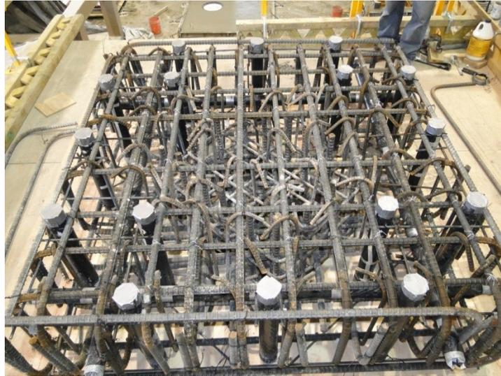
Figure 126. Placing bottom layer of top block reinforcement through column cage
