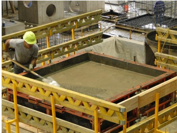
Figure 131. Finishing top block surface
