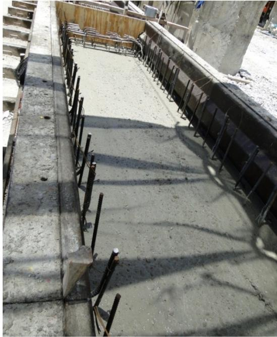
Figure 241. Concrete poured to 5 inches
