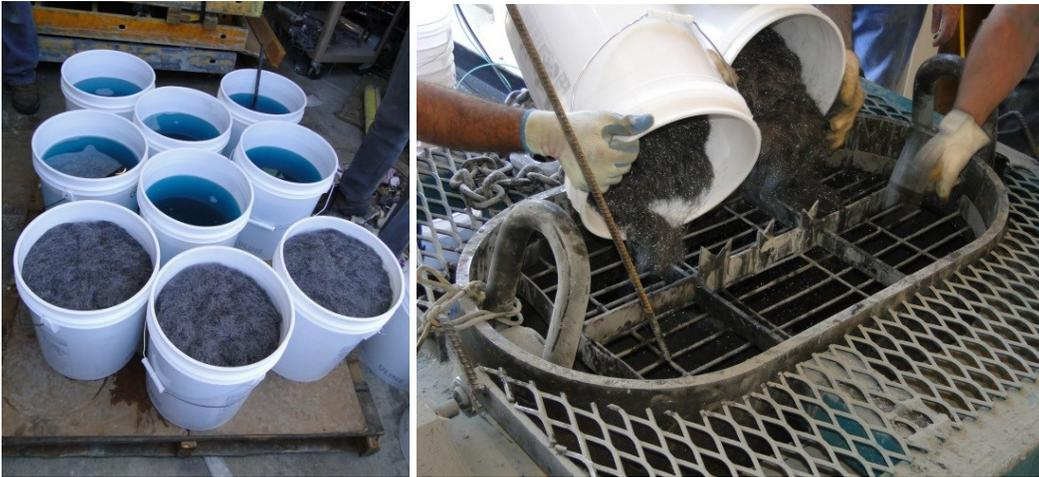
Figure 178. Addition of Micro-Fibers to Mixer
