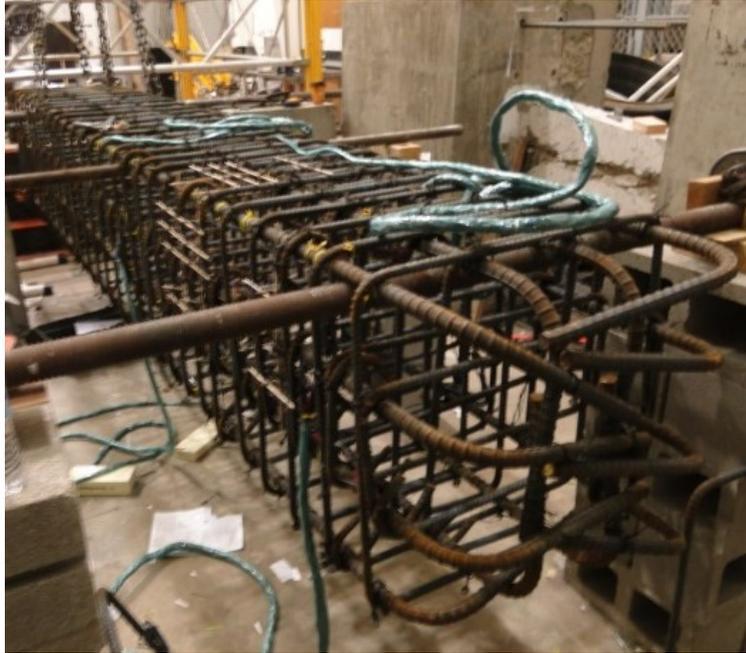
Figure 159. Completed Column Reinforcement Cage
