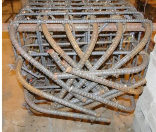
Figure 4. Photo of the bottom of the completed column caging
