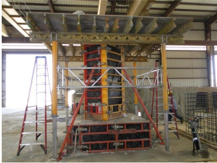
Figure 102. Attaching plywood to supporting beams
