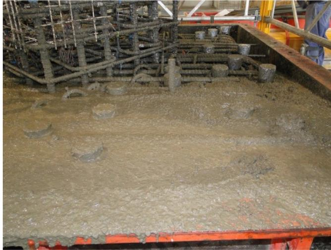
Figure 81. Bottom block casting
