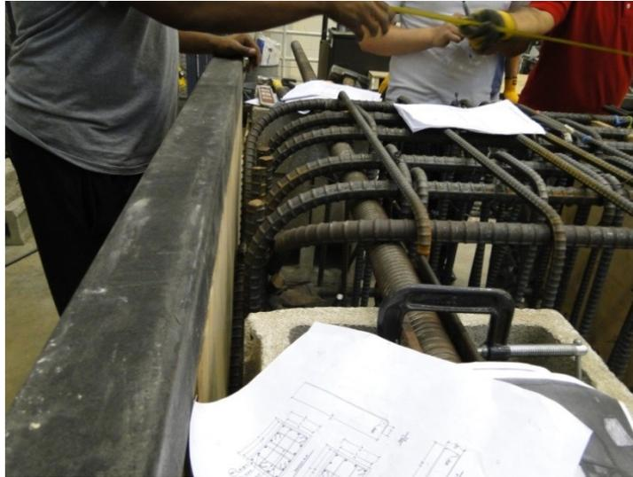
Figure 46. Marking of hoop location relative to the base.
