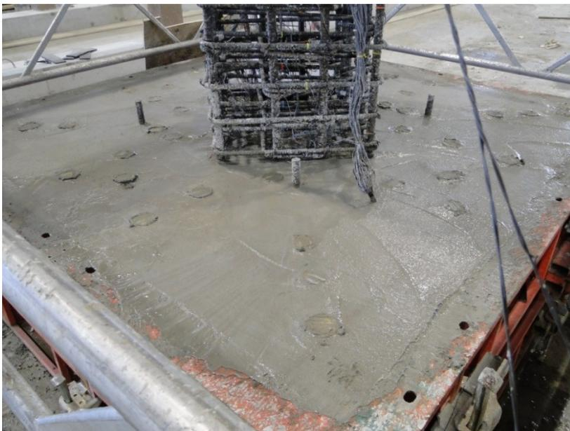
Figure 86. Completed bottom block casting
