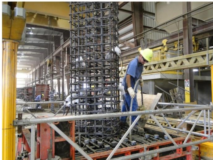
Figure 80. Vibrating the bottom of the footing block
