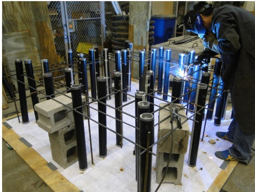
Figure 22. Raising and welding the reinforcement grid.
