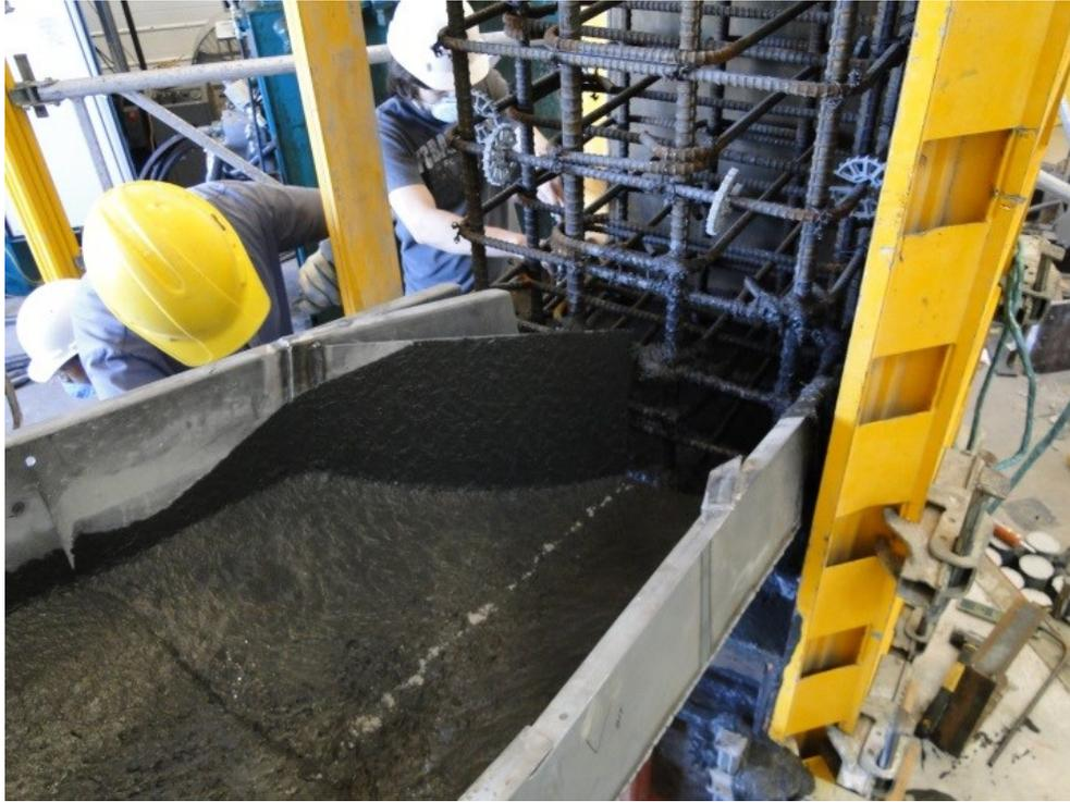
Figure 180. Pouring of UHP-FRC 40" Section
