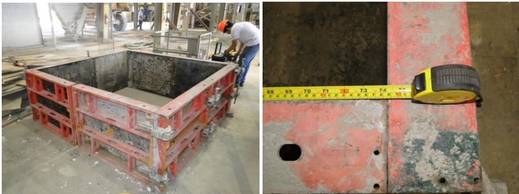
Figure 121. Construction of top block formwork
