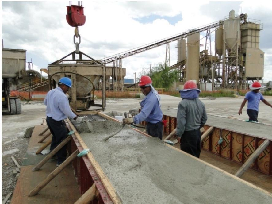
Figure 277. Vibrating during CIP casting
