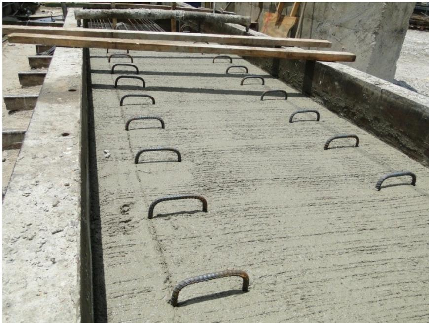
Figure 261. Finished slab beam with horizontal shear reinforcement
