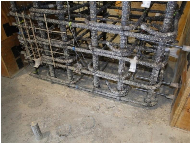
Figure 99. Removal of Laitance Layer
