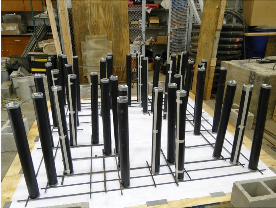
Figure 21. All bars laid out, marked and ready to be welded.
