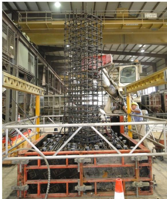
Figure 78. Pouring of concrete into the footing block
