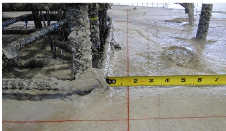
Figure 88. Checking column concrete cover
