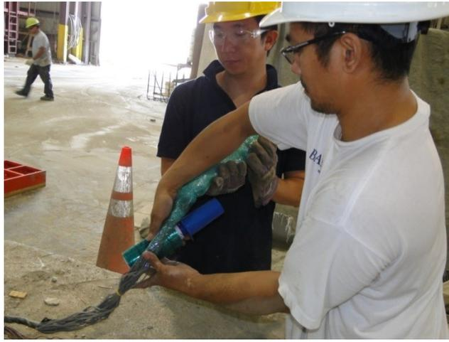
Figure 137. Wrapping footing block wires
