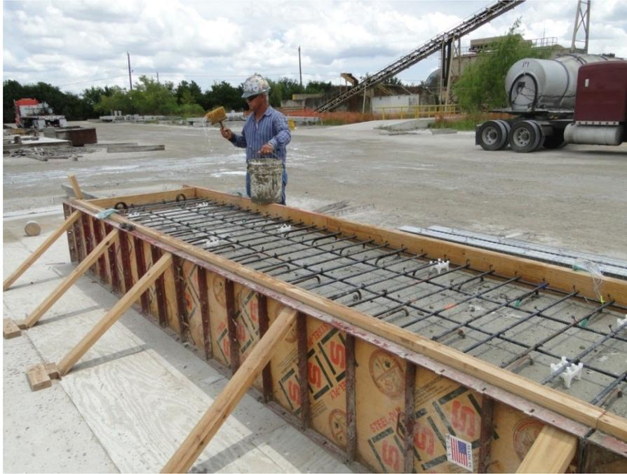
Figure 274. Wetting concrete surface prior to CIP casting
