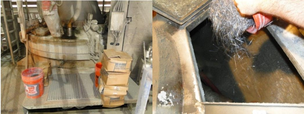
Figure 128. Addition of steel fibers to mixer.
