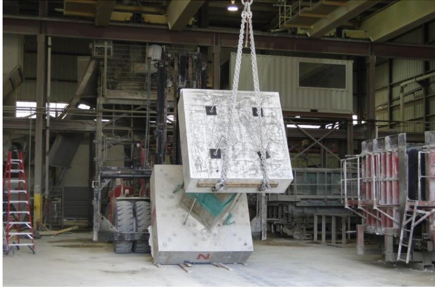
Figure 150. Lowering column to the floor
