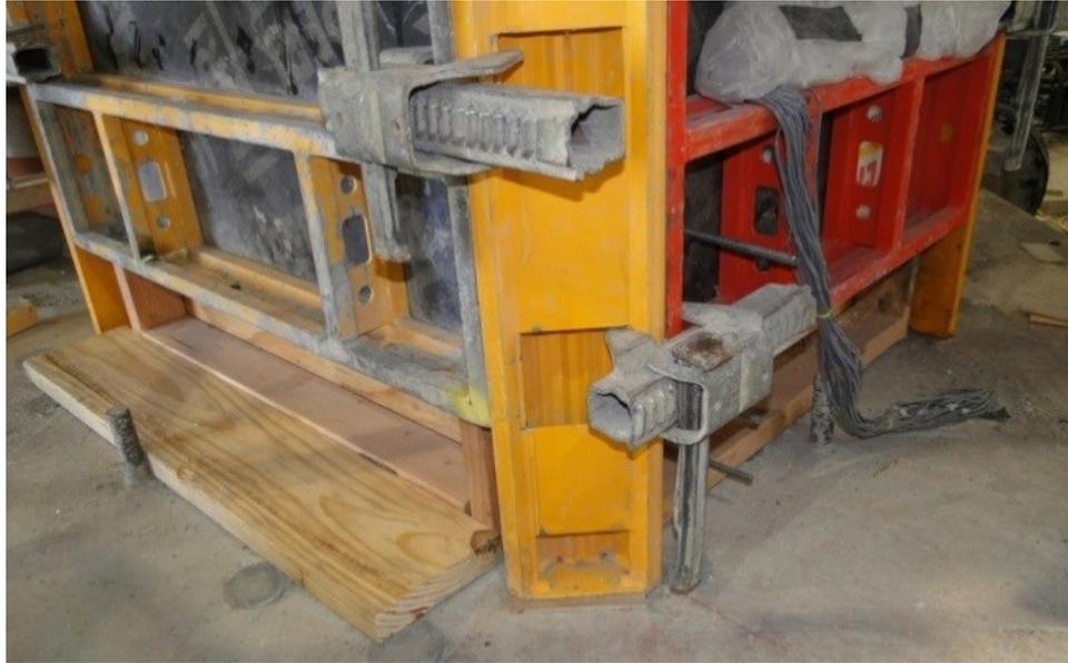
Figure 106. Inserting wooden pieces to secure formwork
