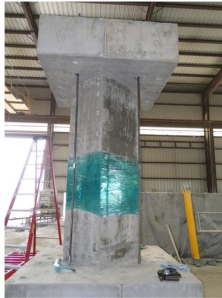
Figure 138. Inserting post tensioning rods
