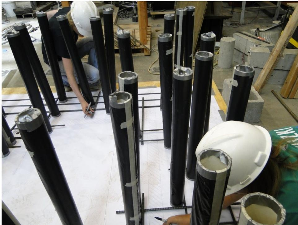
Figure 20. Marking the location of the pipes on the paper and reinforcing bars.
