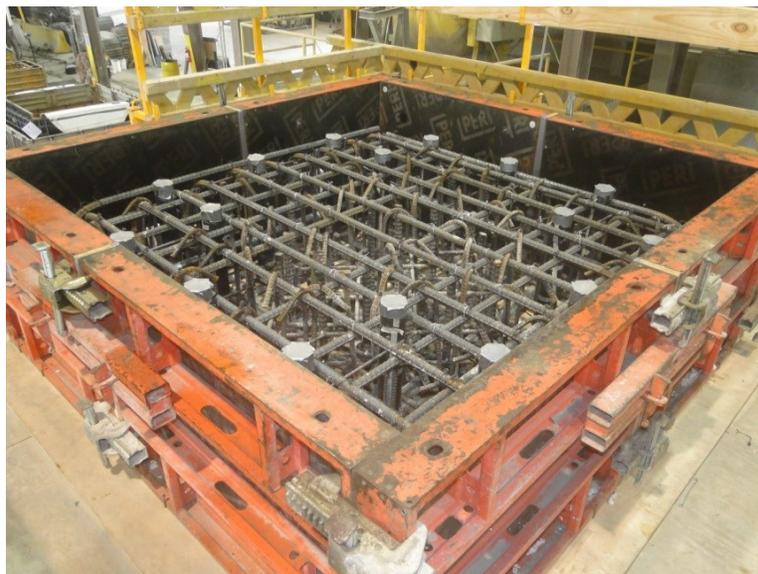
Figure 127. Top block cage and formwork ready for casting
