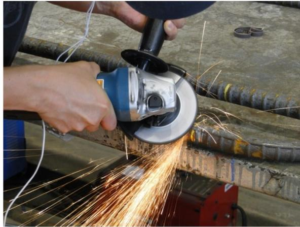
Figure 22. Grinding of deformed rebars with handheld grinder
