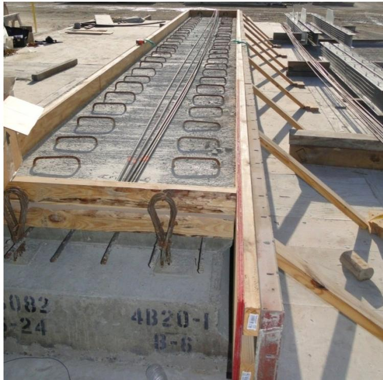
Figure 269. Box beam in CIP formwork
