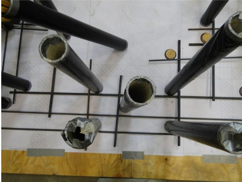
Figure 19. Marking the location of the reinforcement grid on the paper printout.
