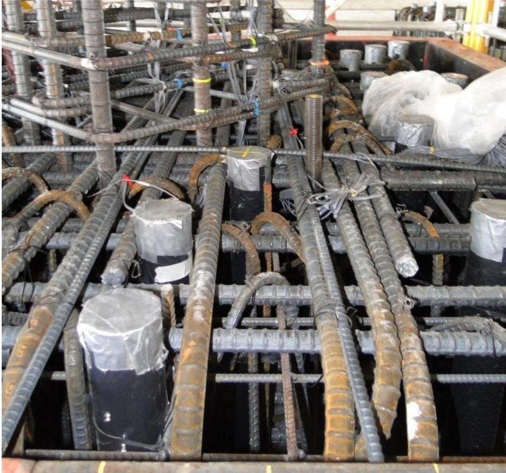
Figure 74. Placement of Footing Strain Gauges
