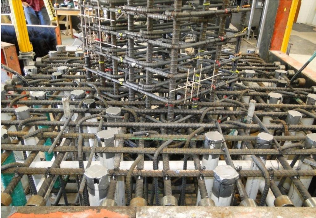
Figure 139. SP3 column and footing cage prior to casting
