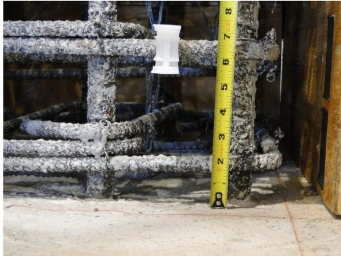
Figure 94. Checking of hoop spacing
