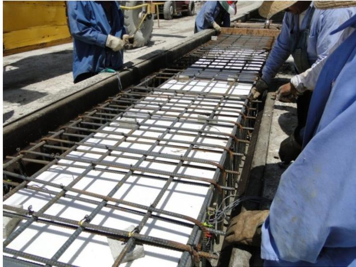
Figure 244. Top reinforcement for box beam without horizontal shear reinforcement
