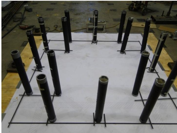
Figure 54. Top block reinforcement grid ready to be welded
