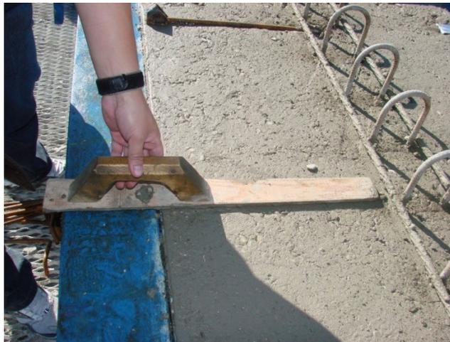
Figure 191. Applying a wood float finish (Texas Prestressed, Elm Mott, Texas; I-girder)
