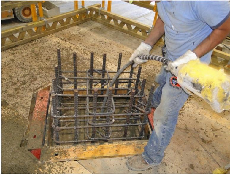
Figure 116. Vibrating column section
