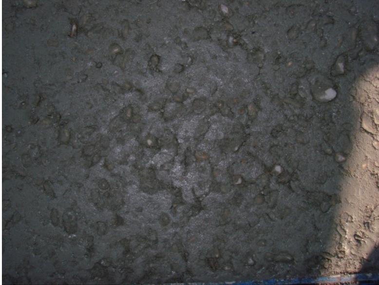
Figure 192. Wet concrete surface after wood float finish
