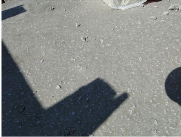
Figure 297. Surface finish on SCC slab beam
