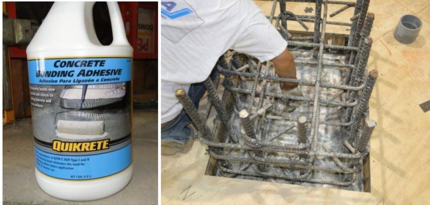
Figure 124. Addition of bonding adhesive
