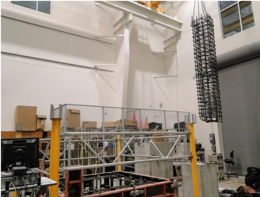
Figure 55. Placing of the column cage into the footing block
