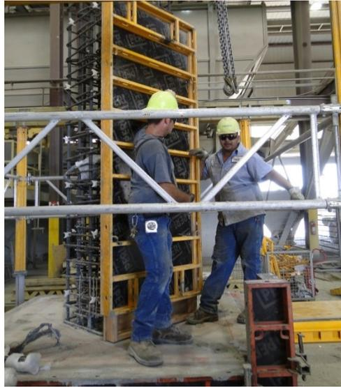
Figure 89. Placing first column formwork panel
