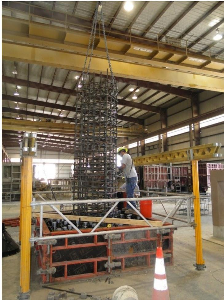
Figure 69. Placement of the column cage
