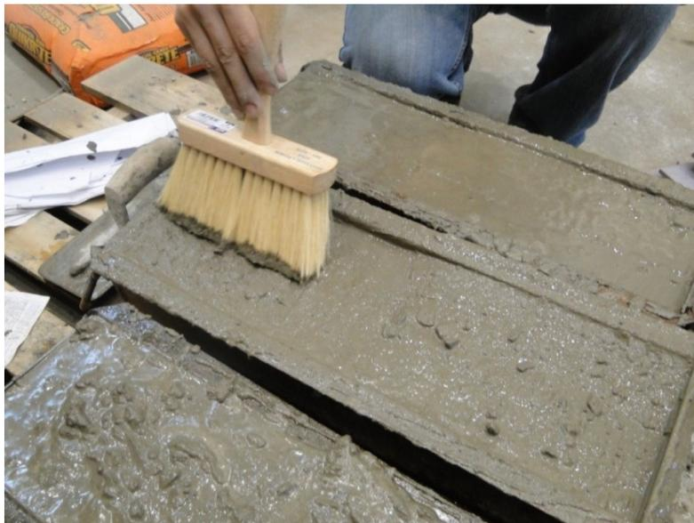
Figure 200. Surface preparation using a concrete broom
