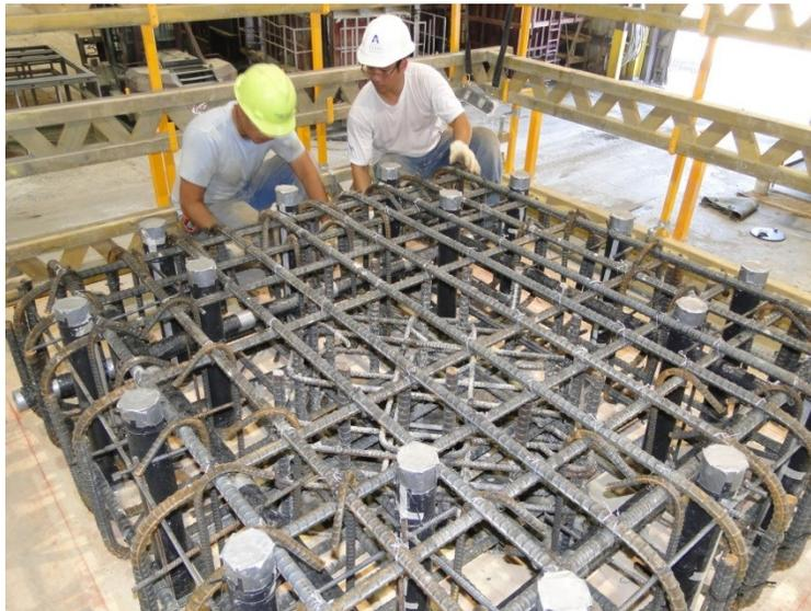
Figure 125. Placing of top block cage
