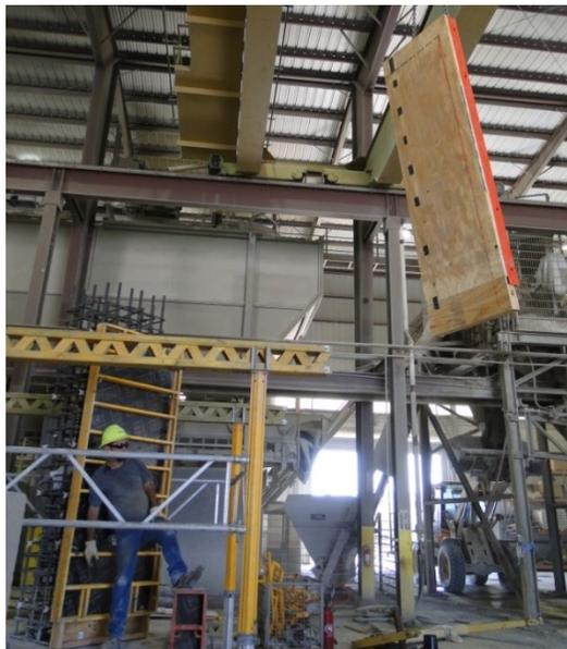
Figure 90. Lifting of formwork panel
