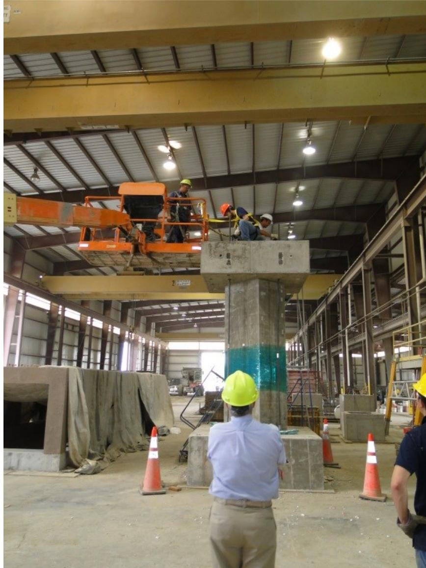
Figure 141. Post tensioning of column
