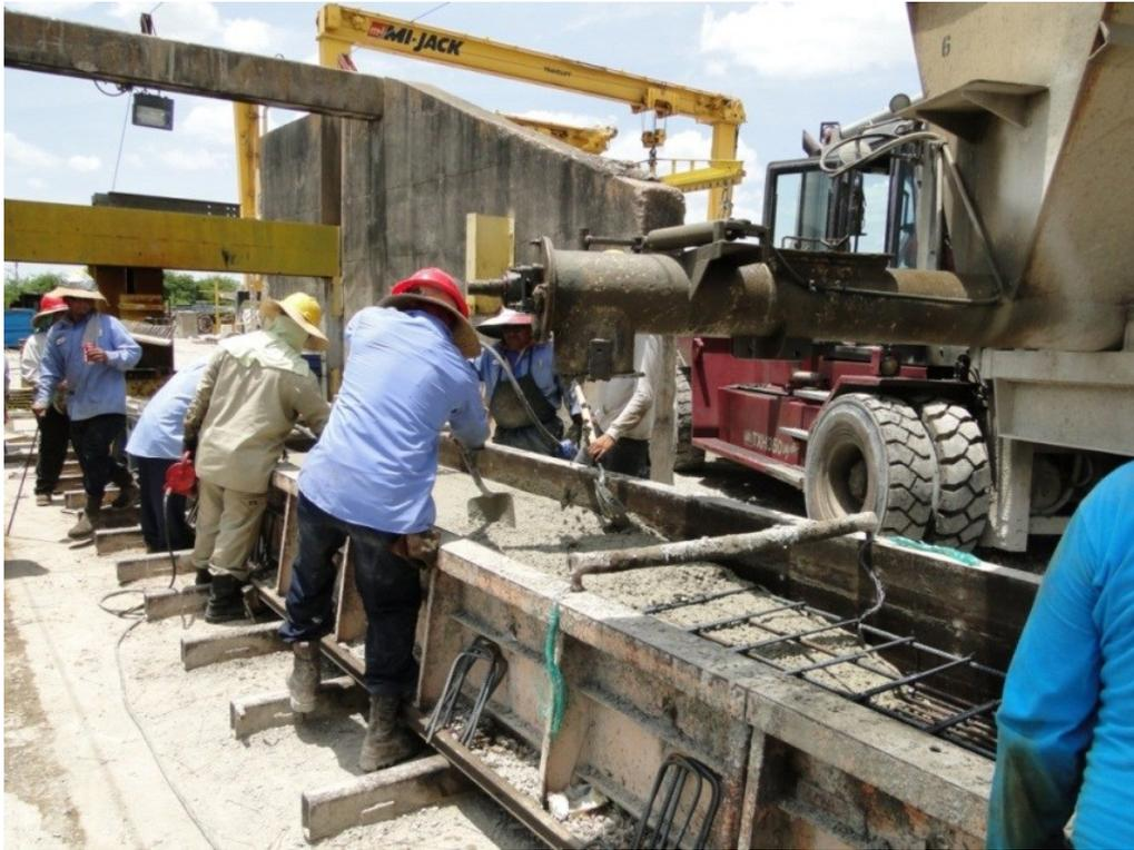
Figure 258. Slab beam casting
