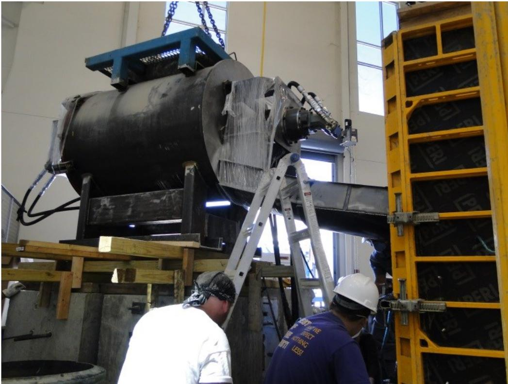
Figure 67. Elevated mixer ready for pouring
