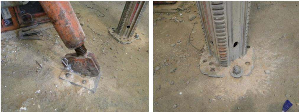
Figure 105. Drilling supports to the floor
