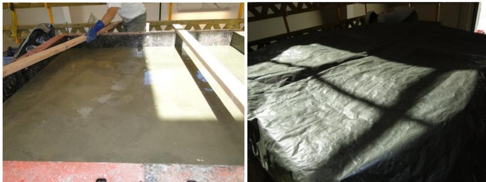
Figure 169. Finishing of top block surface and covering for curing
