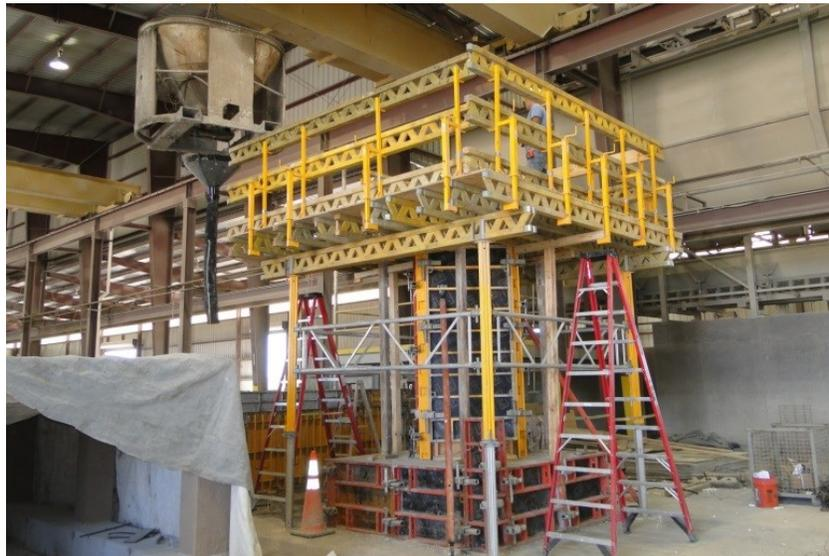
Figure 113. Lifting bucket over column
