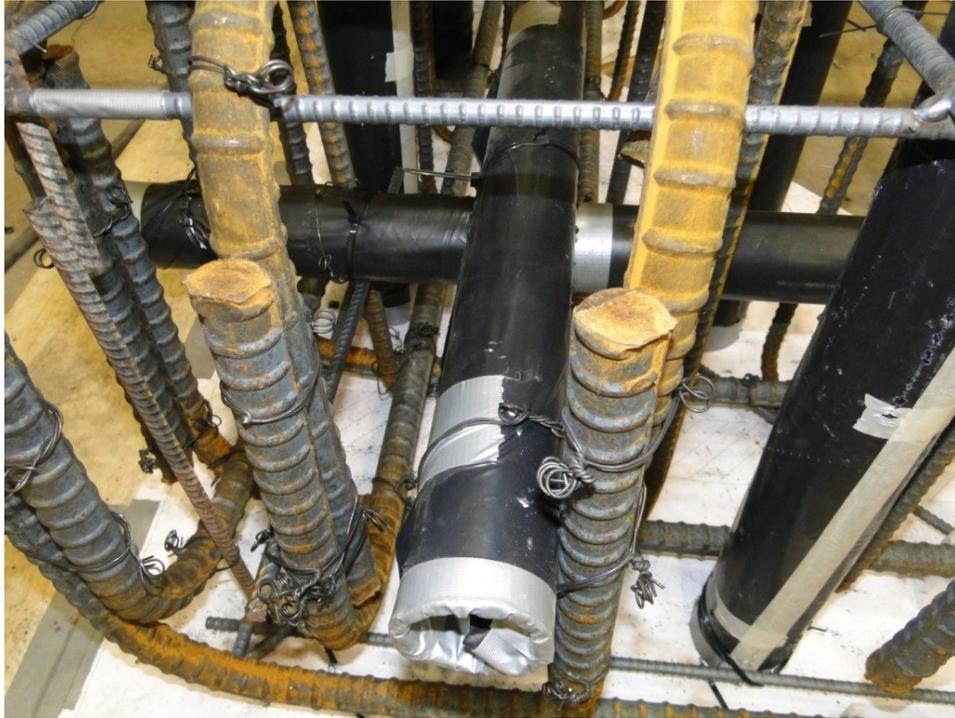
Figure 61. Tying horizontal pvc pipe
