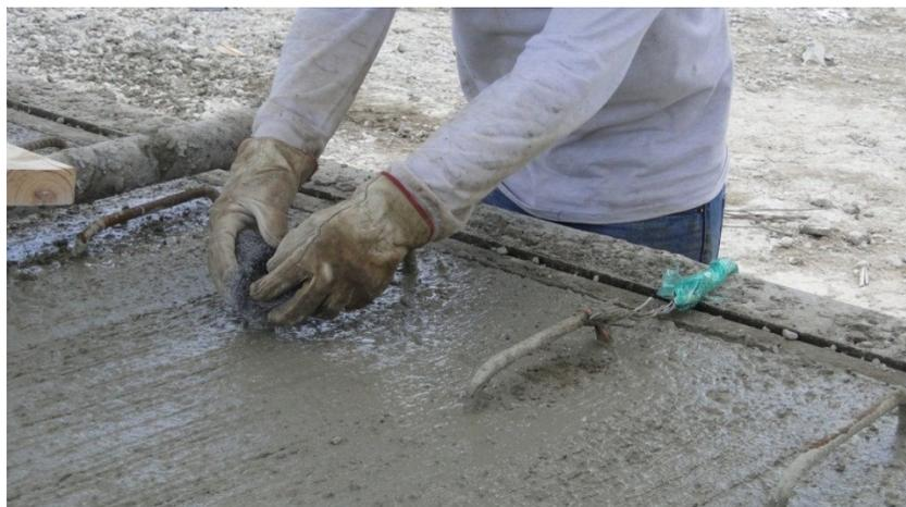
Figure 247. Cleaning of horizontal shear reinforcement
