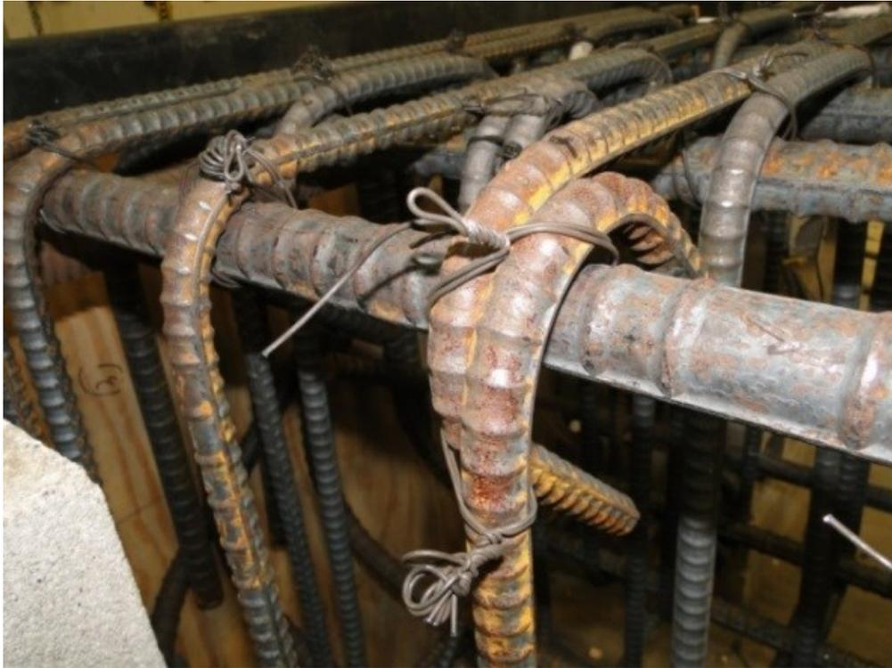
Figure 48. Tying of transverse reinforcement
