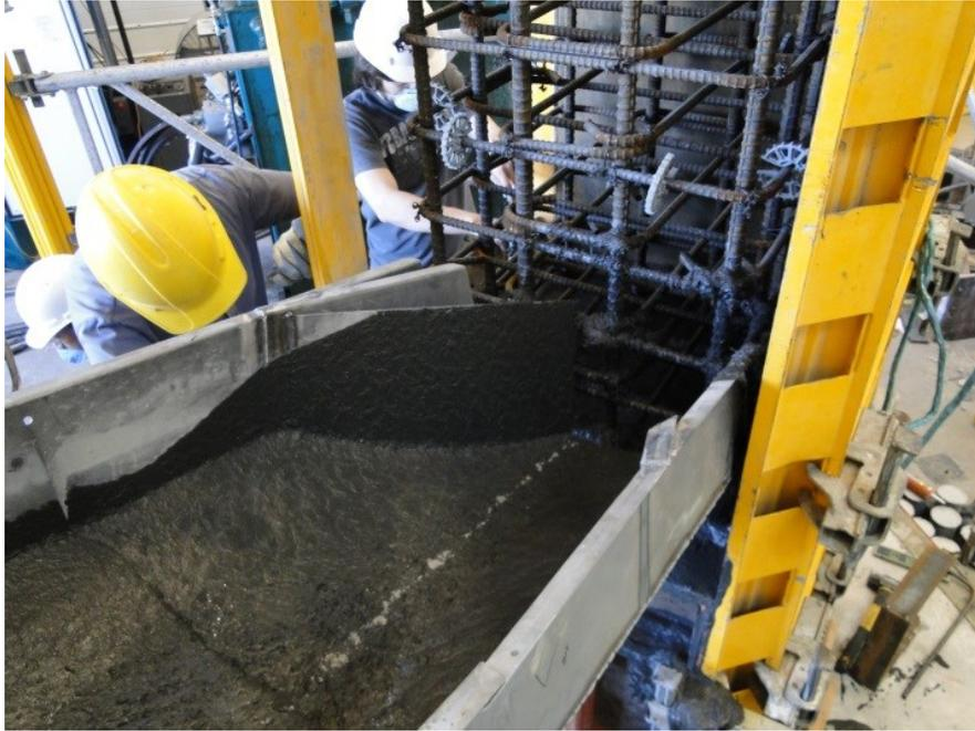
Figure 68. Pouring of UHP-FRC 40 in. section
