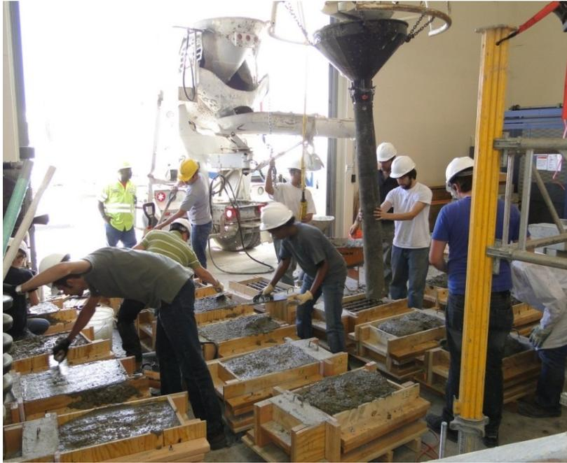
Figure 216. Casting of CIP part of specimens
