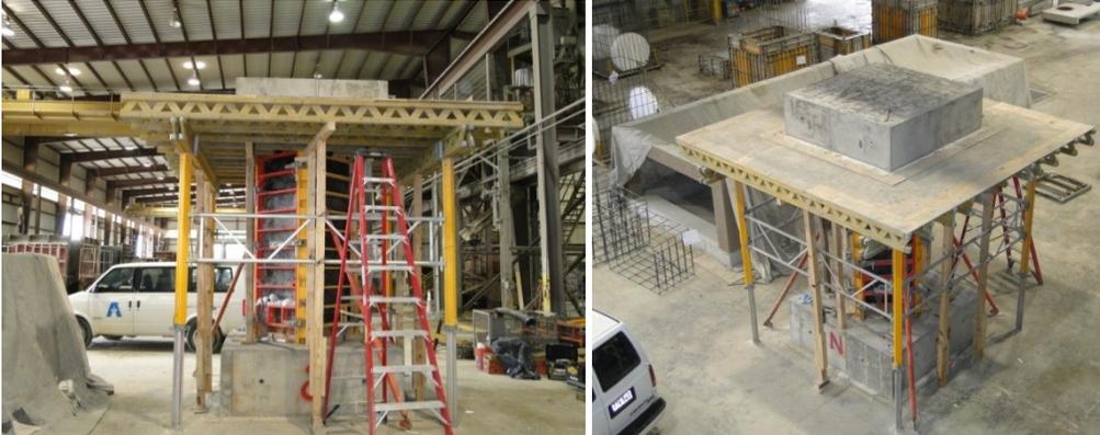
Figure 134. Demolding of top block formwork
