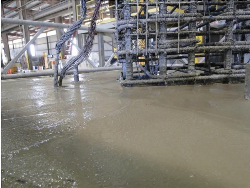
Figure 85. Finished surface of bottom block
