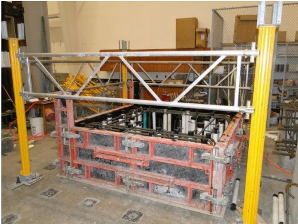
Figure 158. Footing Block Reinforcement and Formwork
