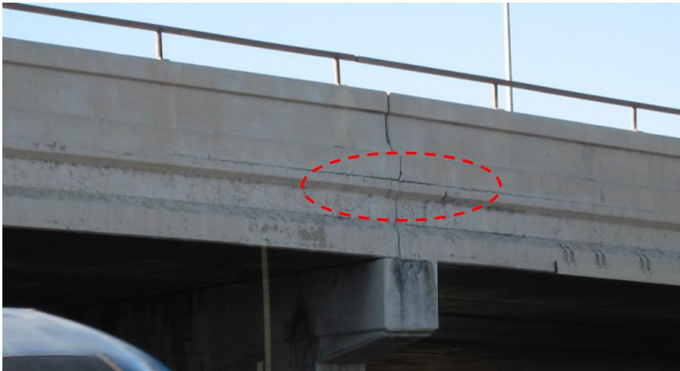
Figure 1. Interface cracks on Riverside Dr. Underpass at I-35
